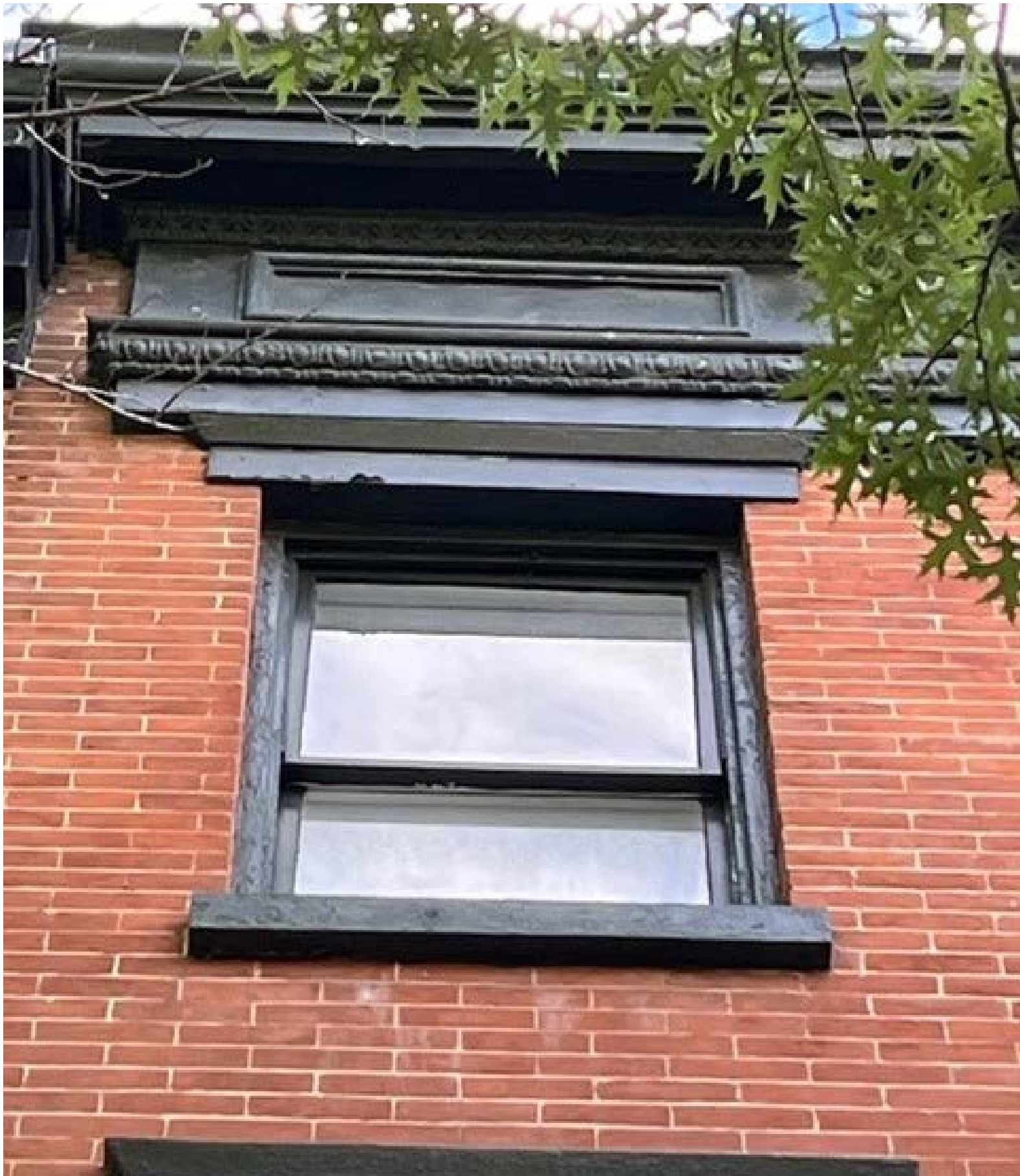
434- Painted lintels + Sill (Top/Bottom), to be stripped + restored to original stone
