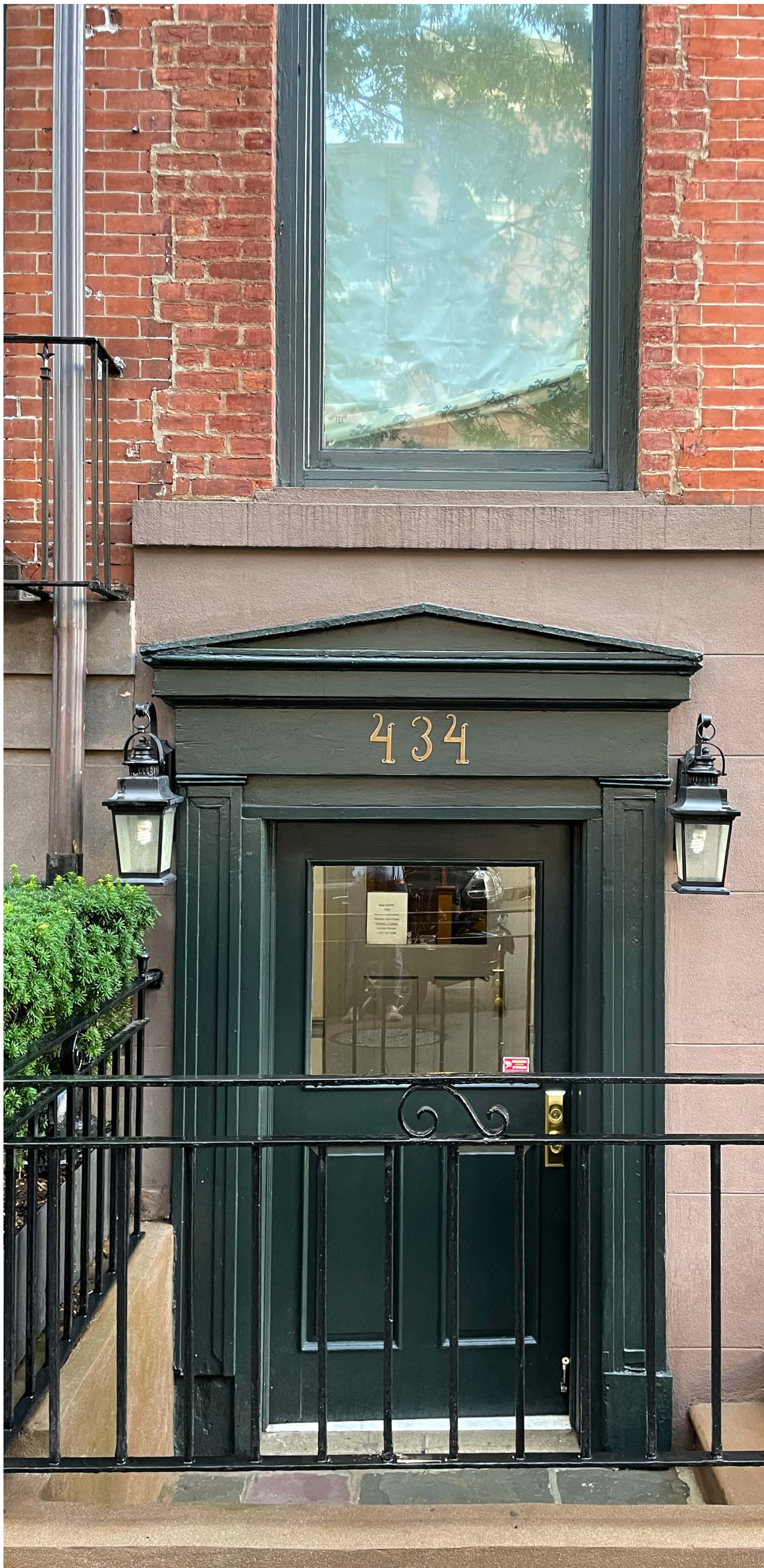
EXISTING 434 BASEMENT ENTRY- TRIM/CASING
