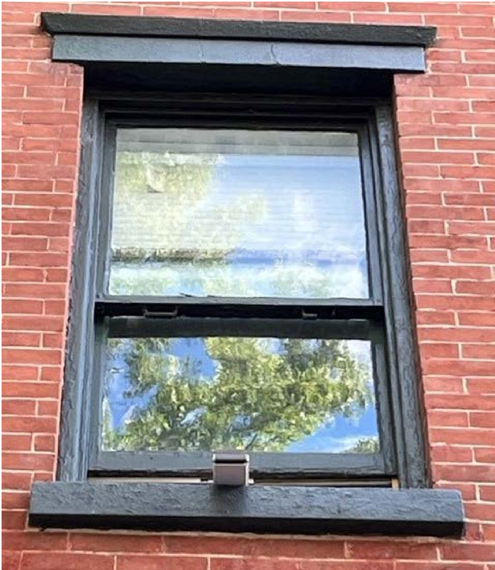
436- Painted lintels + Sill (Top/Bottom), to be stripped + restored to original stone
