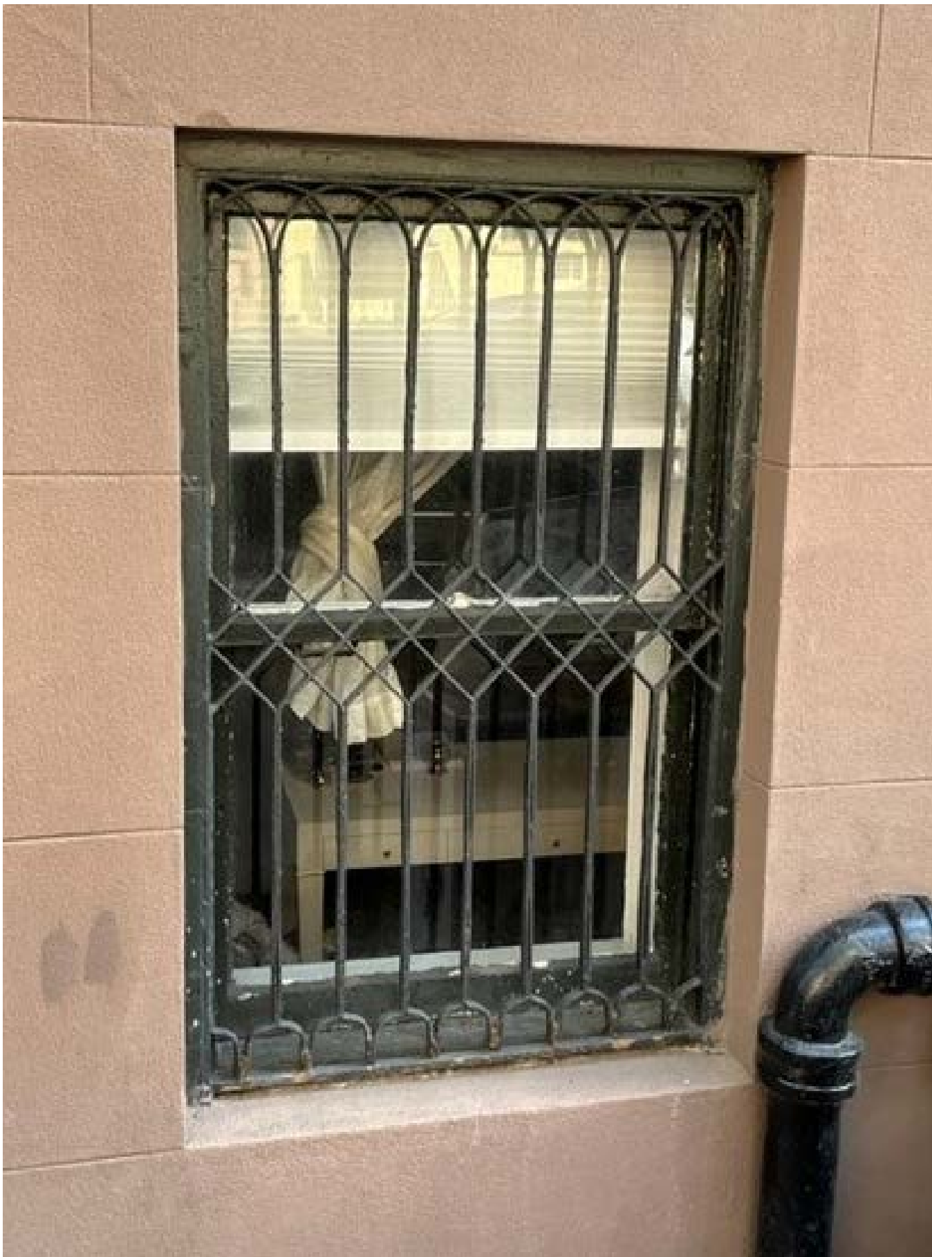
434-436- Basement Window condition, existing grates to be painted Farrow + Ball, Pitch Black, No.256 Satin Finish
