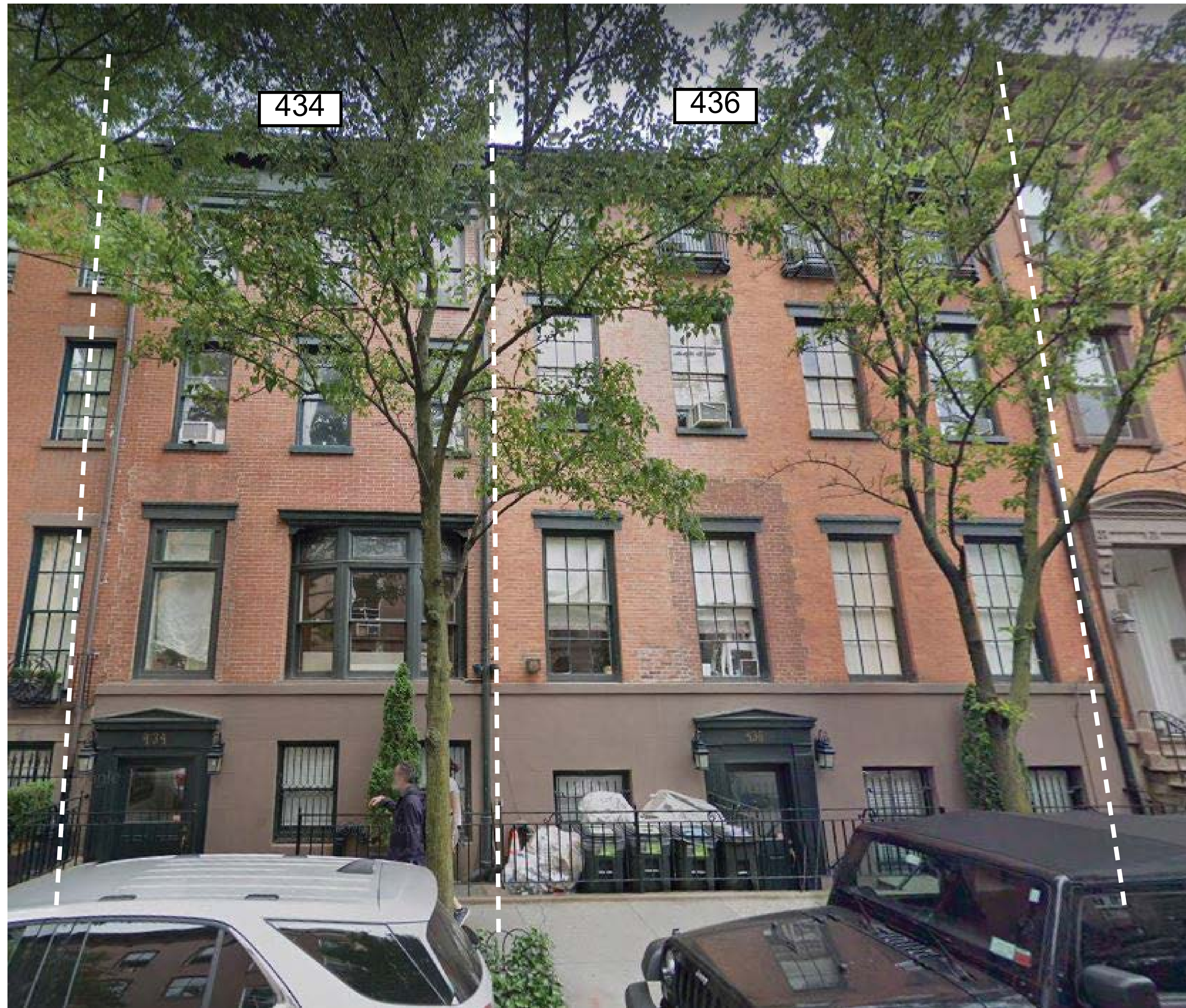
EXISTING 434-436 NORTH FACADE, FACING 22nd STREET
