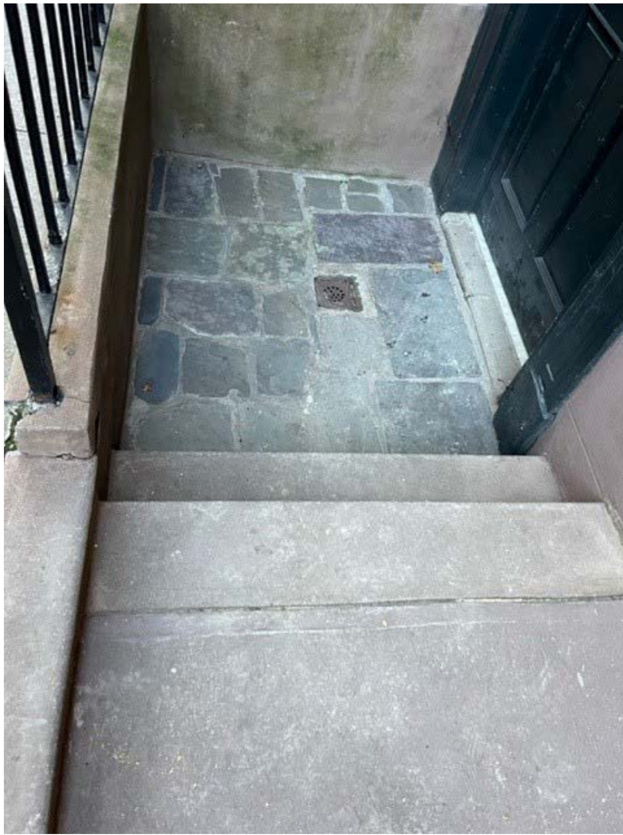
1- EXISTING PAVERS AT 434 ENTRY
