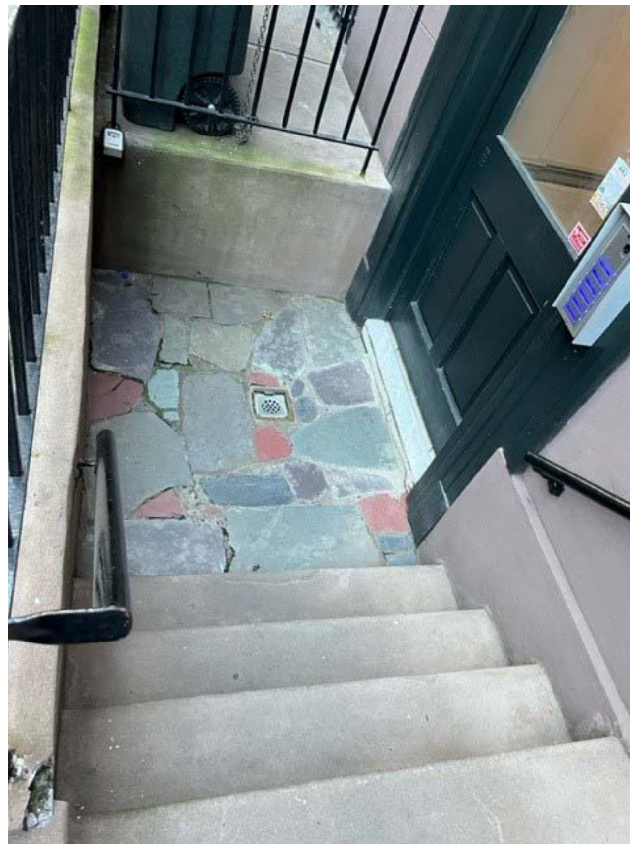
2- EXISTING PAVERS AT 436 ENTRY
