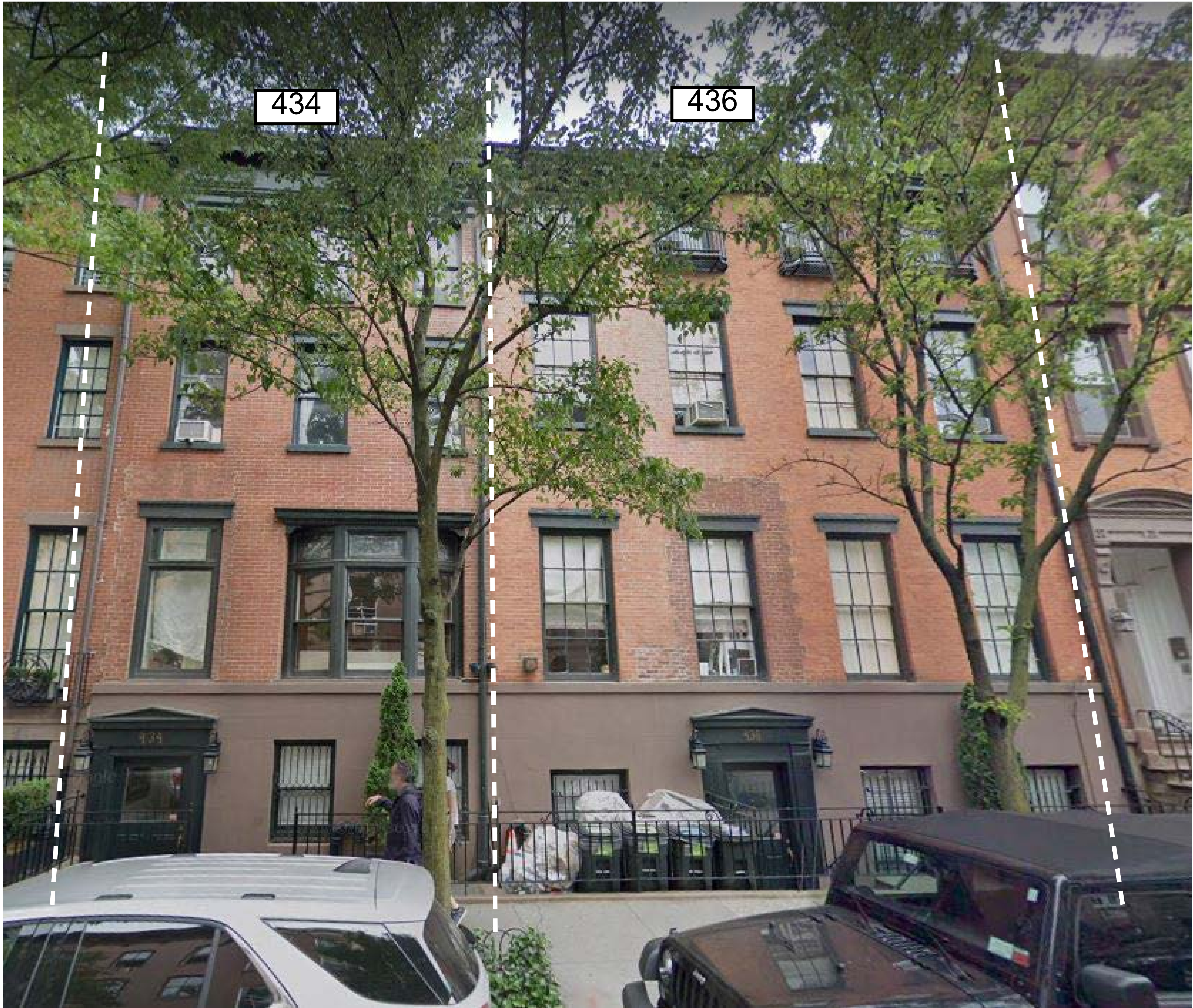
EXISTING 434-436 NORTH FACADE, FACING 22nd STREET
