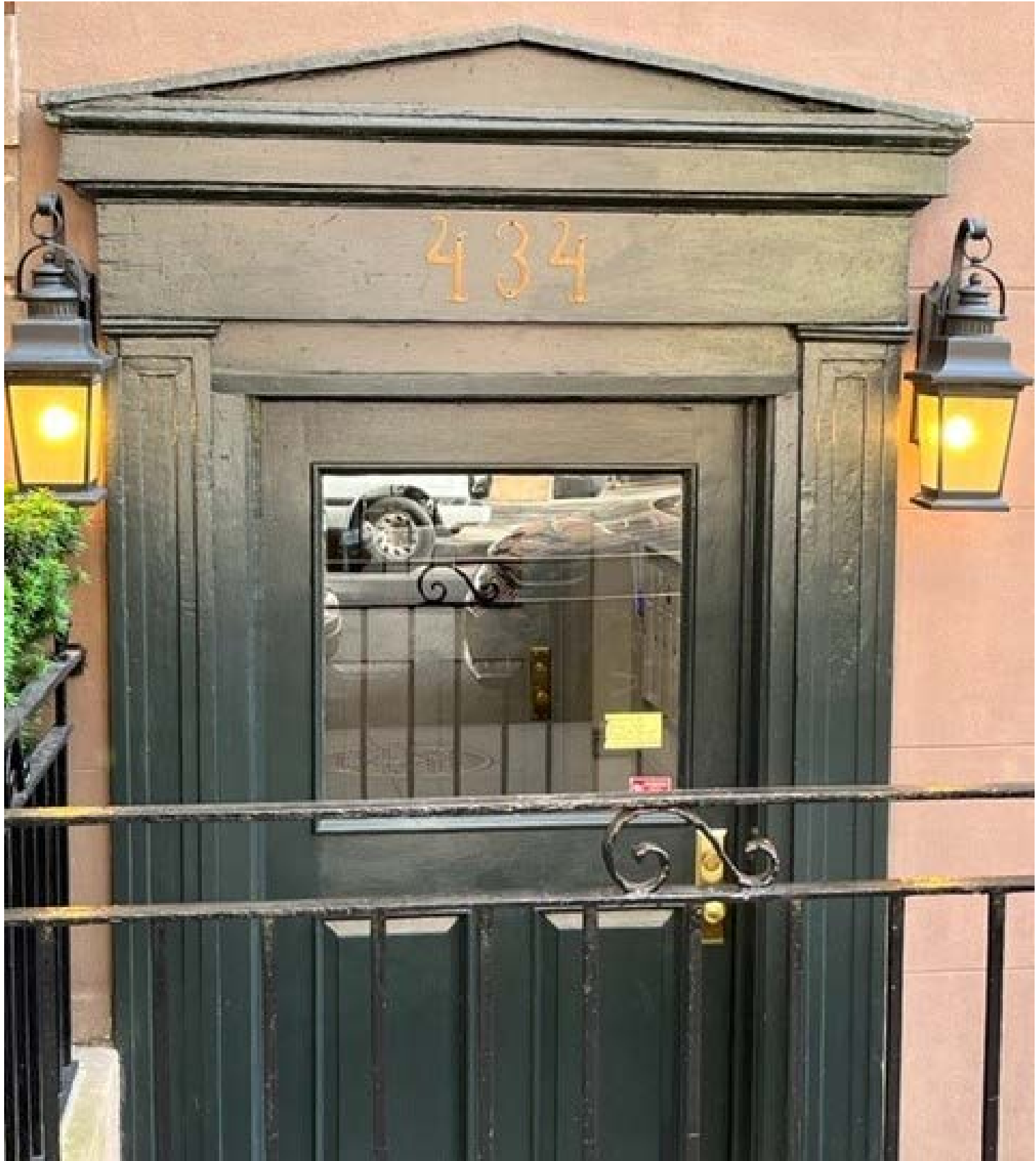
434- Existing Basement Entry Condition
