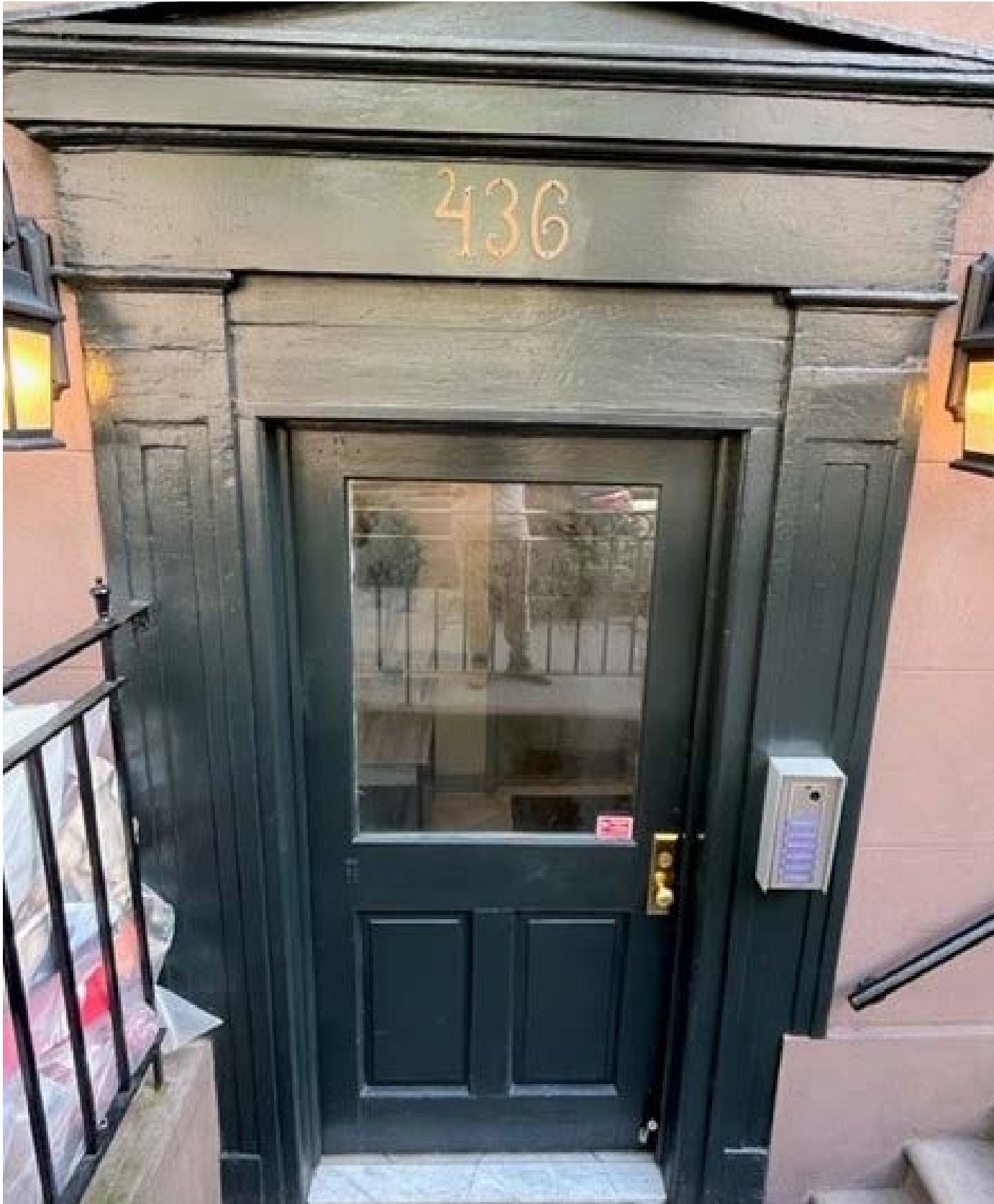
436- Existing Basement Entry Condition
