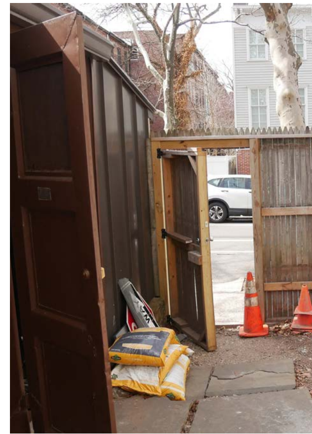
NORTH WALL OF GARAGE
