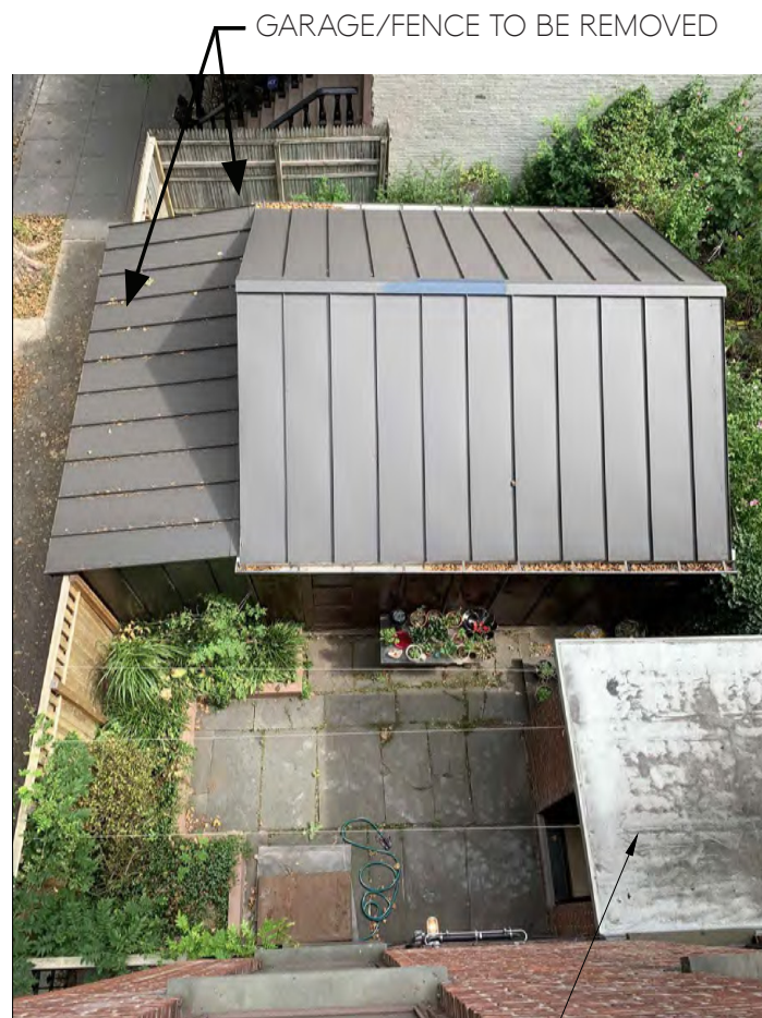
VIEW OF EXISTING REAR YARD, GARAGE, AND FENCE
