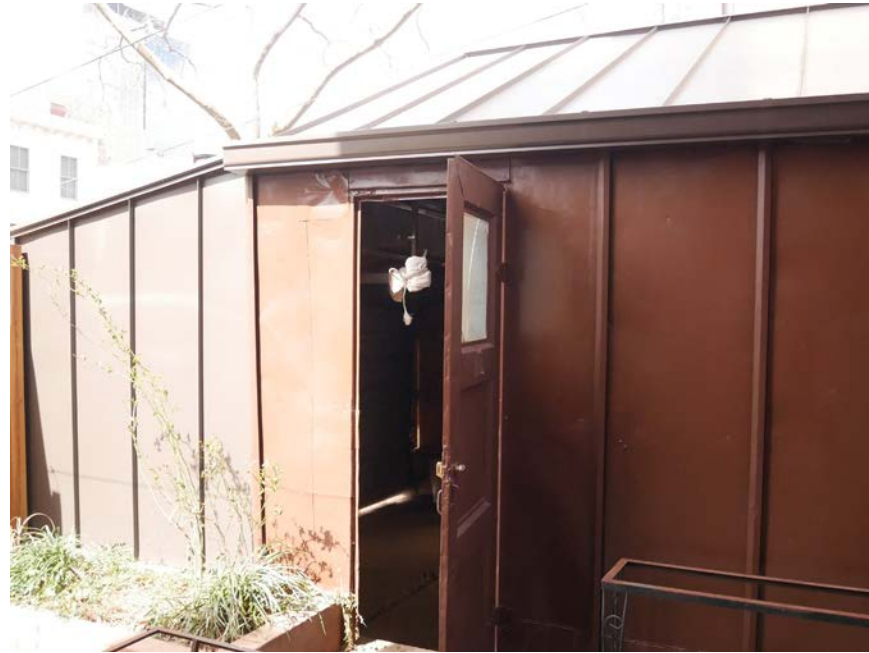
SOUTH WALL OF GARAGE
