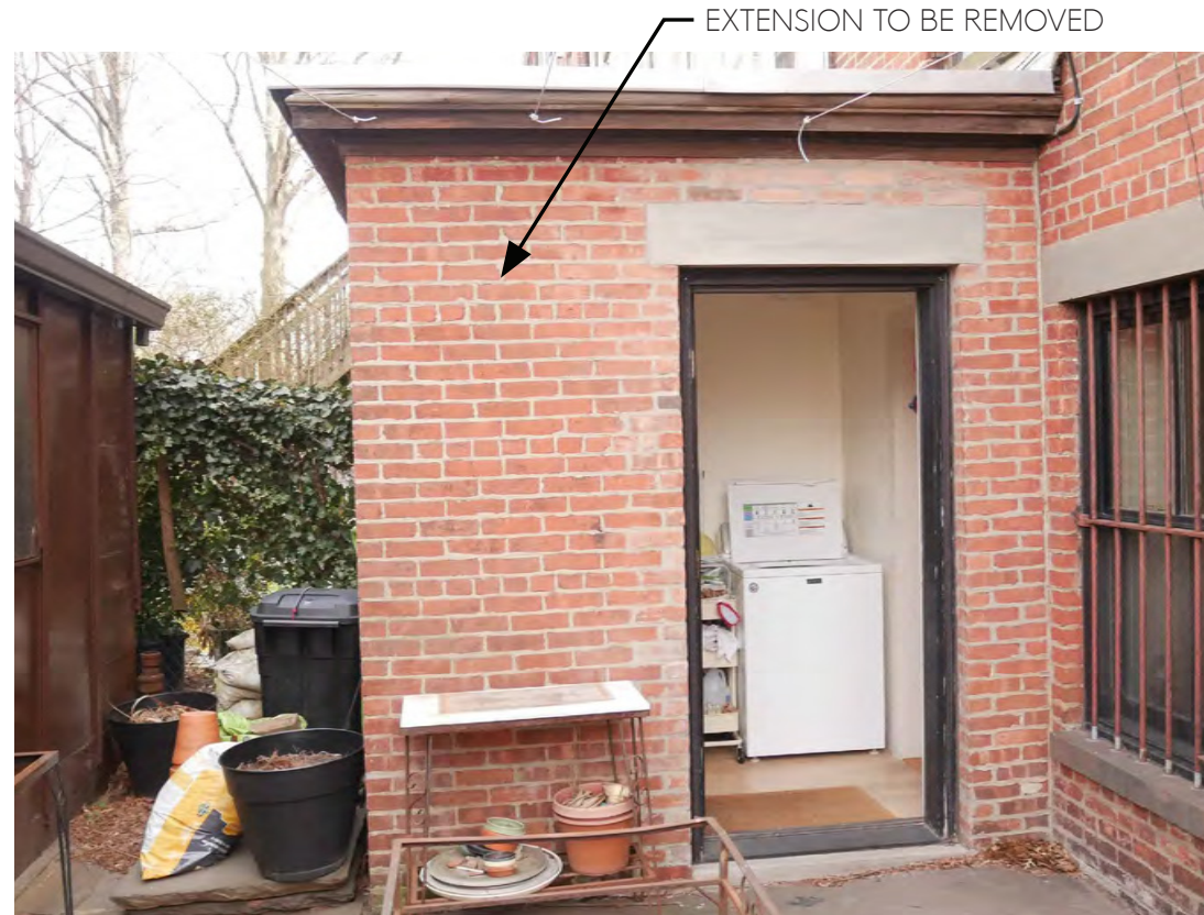
VIEW OF EXISTING REAR YARD EXTENSION
