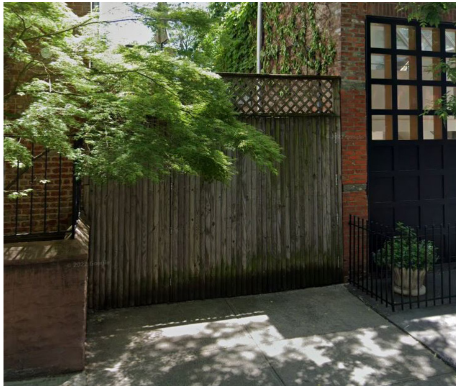
EXISTING WOOD FENCE 192 DEAN STREET, BROOKLYN
