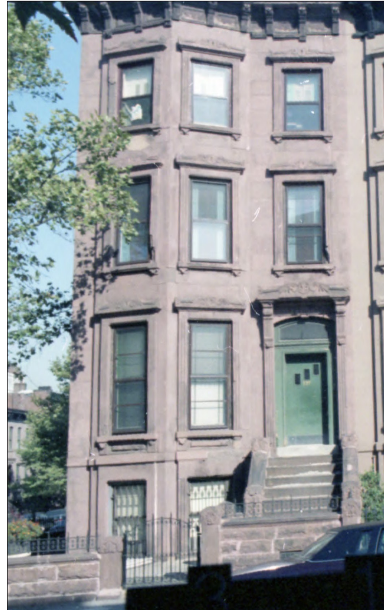
HISTORIC CONDITION: 137 ST MARKS AVE
