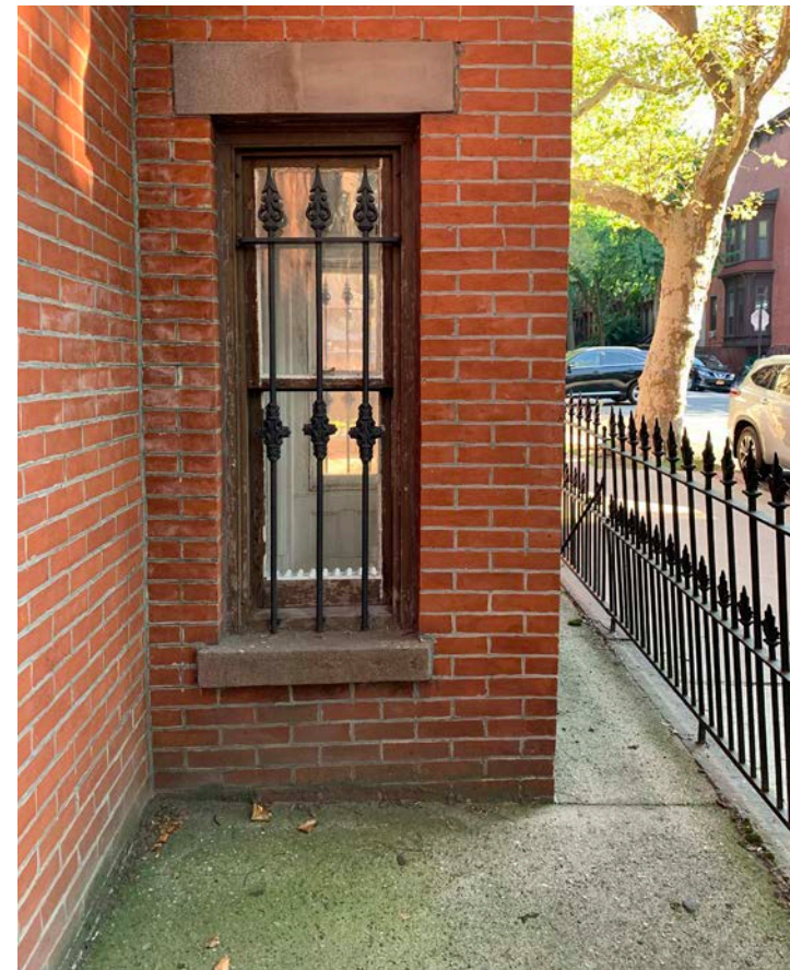
VIEW OF SIDE YARD FACING SOUTH AT BAY WINDOW
