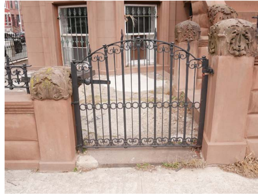
VIEW OF FRONT YARD/AREAWAY FACING NORTH
