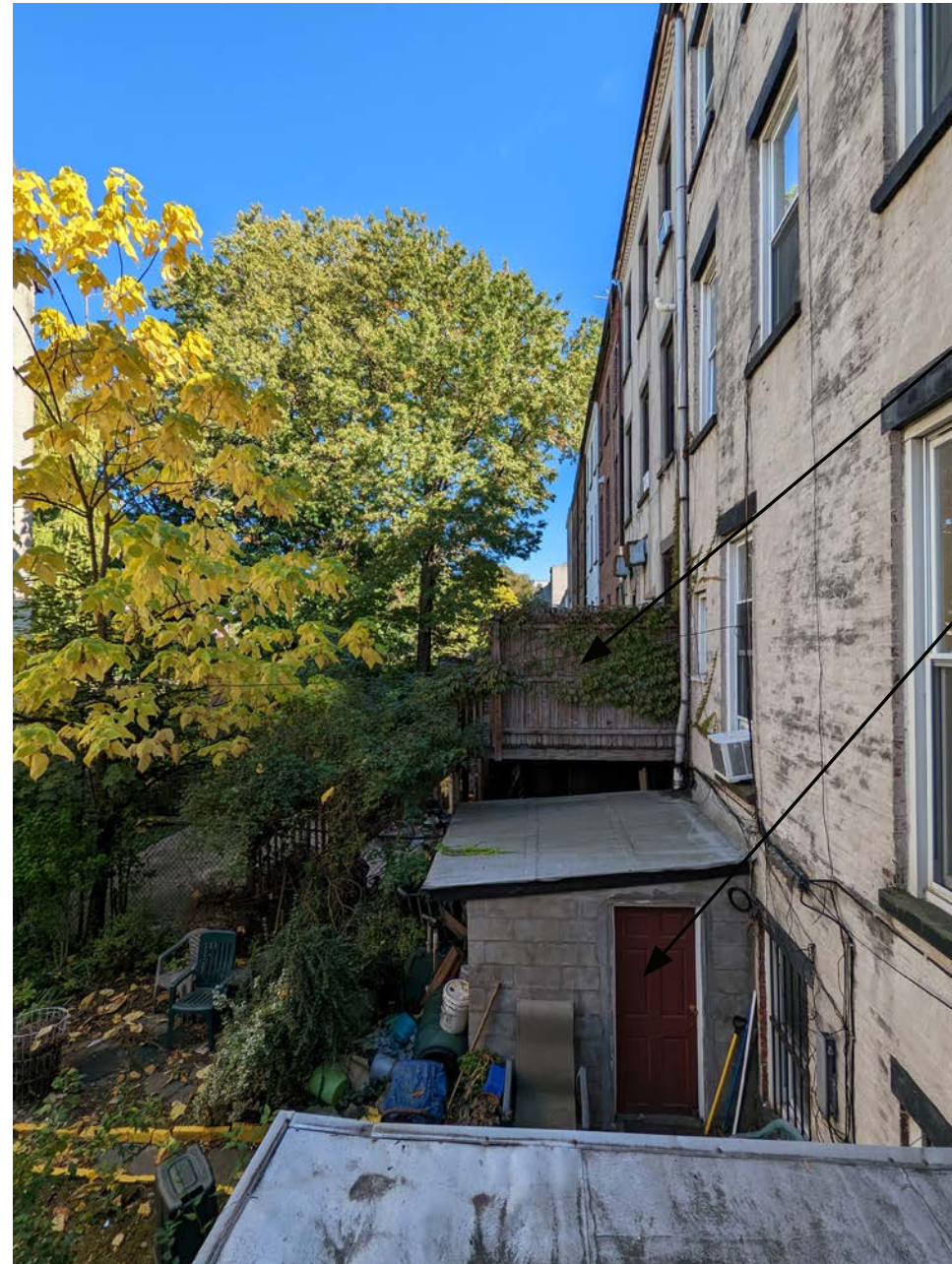
VIEW OF EXISTING NEIGHBORING FACADE FROM 137 ST MARKS FACING EAST
