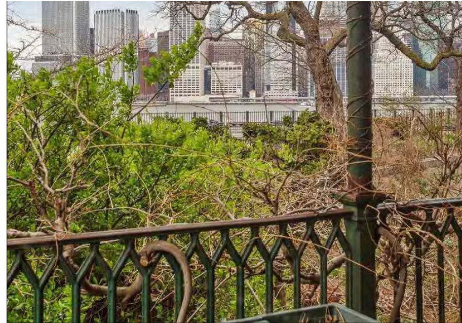
BALCONY BALUSTRADE, MONTAGUE TERR, BROOKLYN HEIGHTS
