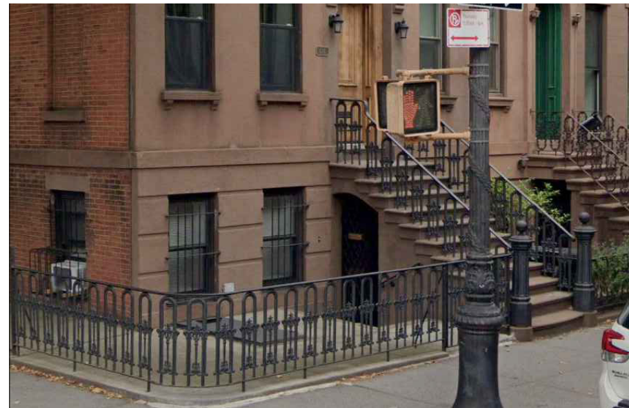
FENCE AND STAIR BALUSTRADE, CLINTON ST, CARROLL GARDENS
