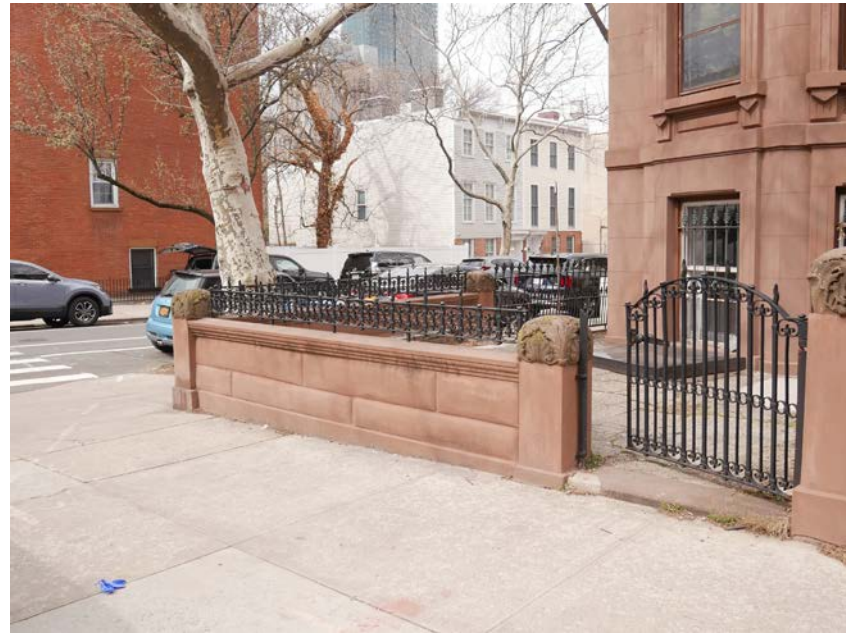
VIEW OF FRONT YARD FACING NORTHWEST
