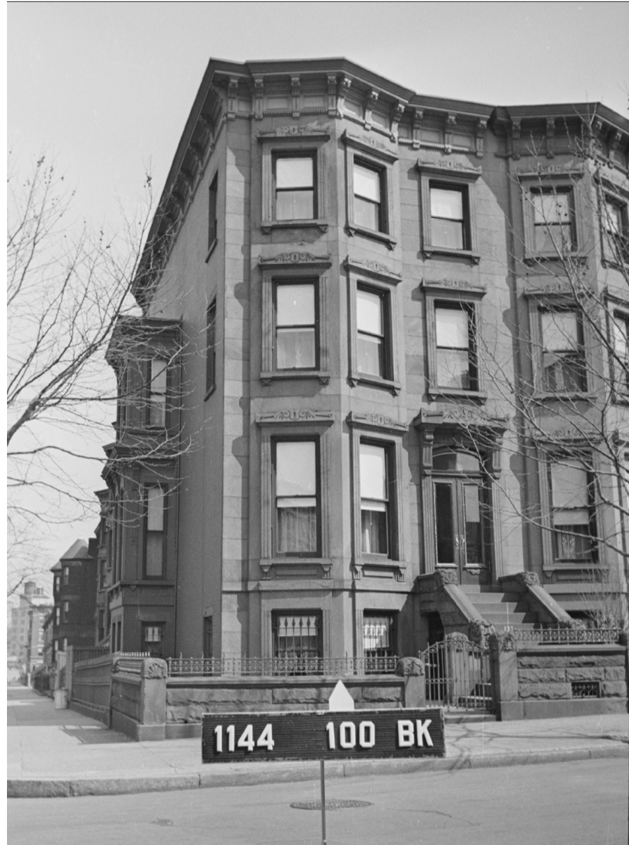
HISTORIC CONDITION: 137 ST MARKS AVE
