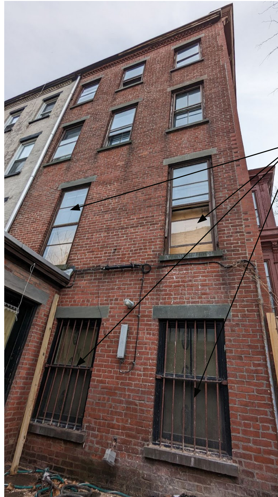
VIEW OF EXISTING REAR FACADE
