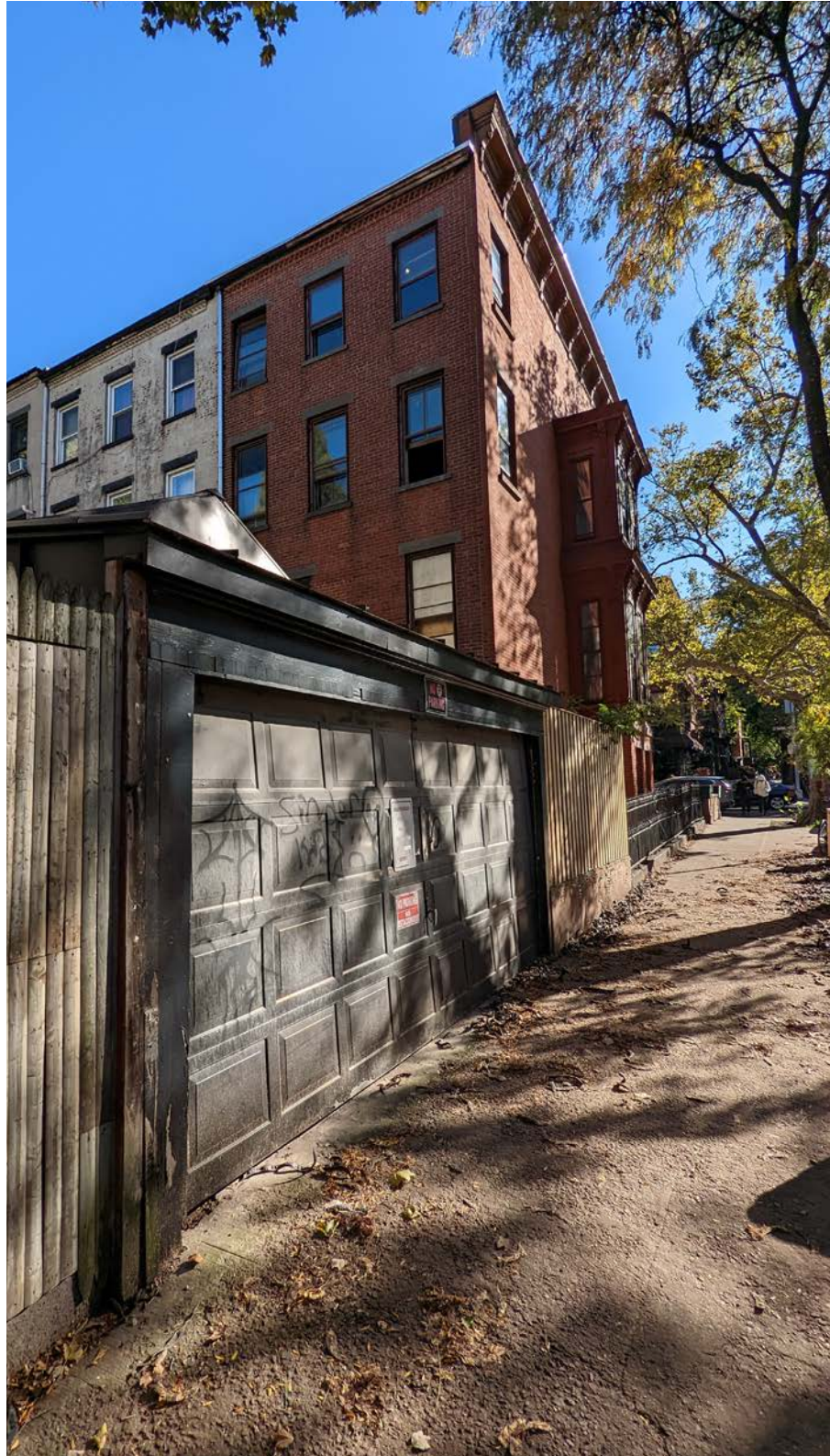
VIEW FROM CARLTON AVE: FACING SOUTHEAST
