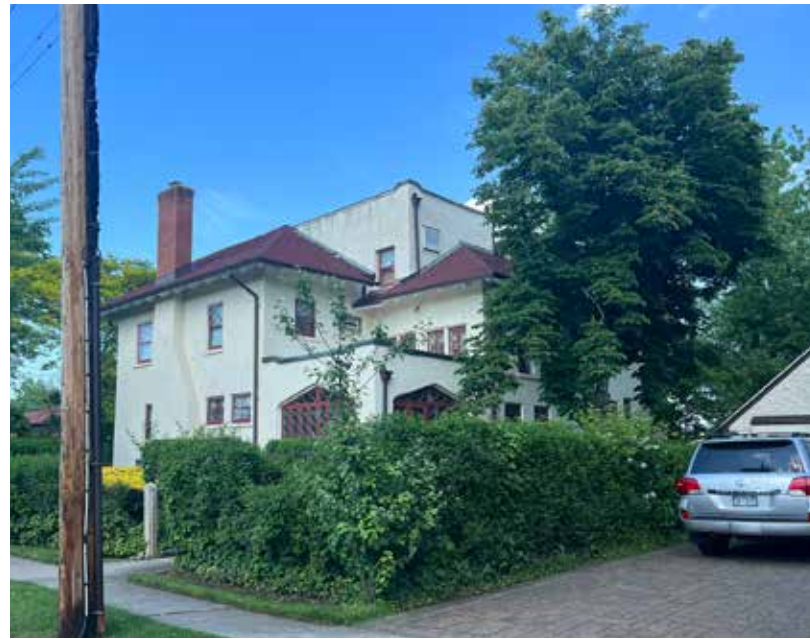
EXISTING REFERENCE: 104 KNOLLWOOD, DOUGLASTON, NY
