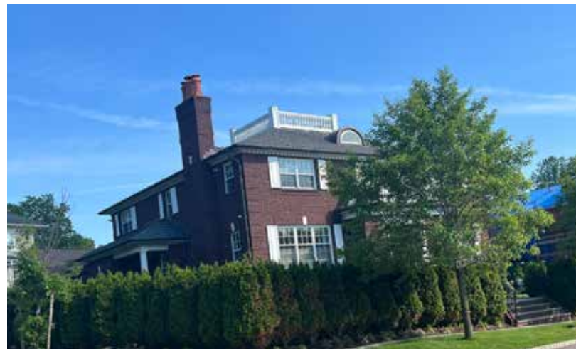
EXISTING REFERENCE: 27-03 SHORE RD, DOUGLASTON, NY
