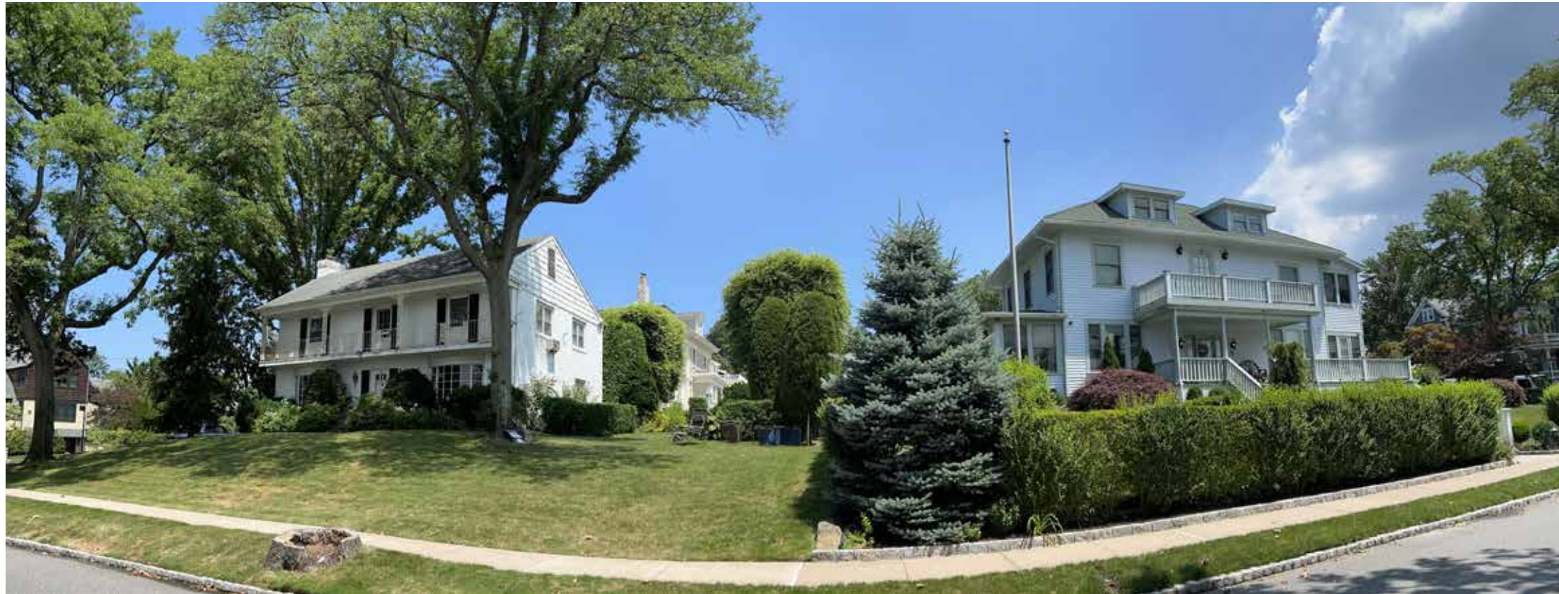
EXISTING WEST VIEW_SHORE ROAD
