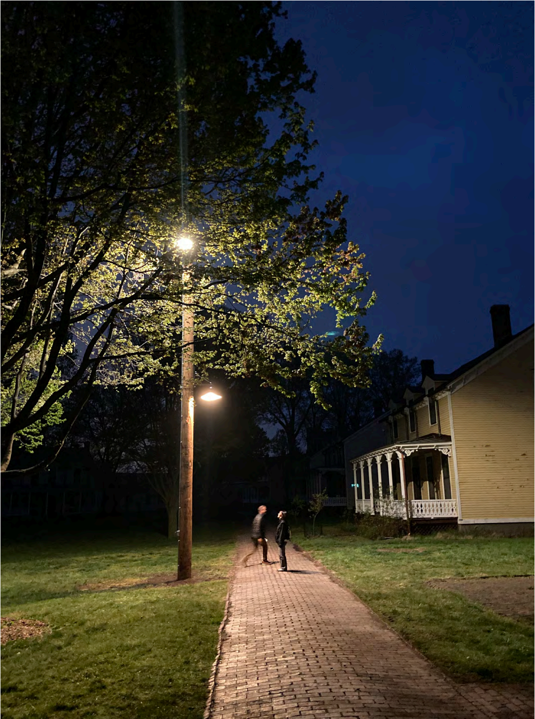
Left: Photograph of lighting mock-up in Nolan Park with Building 9 at background. Right: Photograph of same mock-up showing the combination moonlight and streetlight on one post.
