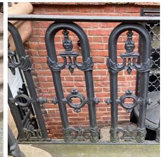
restore original railing, paint black
