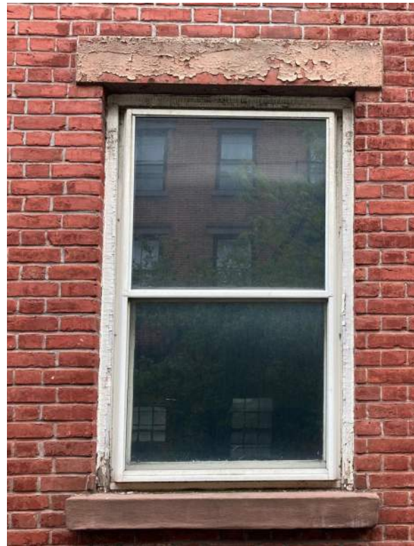
existing window lintel proposed lintel material: cast stone tinted to match brownstone
