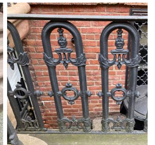
restore original railing, paint black
