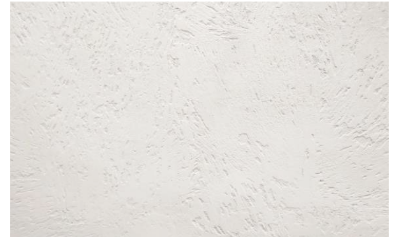
penthouse facade stucco
