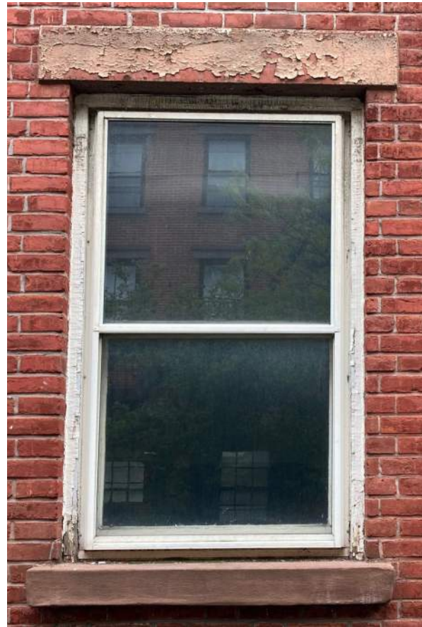
front windows replace existing to match (white finish) Restore existing window sills and headers
