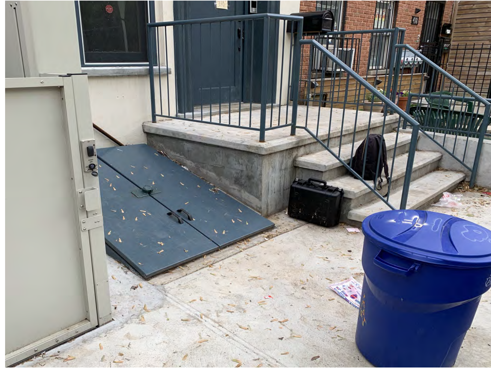
FRONT STOOP & BASEMENT ACCESS HATCH
