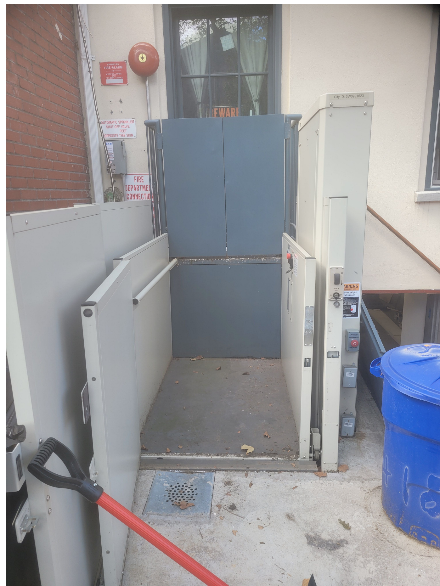
2 PHOTO OF EXISTING LIFT WITH DOORS OPEN Scale:
