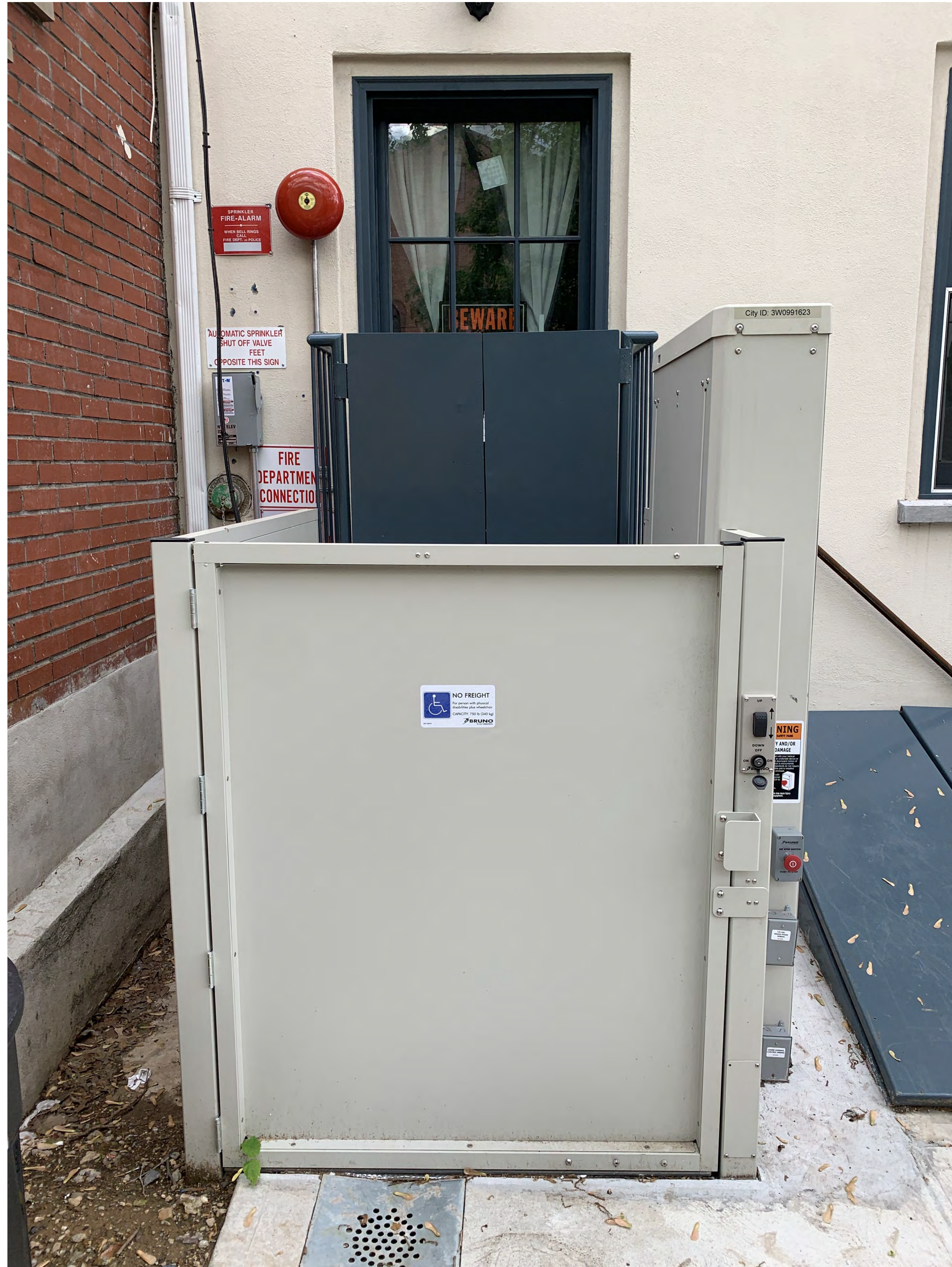
EXISTING FRONT YARD - DIRT AREAWAY BETWEEN LIFT AND FIRE SAFETY EQUIPMENT
