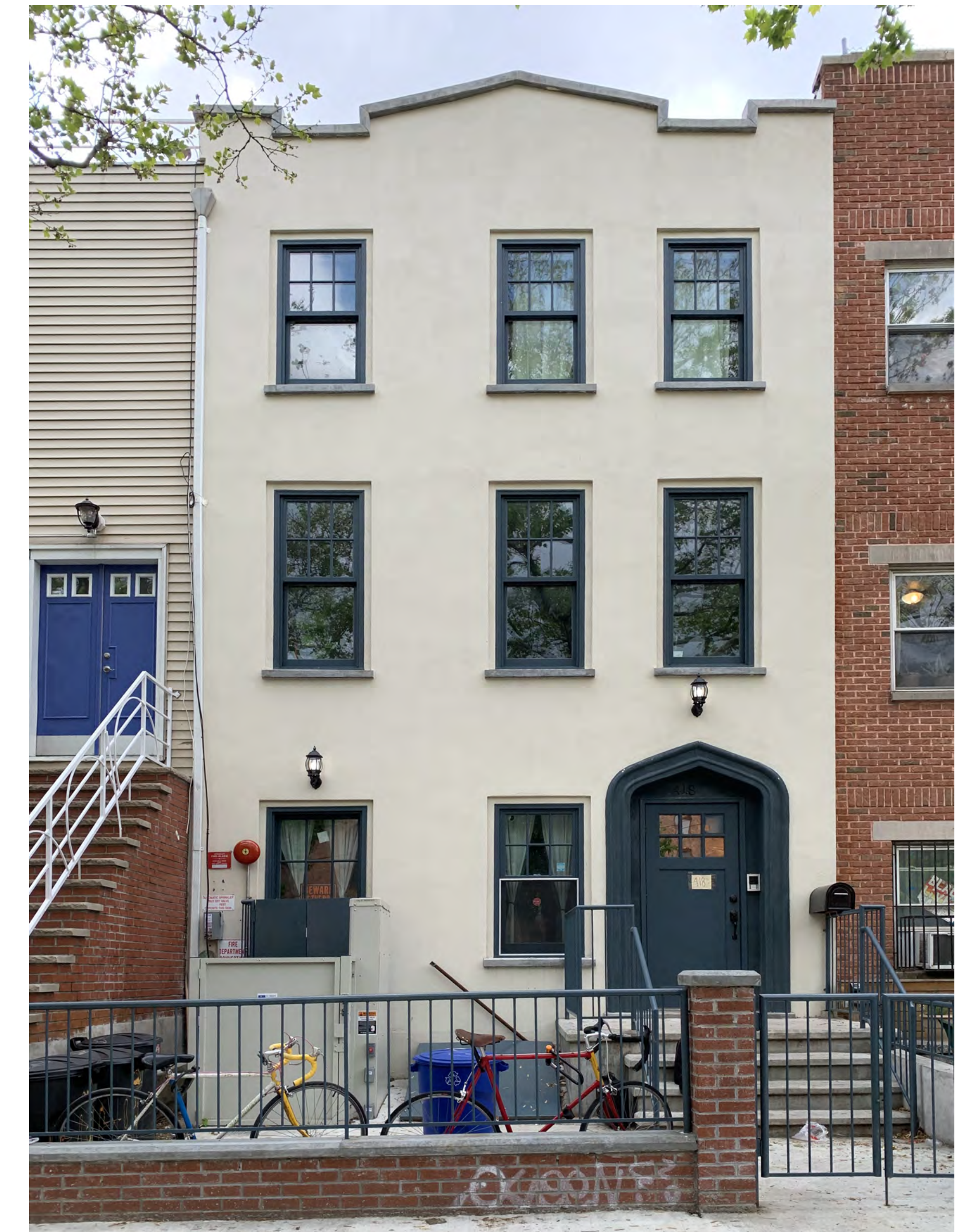
2022 AS-BUILT FRONT FACADE PHOTO 418 A LEWIS AVENUE BLOCK 1679 LOT 37
