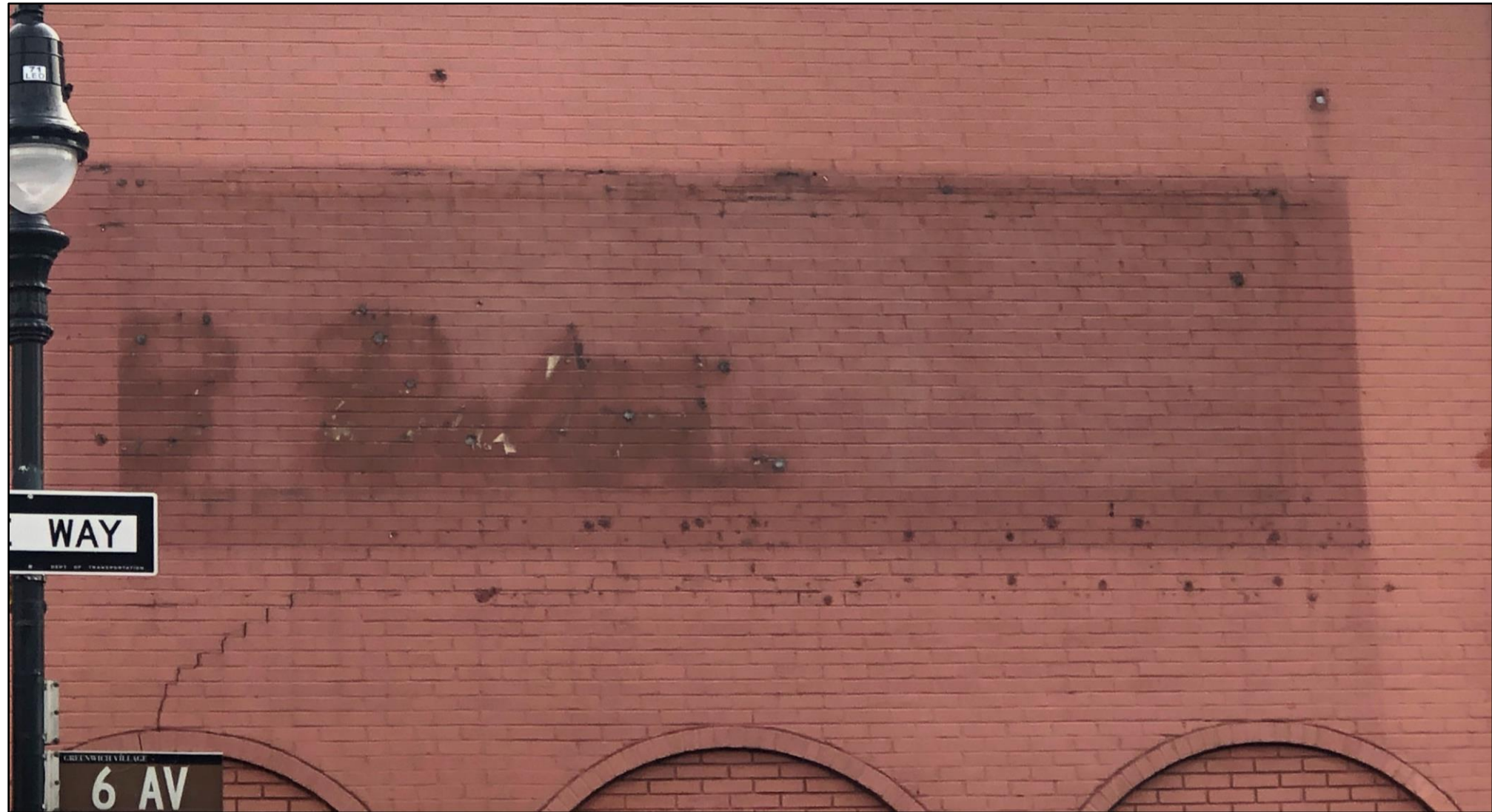
Existing condition at Sixth Avenue elevation, before the temporary banner was installed.
