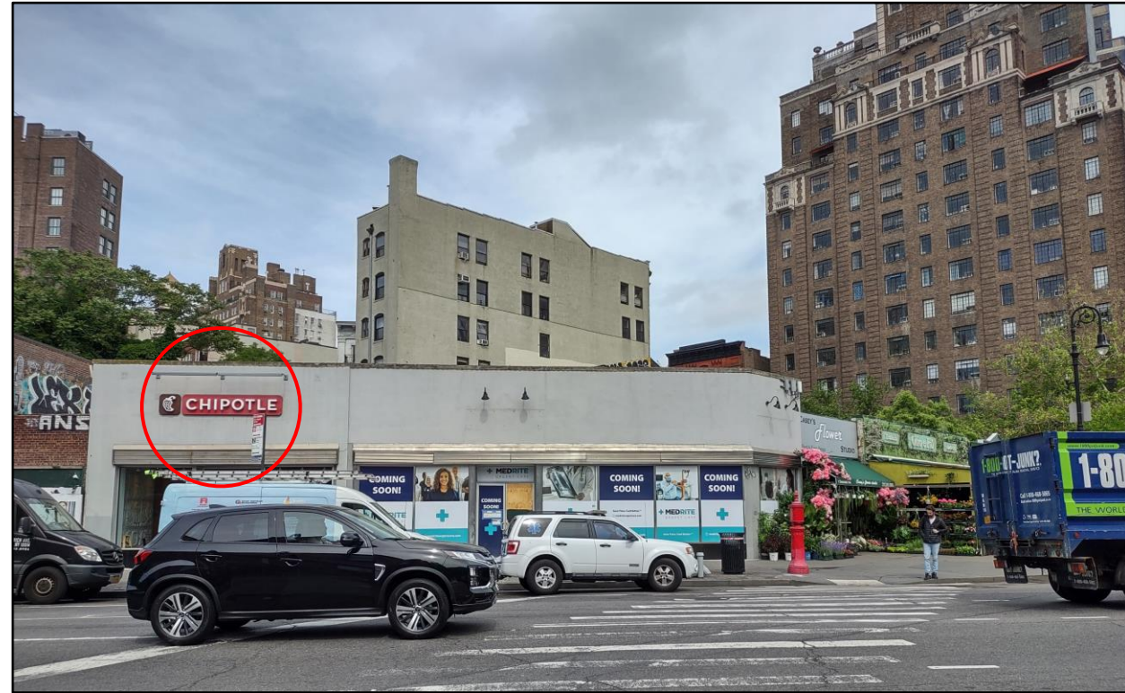
West side of Sixth Avenue, looking west from the intersection with West 8 th Street.
