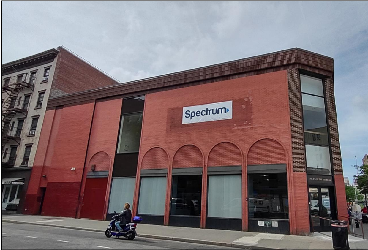
North elevation, on West 8 th Street, and chamfered corner.
