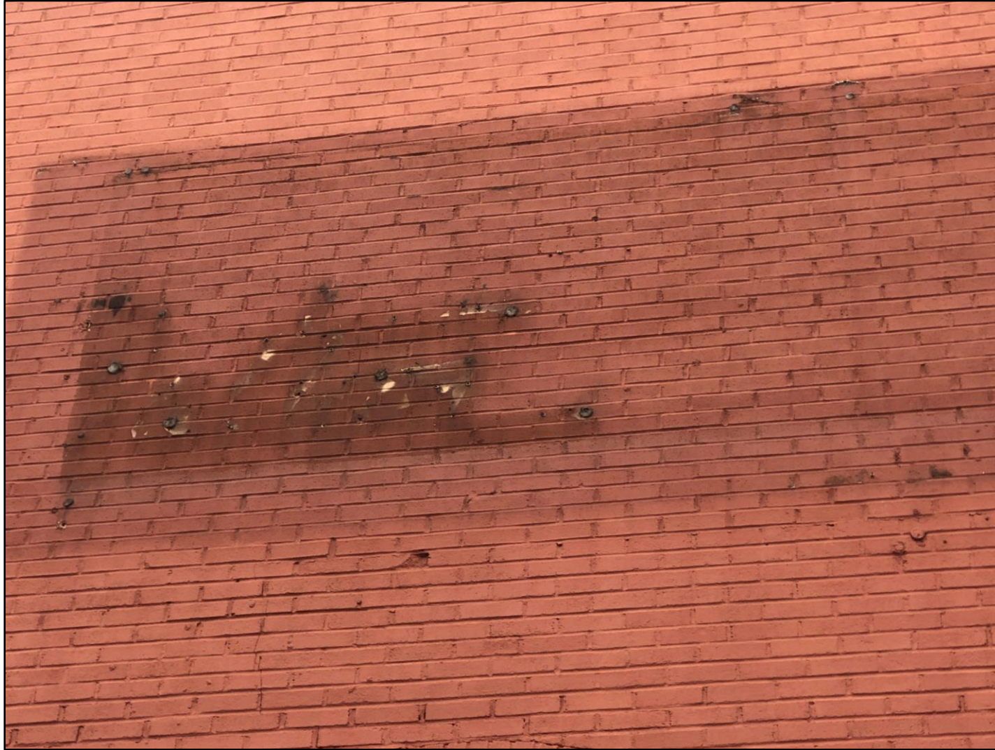
Existing condition at West 8 th Street elevation, before the temporary banner was installed.
