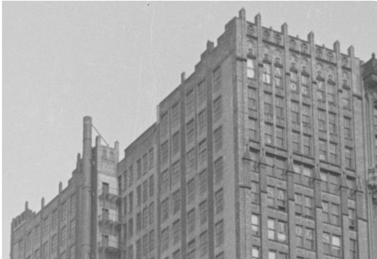
1940 view of the parapet. (LOC)
