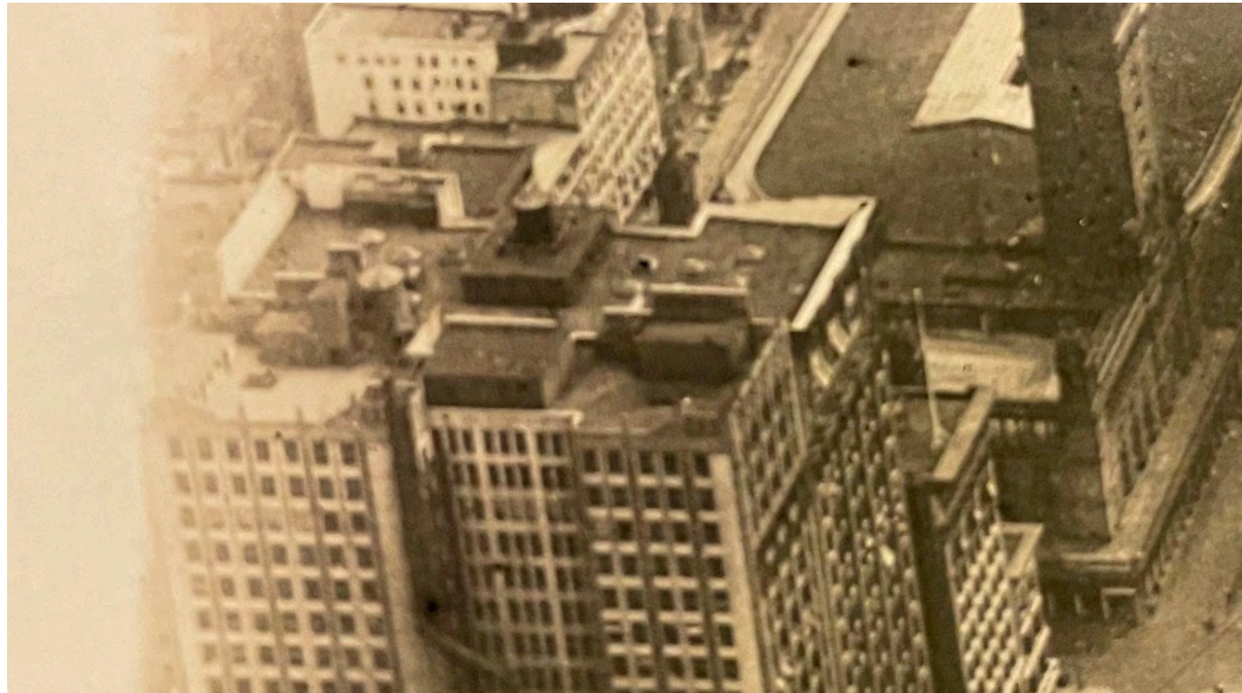
1922 view of the roof. (NYHS)
