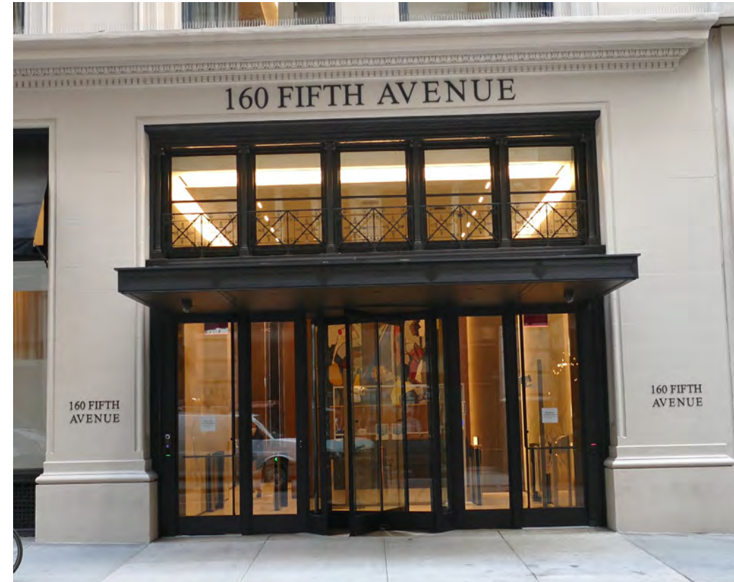
160 Fifth Ave, canopy & revolving door approved 2021.
