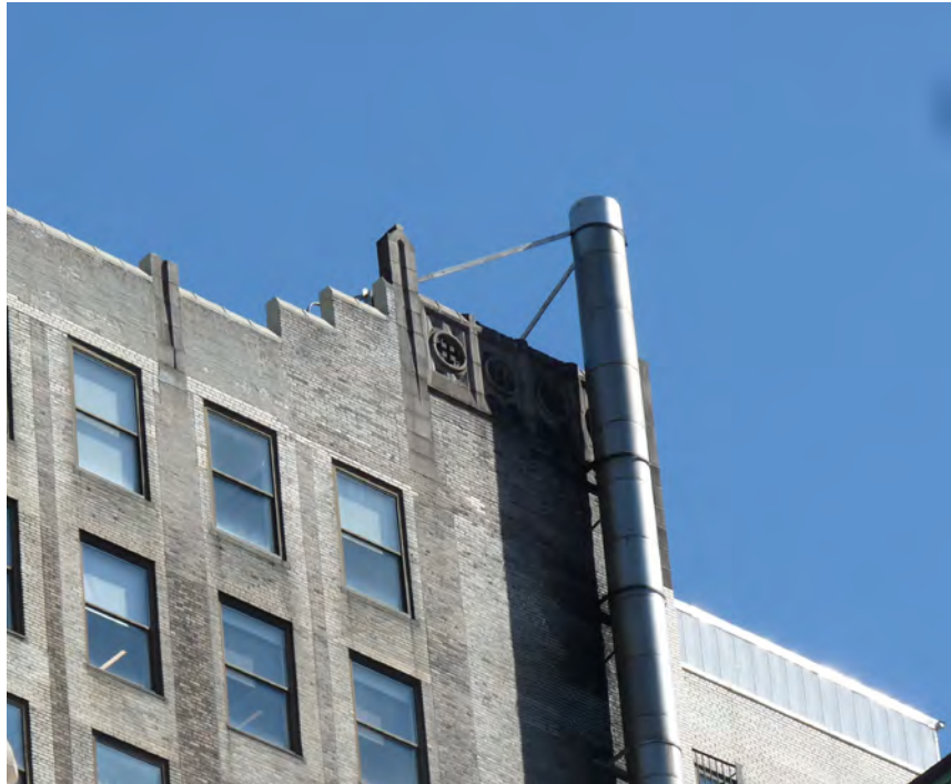
STAIR E BULKHEAD AT WEST PARAPET
