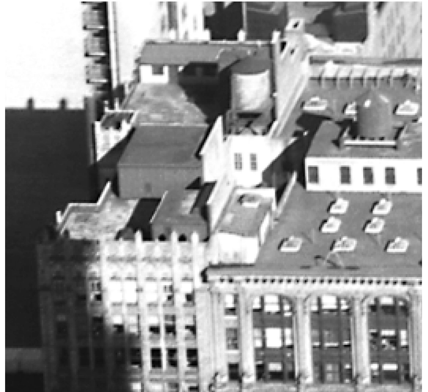
1951 view of the roof. (NYS)
