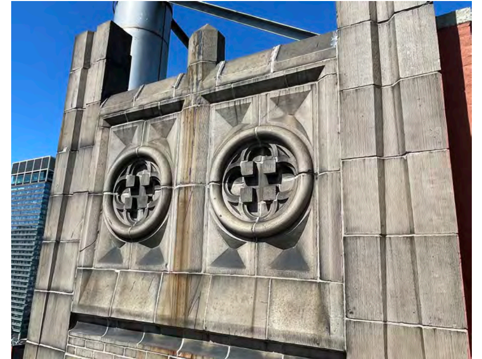
STAIR E BULKHEAD TERRACOTTA DETAILING
