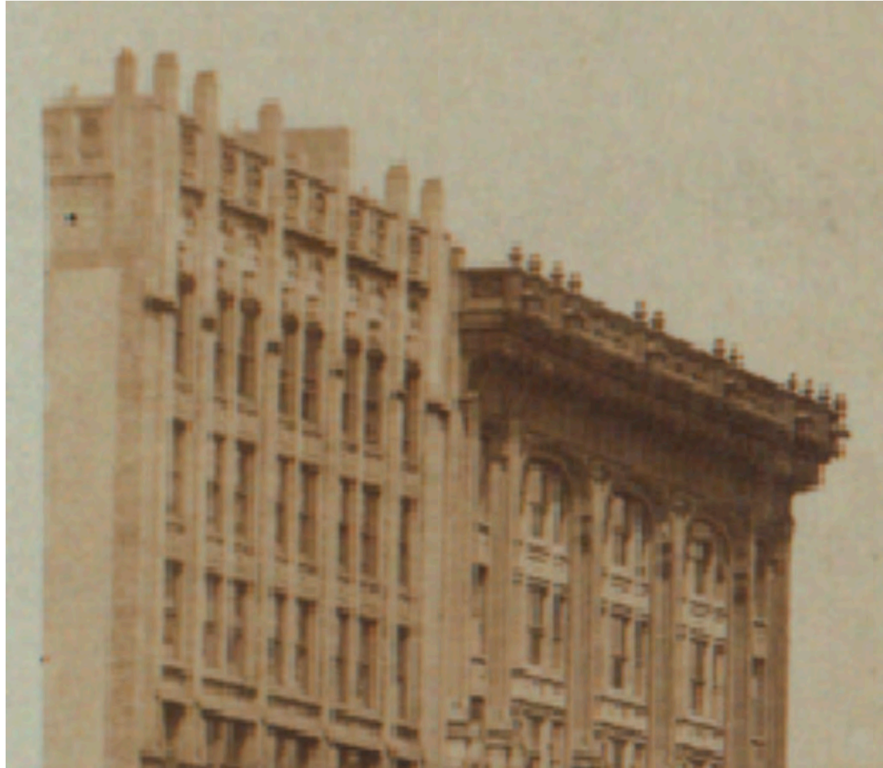
1924 view of the parapet. (NYPL)
