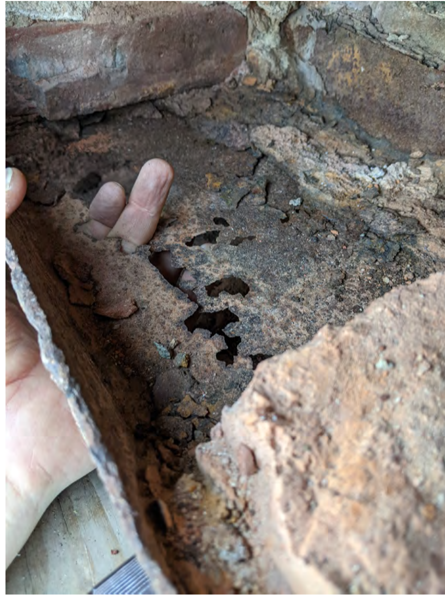
PROBE AT THE BACKUP WALL SHOWING THE EXISTING CORRODED STEEL POST AND BEAMS THAT SUPPORT THE TERRACOTTA CLADDING WALL. MARCH /2022.
