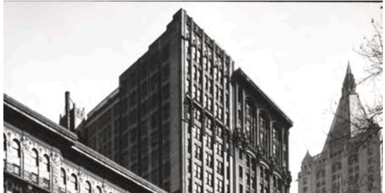
Ca. 1977 view of the parapet. (MCNY)
