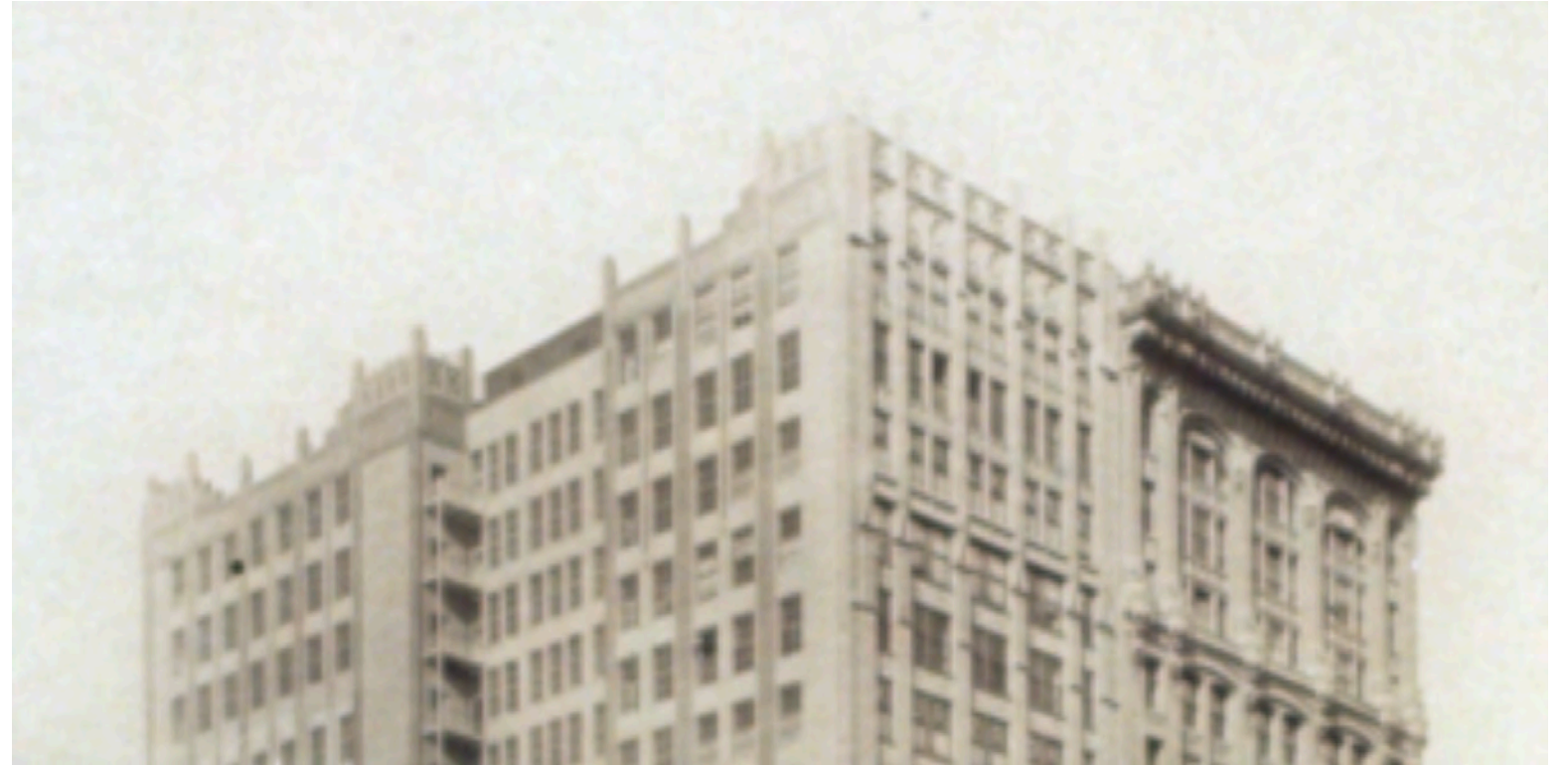
1913 view of the parapet. (LOC)
