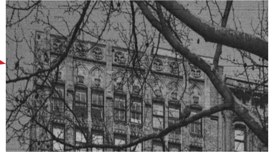
Parapet close-up view
