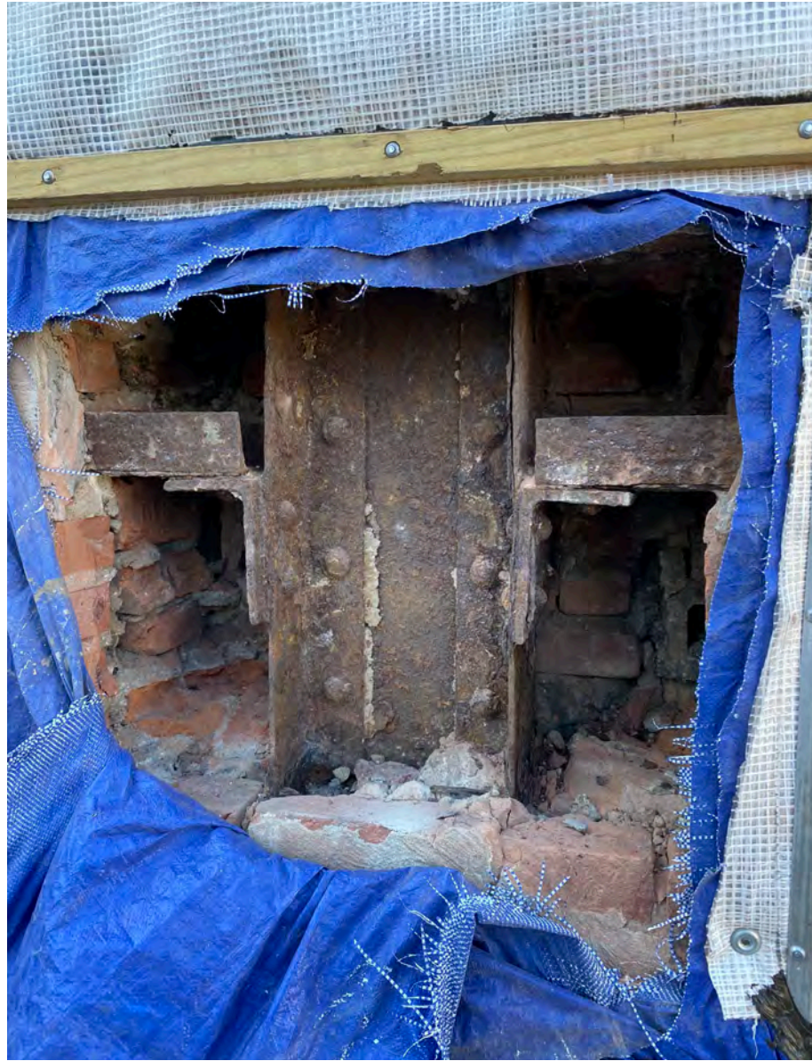
PROBE AT THE BACKUP WALL SHOWING THE EXISTING CORRODED STEEL POST AND BEAMS THAT SUPPORT THE TERRACOTTA CLADDING WALL. MARCH /2022.
