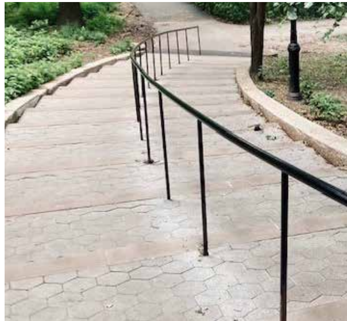
Simple Steel Handrail (Riverside Park)
