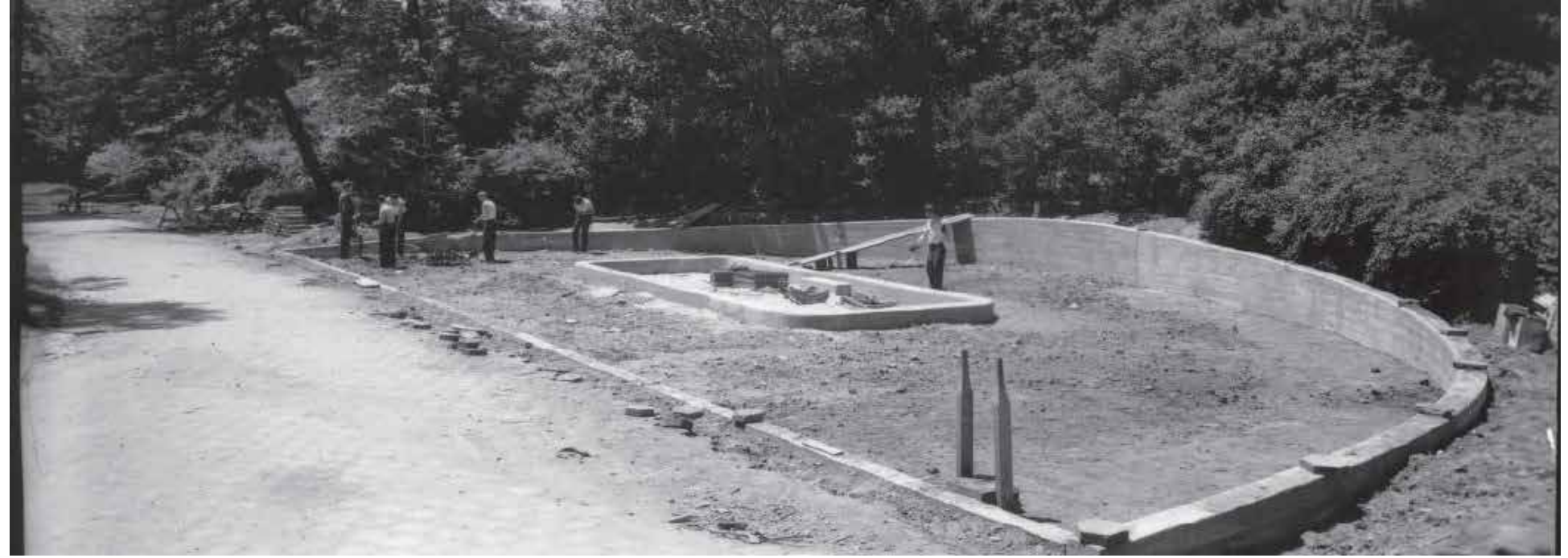
1941 Garfield Tot Lot under construction
