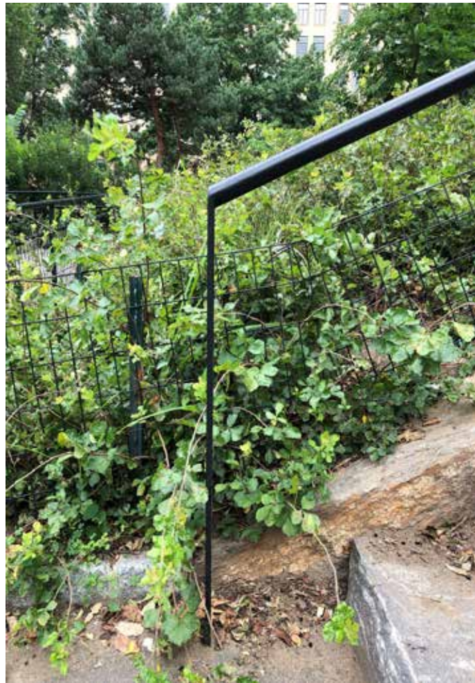
Simple Steel Handrail (Riverside Park)
