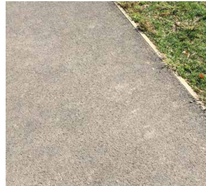
Full Depth Asphalt Pavement and Timber Edge
