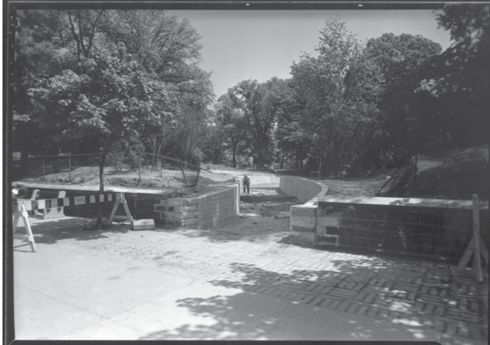
1941 Garfield Entrance under construction
