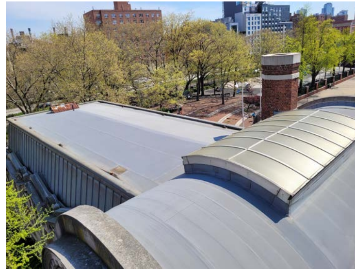
Main Building Roof
