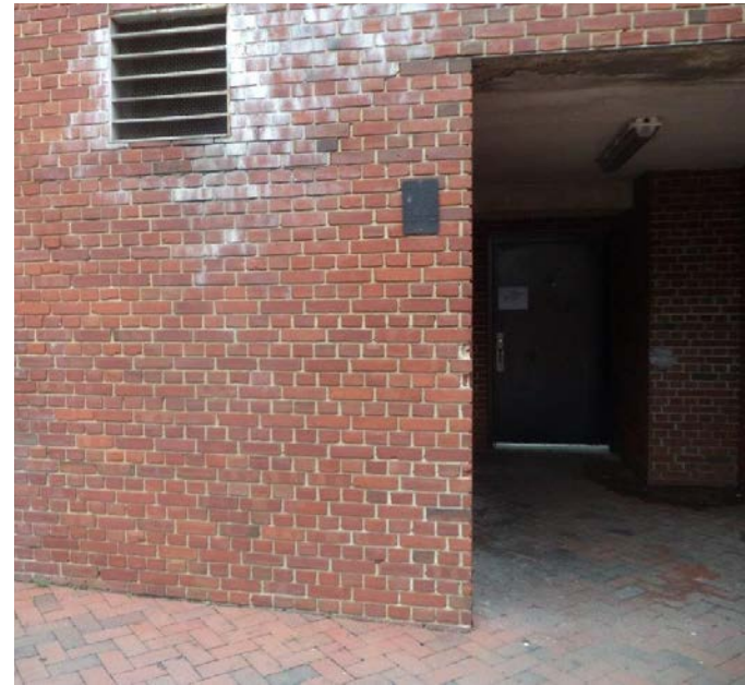
8 - Basement Egress South / Pool Bathroom Entrance
