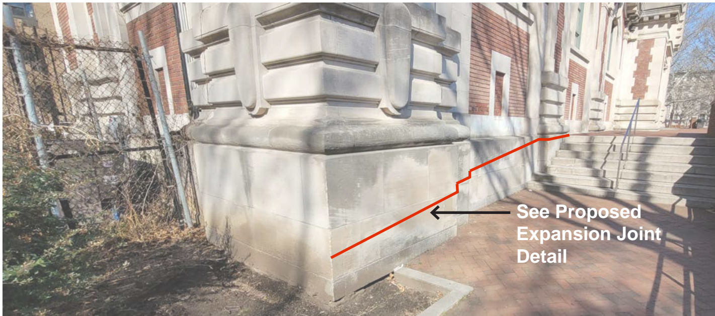
1 - Existing South Stair
