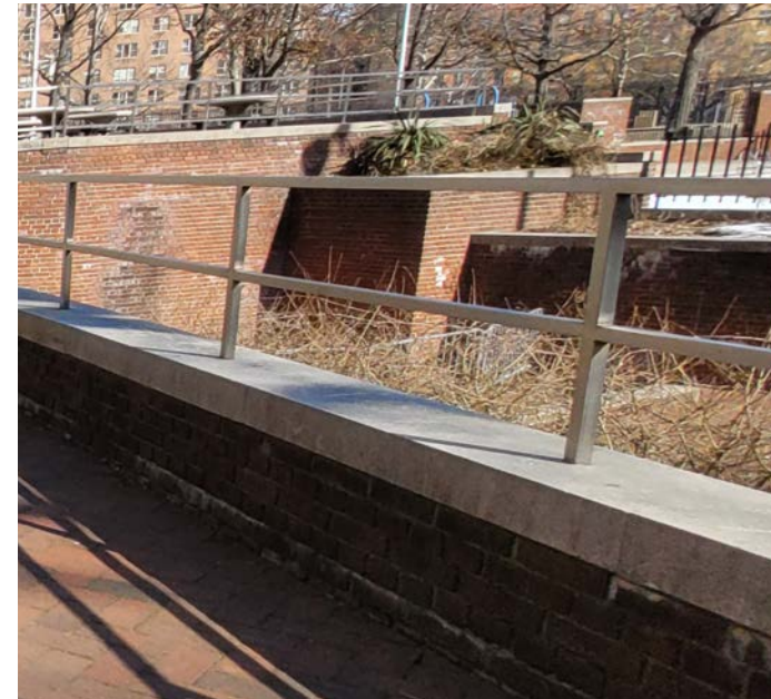
Existing Stainless Steel Guardrail on Parapet
