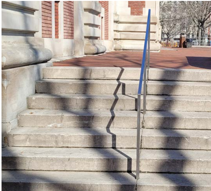
Existing Stainless Steel Handrails
