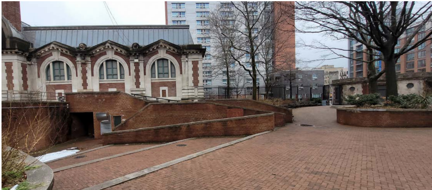
1 - Concrete Steps and Masonry Walls at West Elevation
