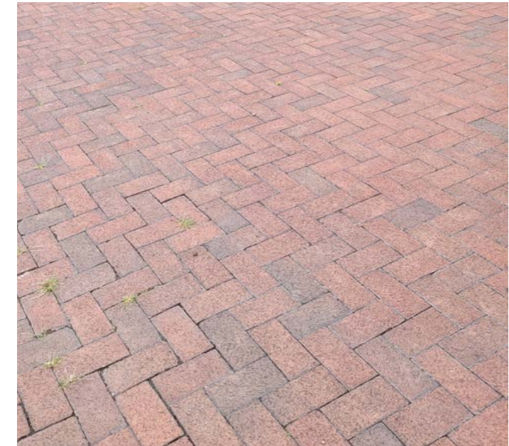
Existing Brick Pavers
