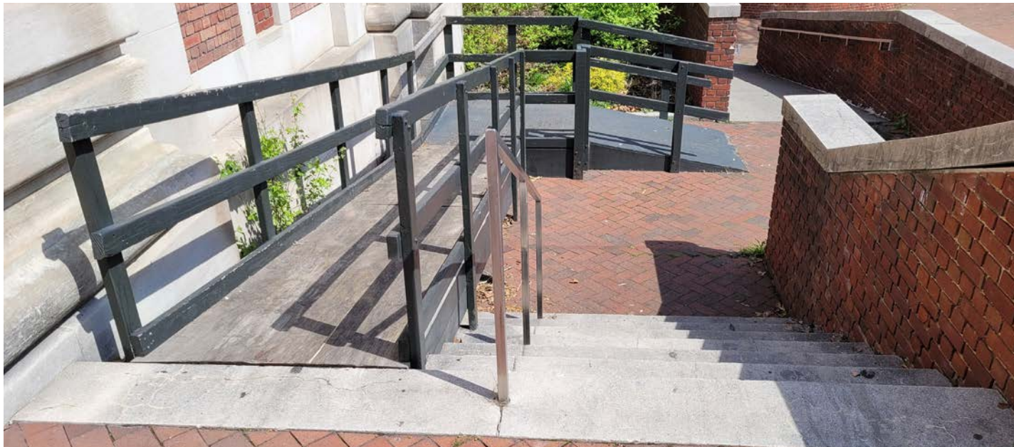
4 - Existing Non-Compliant Wood Ramp at North Stair
