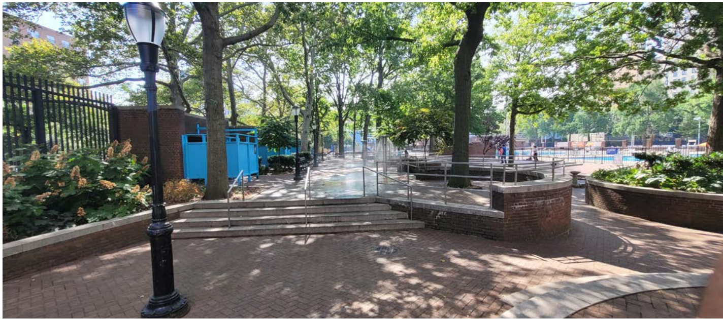
1 - Existing Stainless Steel Handrail and Guardrail near Playground
