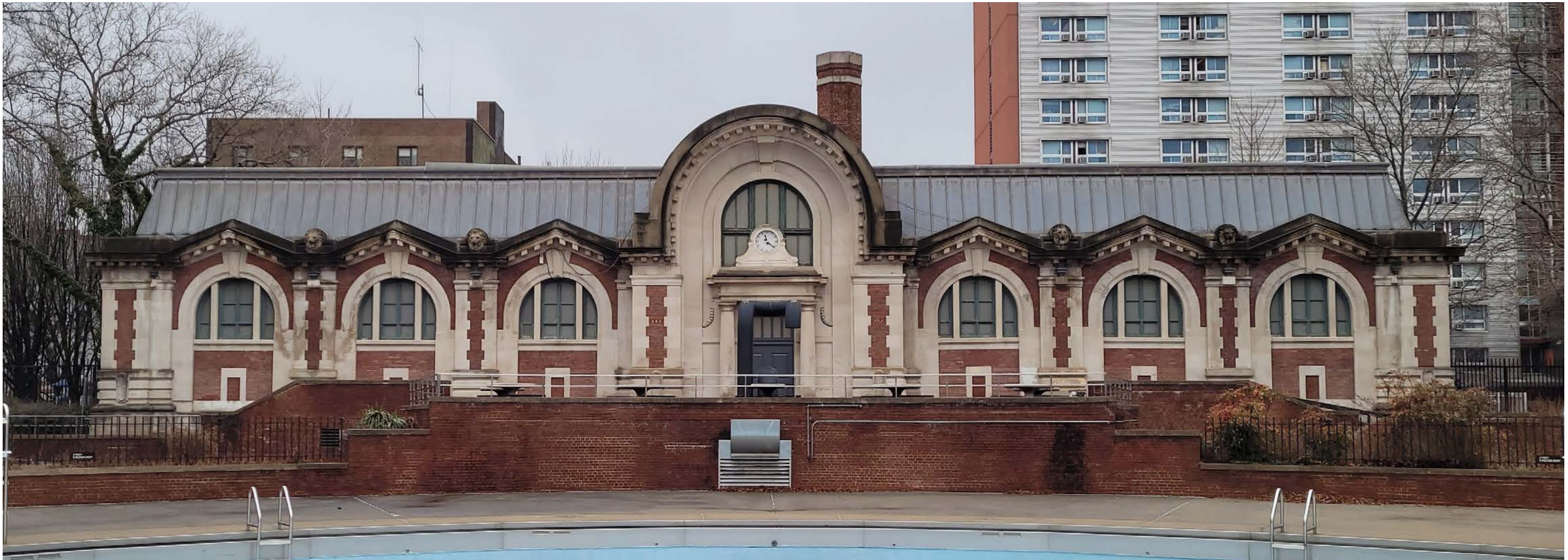
2 - Community Bldg. East Elevation and Park-Facing Entrance (from Pool Deck)
