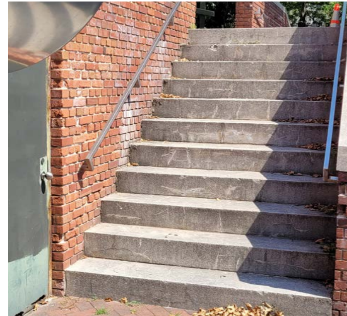
Existing Concrete Stairs
