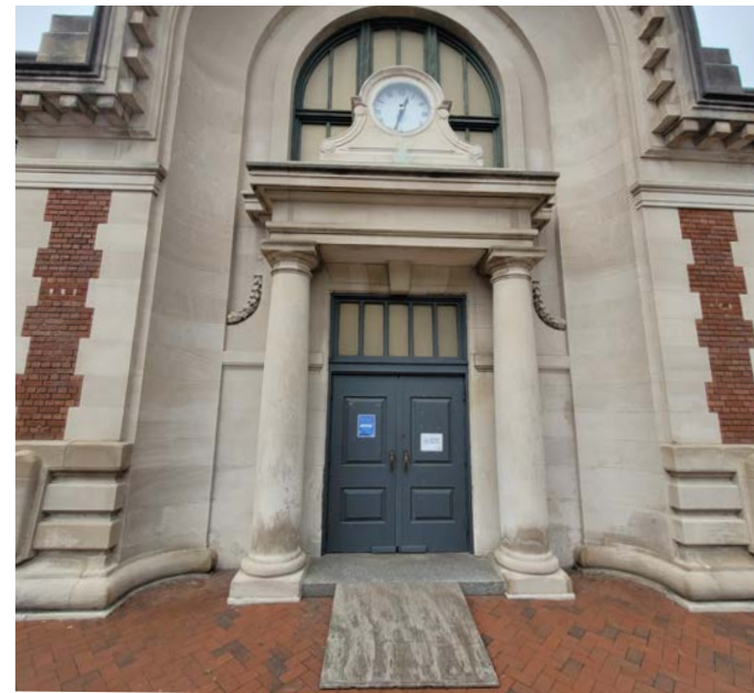
7 - Existing Non-Compliant Wood Ramp at East Entrance of Community Building
