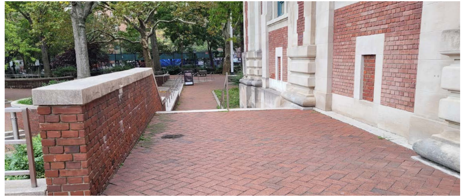
6 - Concrete Steps and Masonry Walls at West Elevation
