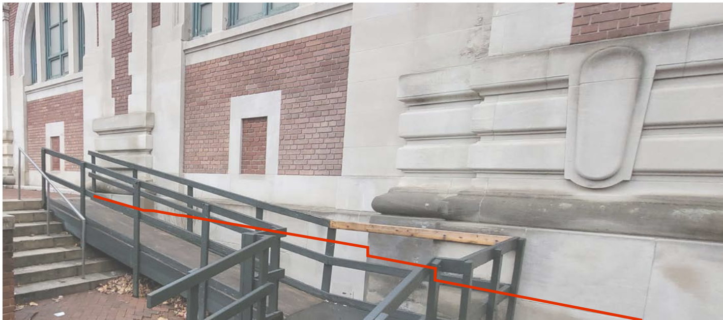
1 - Existing Freestanding Wood Ramp at North Stair
