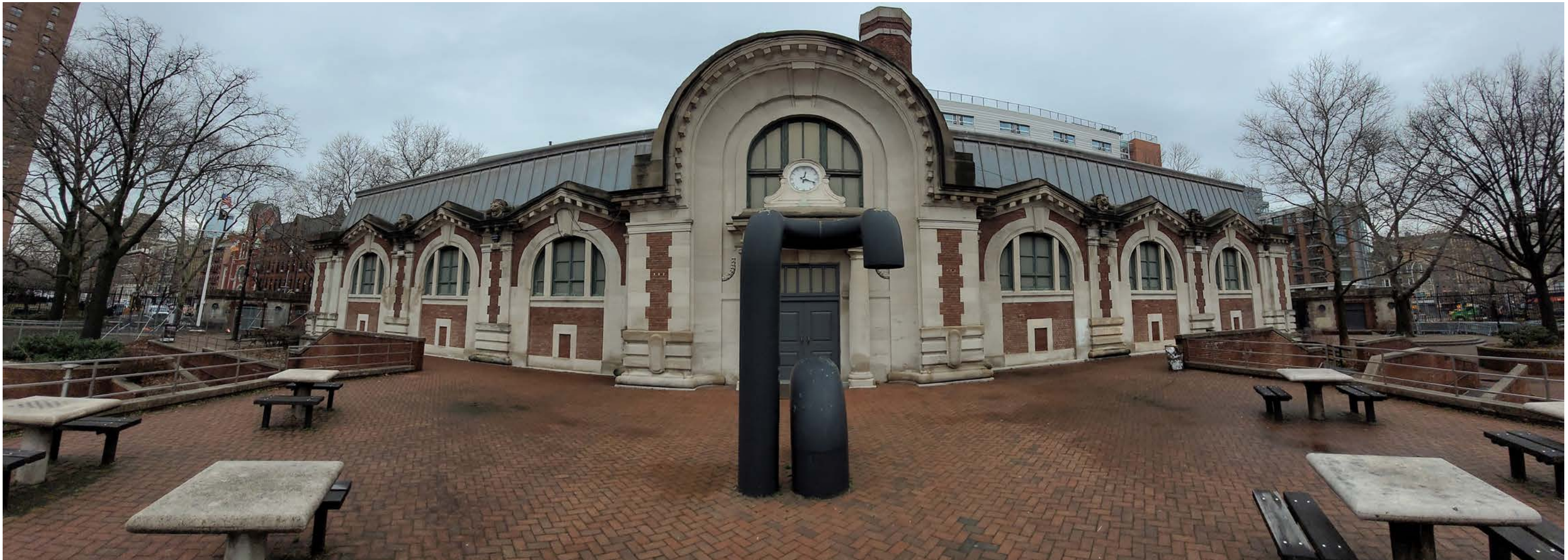
3 - Community Bldg. East Elevation (from Terrace)
