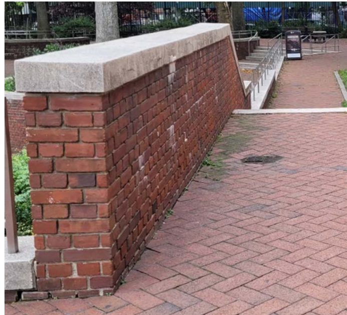
Brick wall with Precast Limestone Coping
