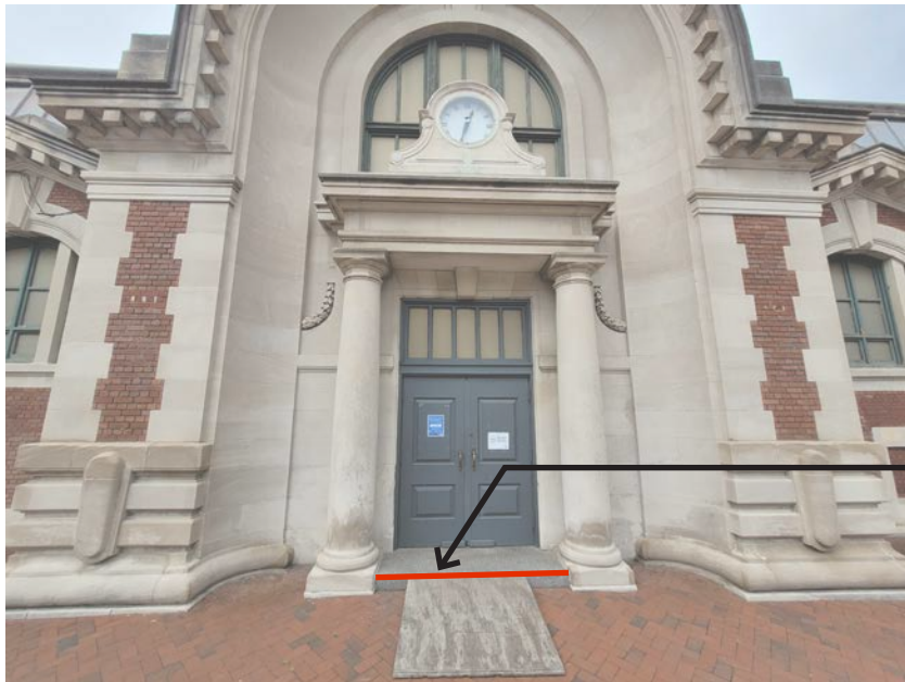
1 - Existing Freestanding Wood Ramp at East Entrance
