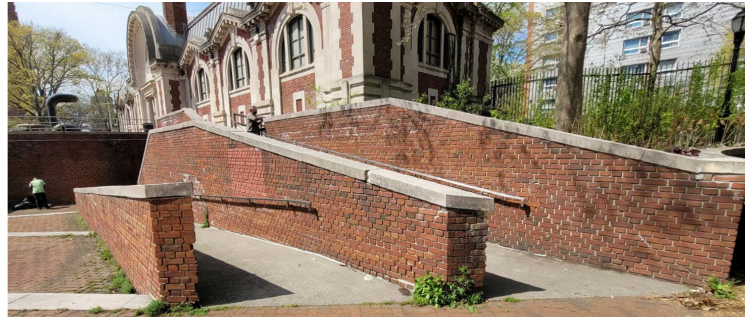
2 - Concrete Ramps to Basement and 1st Floor
