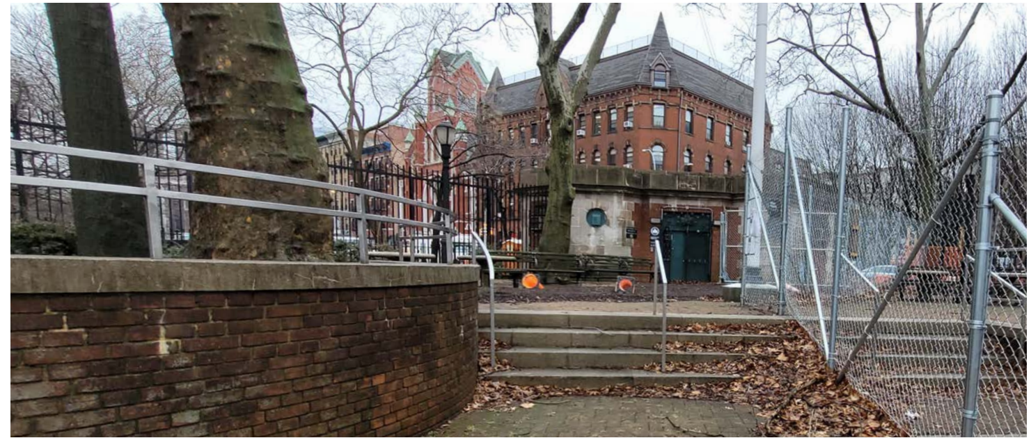
2 - Existing Stainless Steel Handrail and Guardrail near Stanton Street House
