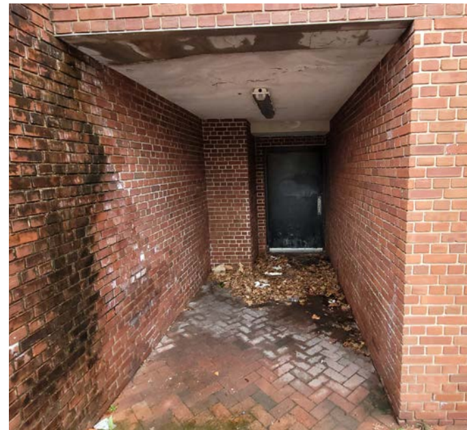
4 - Basement Egress North
