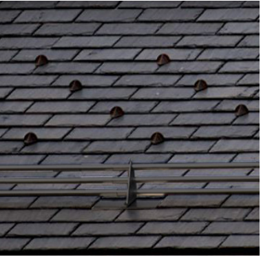
SNOW GUARD: ALPINE SNOW GUARD HALF ROUND PAD STYLE IN COPPER AT UPPER ROOF THREE PIPE STYLE POWDER COATED IN COLOR BLACK AT EVE
