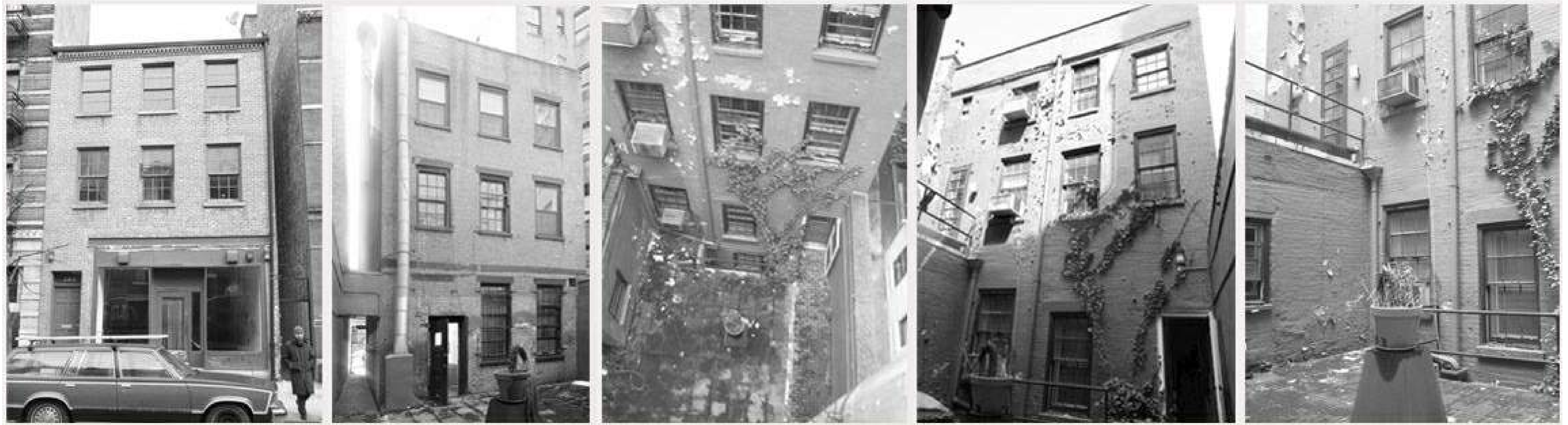
263 WEST 12 th STREET, PRIOR TO RENOVATION IN THE 1990's
