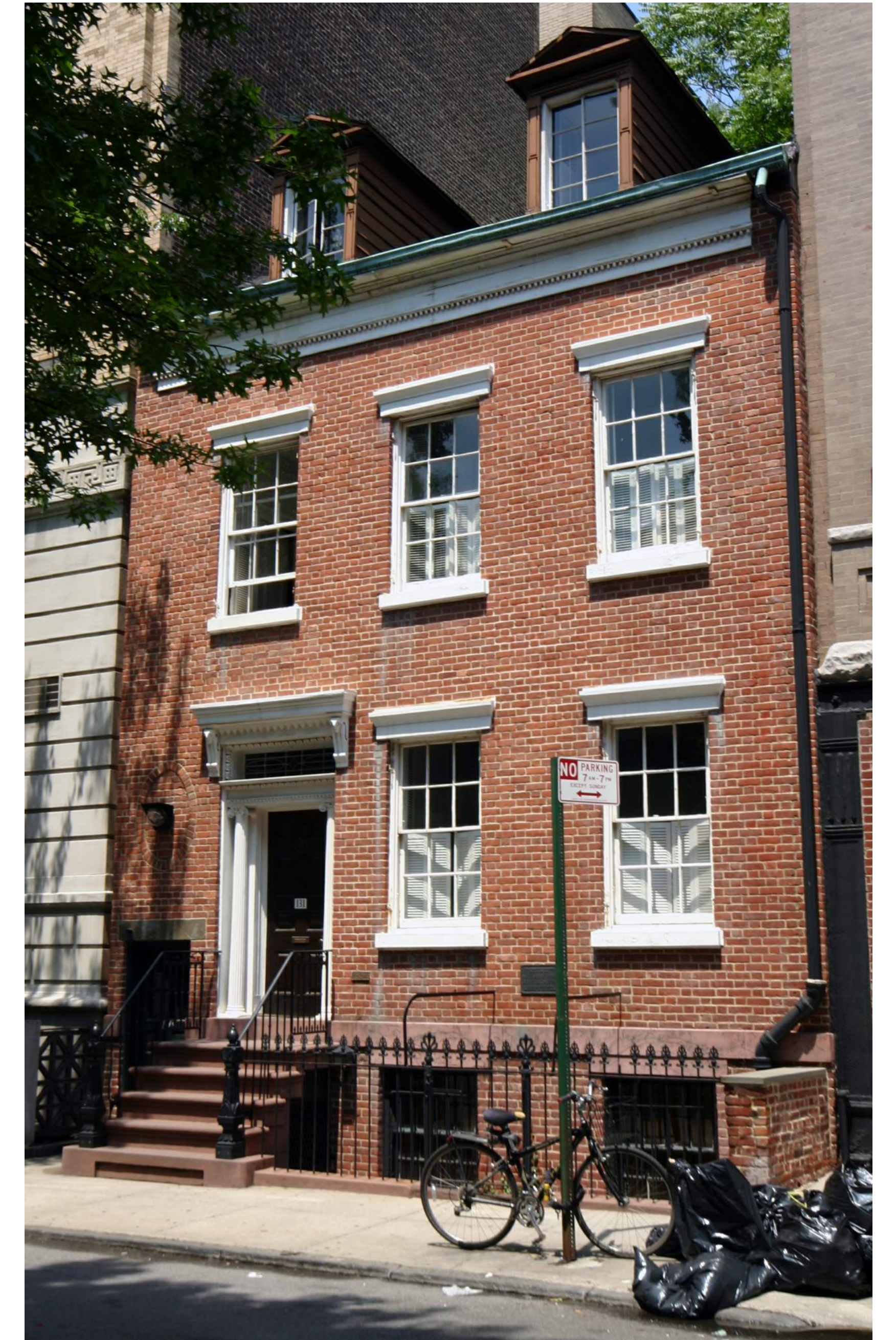
2006: 131 GREENWICH STREET DESIGNATION PHOTO (NYC LPC)
