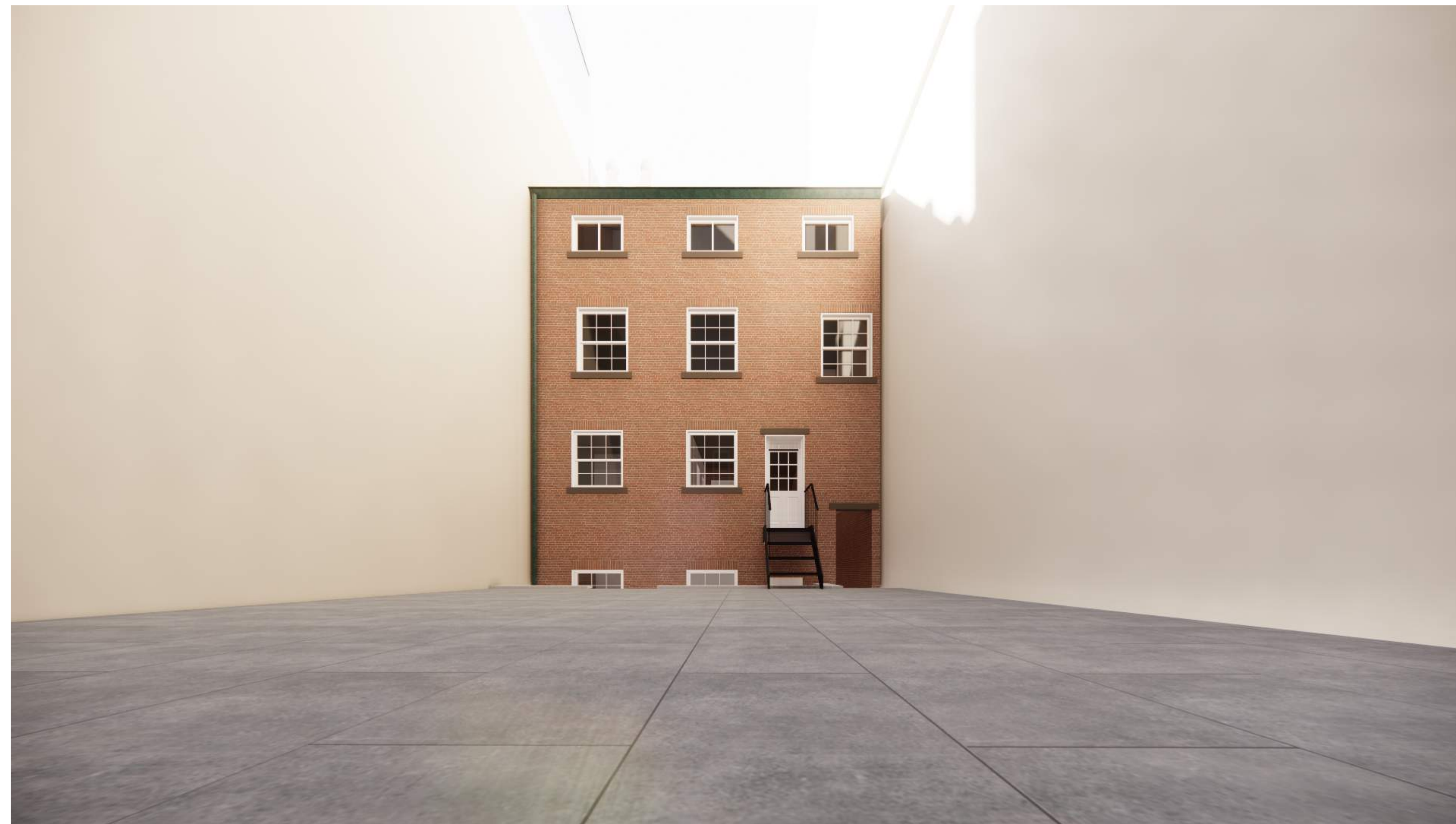
EXISTING REAR FACADE OF FRONT BUILDING
