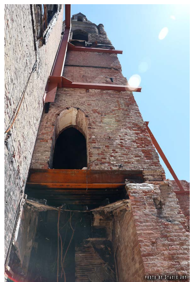
NORTH TOWER BRACING
