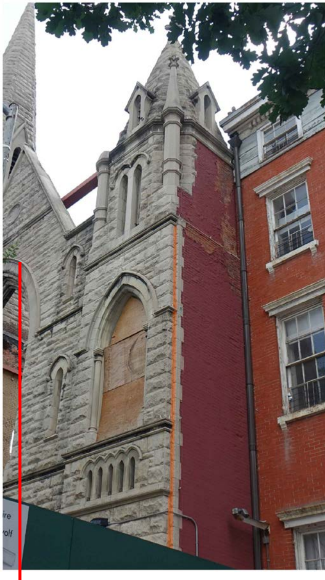
8. SOUTH TOWER – EXTENT OF LIMESTONE CRACK
