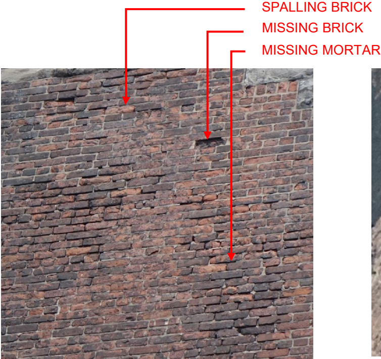
REPRESENTATIVE IMAGE OF DETERIORATED MASONRY SOUTH TOWER
