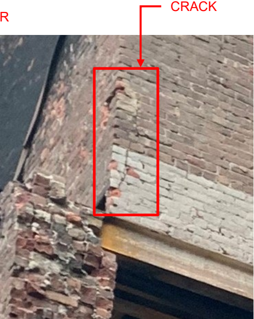
CRACK AT STEEL TRANSFER
