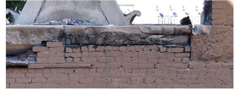
GABLE SILL FRACTURED STONE
