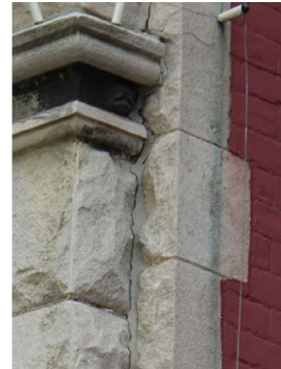
8. SOUTH TOWER – CRACK ENLARGED
