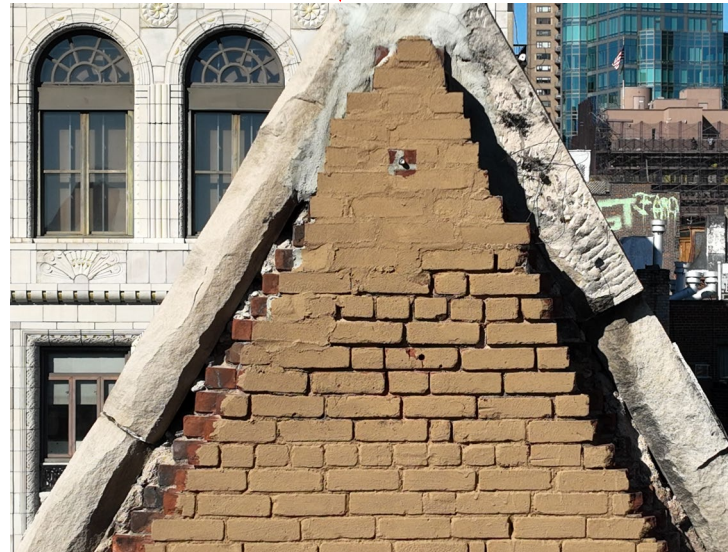
GABLE COPING DAMAGED STONE
