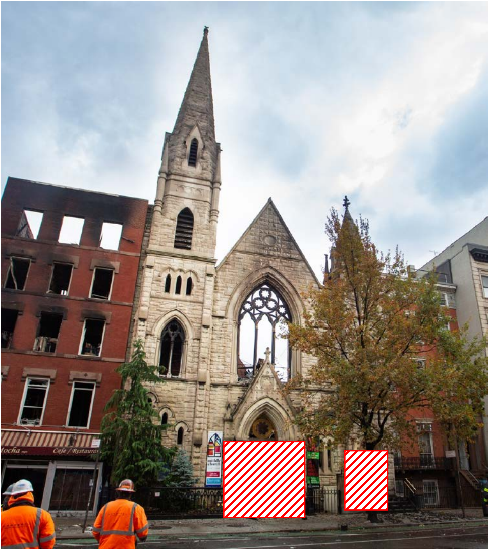
2 ND Ave. FAÇADE MODIFICATIONS REQUIRED FOR EGRESS BY NYC CODE
