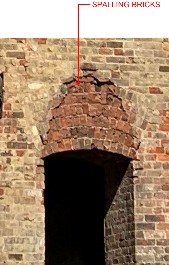
DETERIORATED MASONRY
