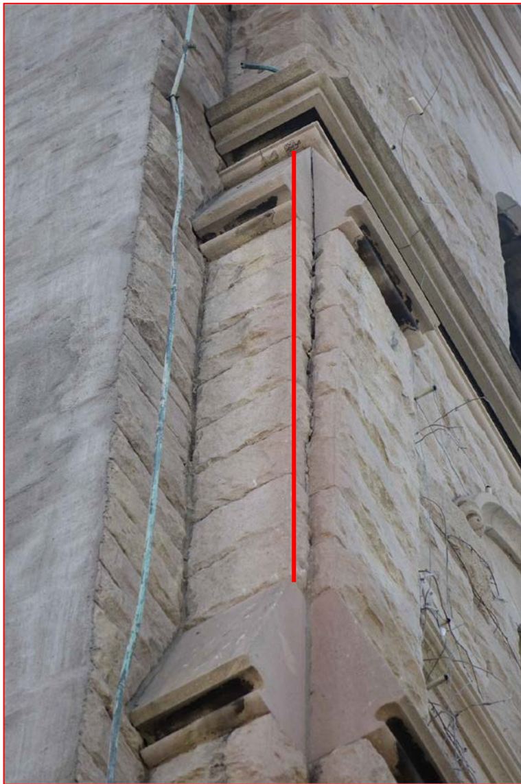
7. NORTH TOWER – EXTENT OF LIMESTONE CRACK
