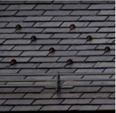
SNOW GUARD: ALPINE SNOW GUARD HALF ROUND PAD STYLE IN COPPER AT UPPER ROOF THREE PIPE STYLE POWDER COATED IN COLOR BLACK AT EVE
