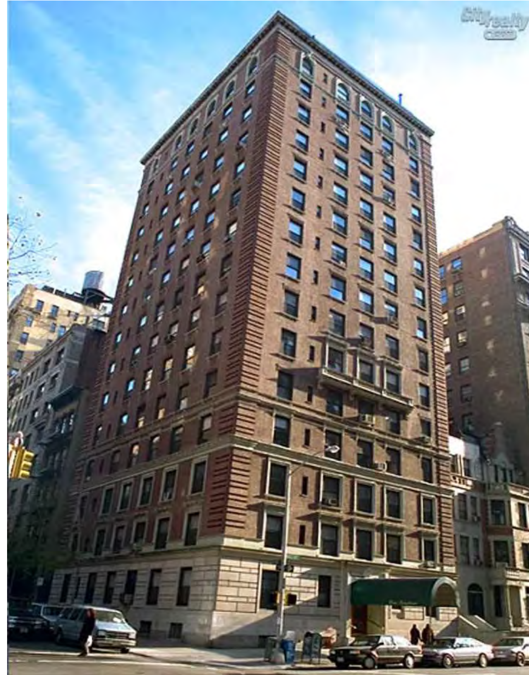
FRONT FACADE IN 1980'S
