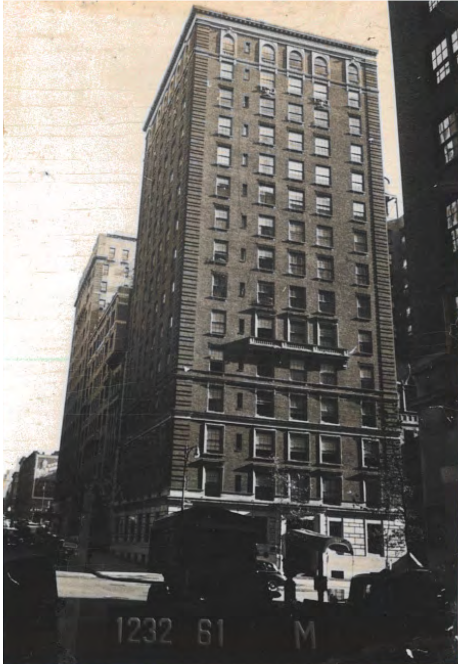
FRONT FACADE IN 1940'S
