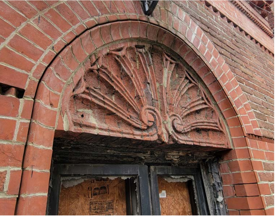
EXISTING SHELL BRICKWORK DETAIL
