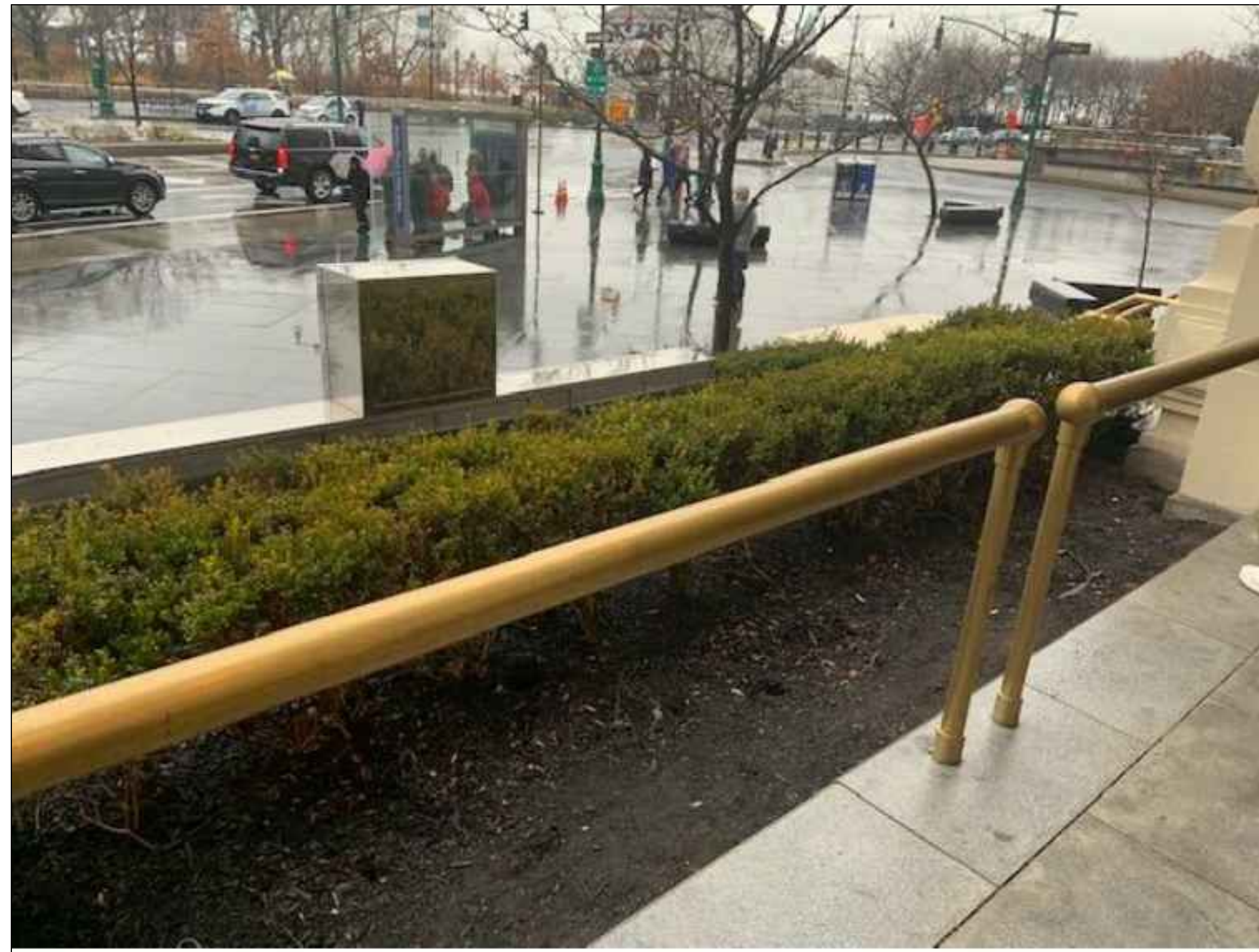
2 SOUTHERN FACADE- RAILING IMAGE Scale: NTS
