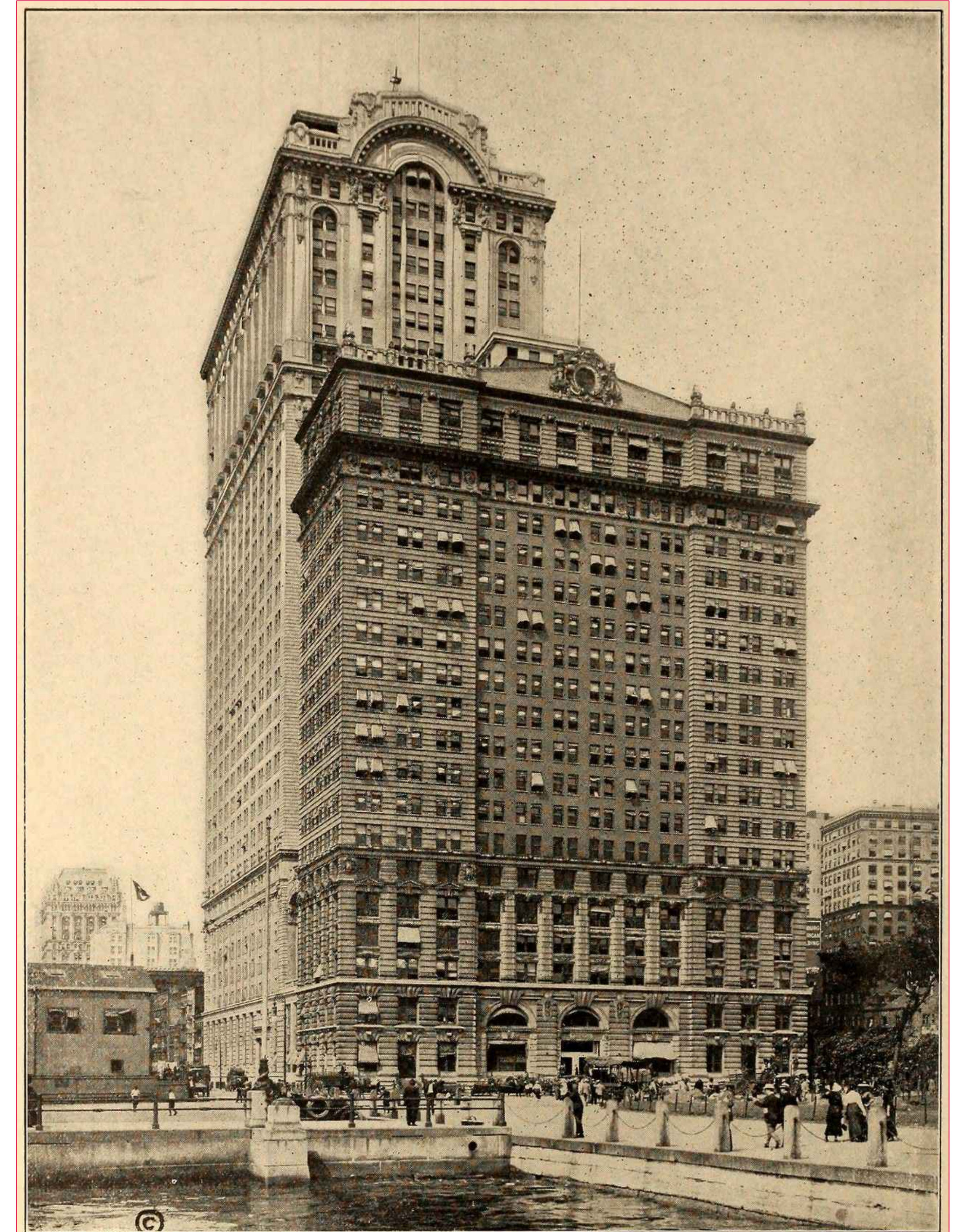
Whitehall Buildings , on Battery Place, between West and Washington Streets, the largest single office building in the world. The original building, 20 stories, 254 feet high, was finished in 1903 at a cost of $1,000,000; the new addition of 32 stories, 416 feet high, was finished in 1911, and cost $4,600,000. The building covers 21 city lots. Home of the Weather Bureau and of the Millionaires' Club.
