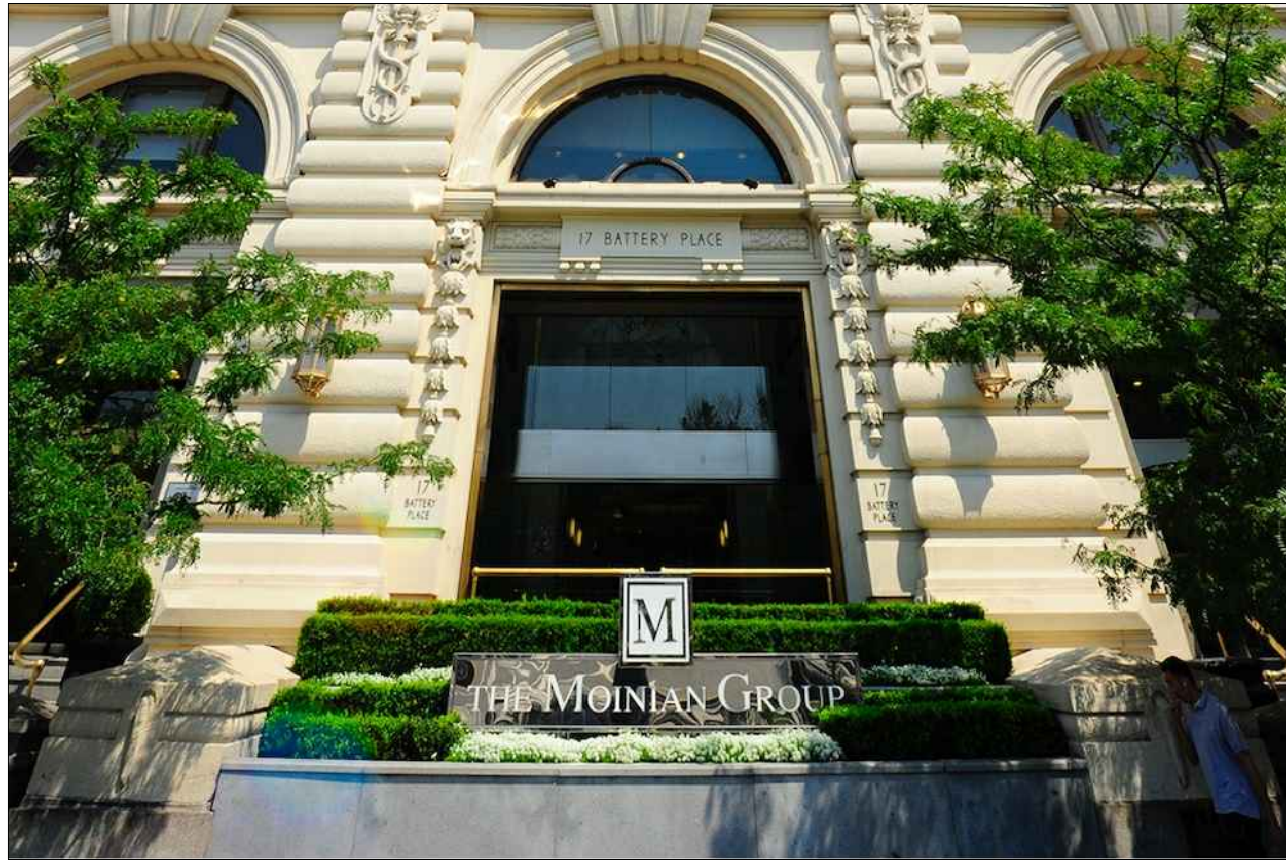
1 SOUTHERN FACADE- RAILING IMAGE Scale: NTS
