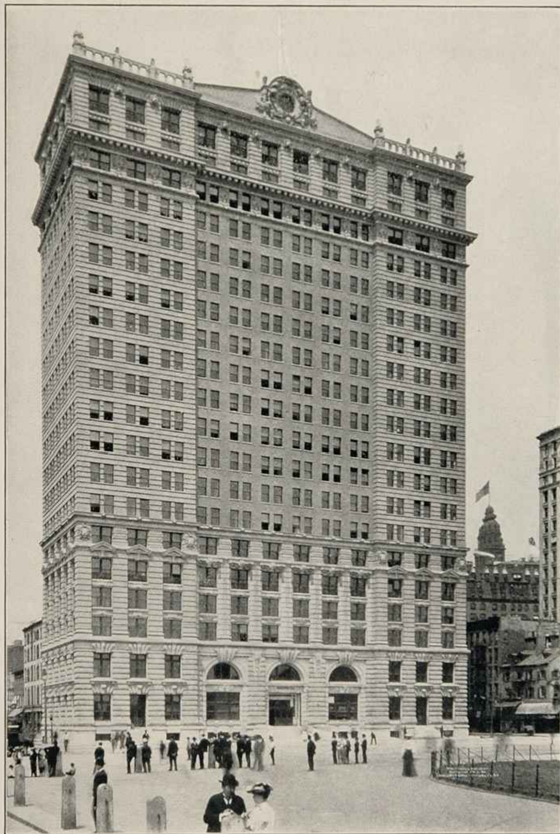
Henry J. Hardenbergh, Arch't Whitehall Building Battery Place Realty Co. WHITEHALL BUILDING , Battery Place, West and Washington Streets. Occupies a commanding site overlooking Park, Harbor and Hudson River. Twenty-story office-building. Steel, granite and brick. 440 offices. Owned by Battery Place Realty Co., Wm. H. Chesebrough, Pres.
