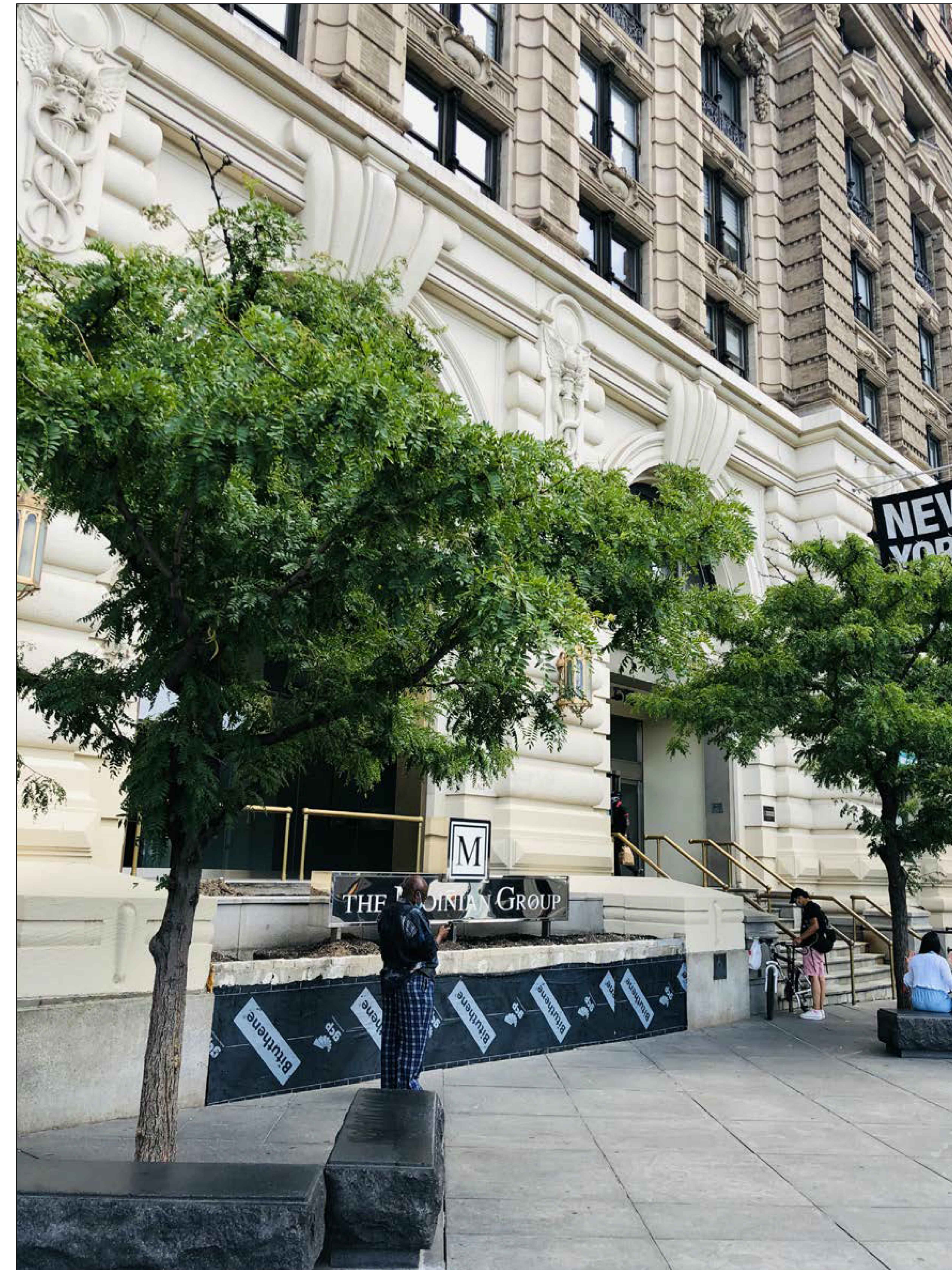
3 SOUTHERN FACADE- RAILING IMAGE Scale: NTS
