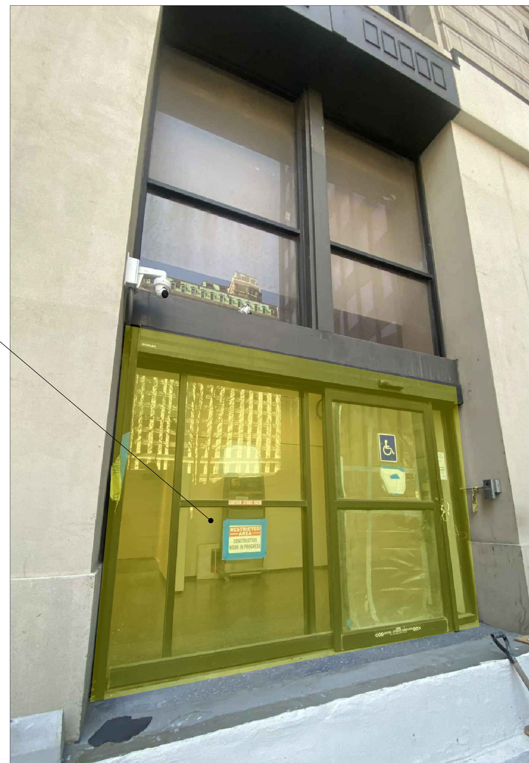
B EXISTING EASTERN FACADE Scale: NA
