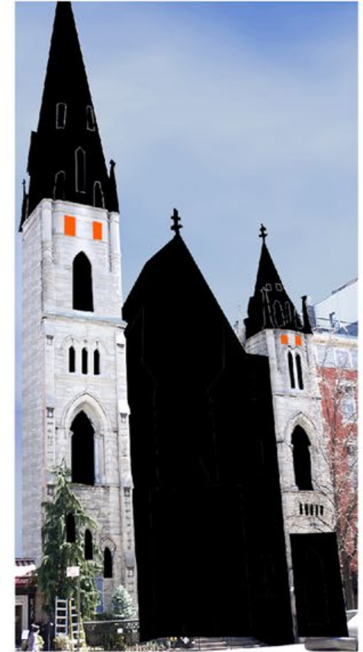
MINIMUM OF MATERIALS DAMAGED OR TO BE REMOVED FOR SAFETY
