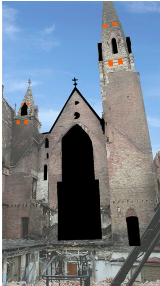
ORIGINAL MATERIALS LOST IN FIRE OR REMOVED FOR EGRESS & SITE ACCESS
