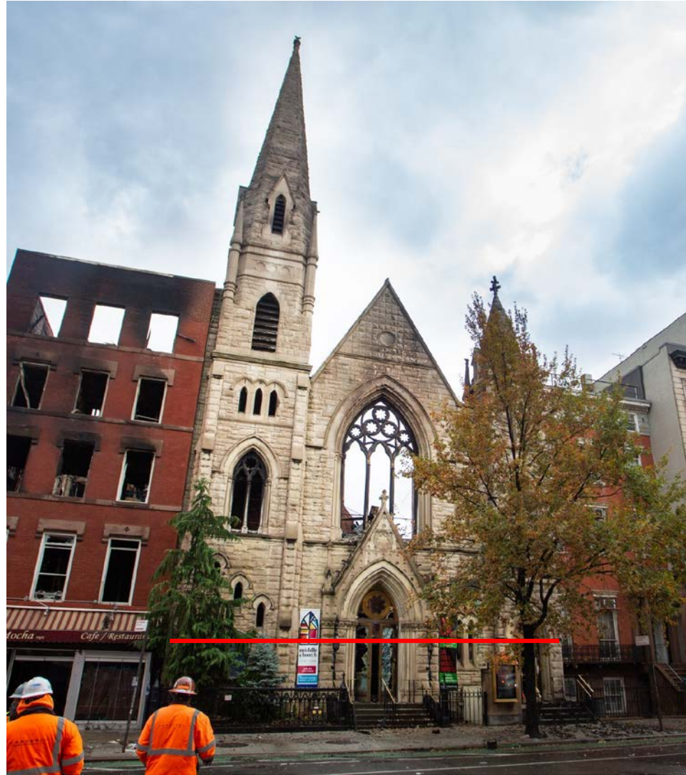
POSSIBLE SALVAGE OF STONE BELOW 8'-0"
