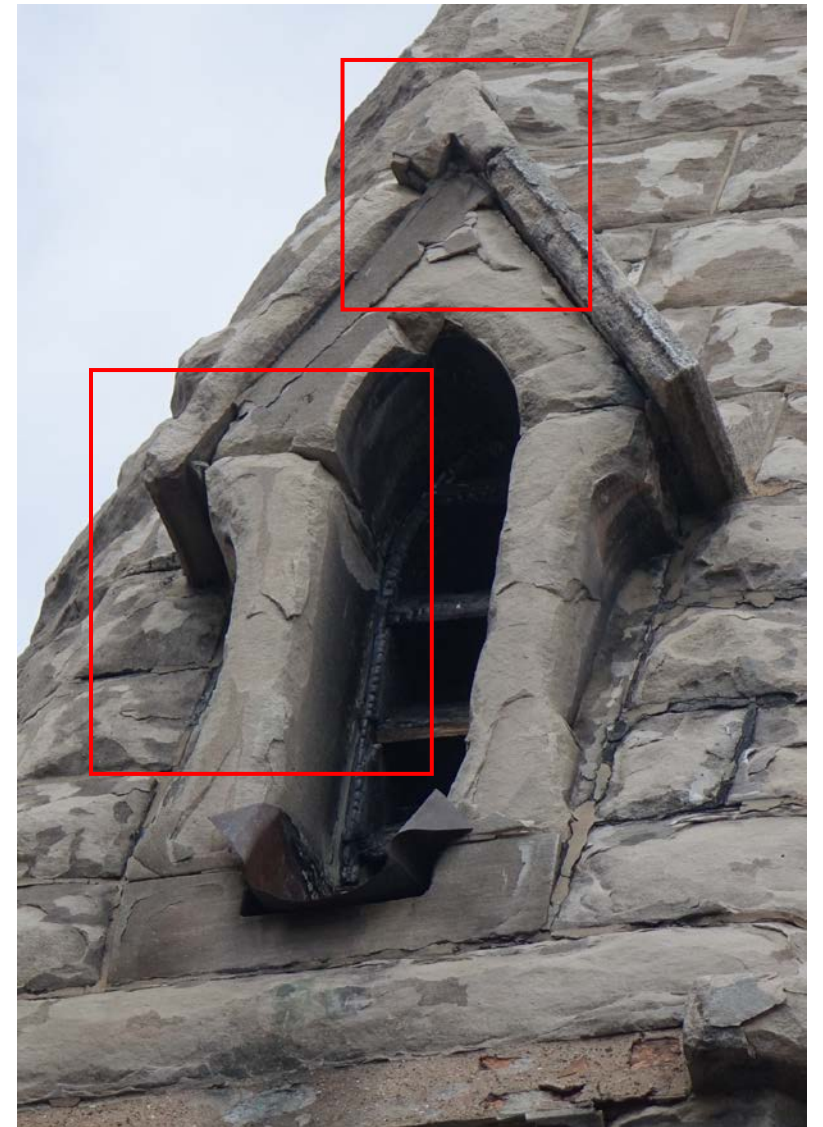
SOUTH SPIRE POST-FIRE
