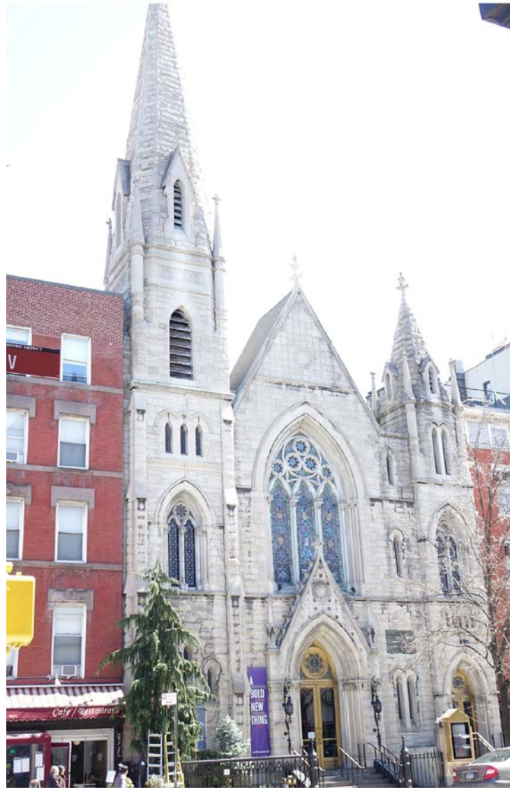
2 nd Ave. FAÇADE – PRE FIRE
