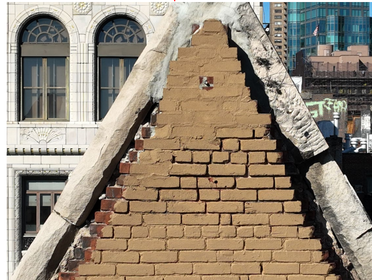
GABLE COPING DAMAGED STONE
