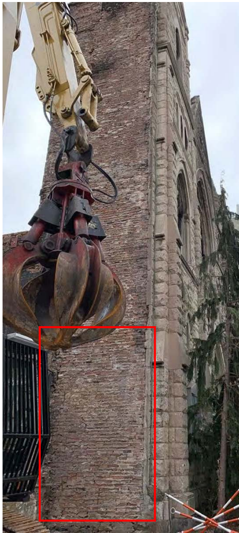
NORTH TOWER – NORTH WALL
