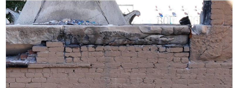
GABLE SILL FRACTURED STONE
