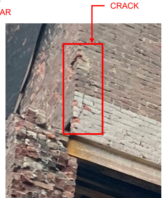
CRACK AT STEEL TRANSFER
