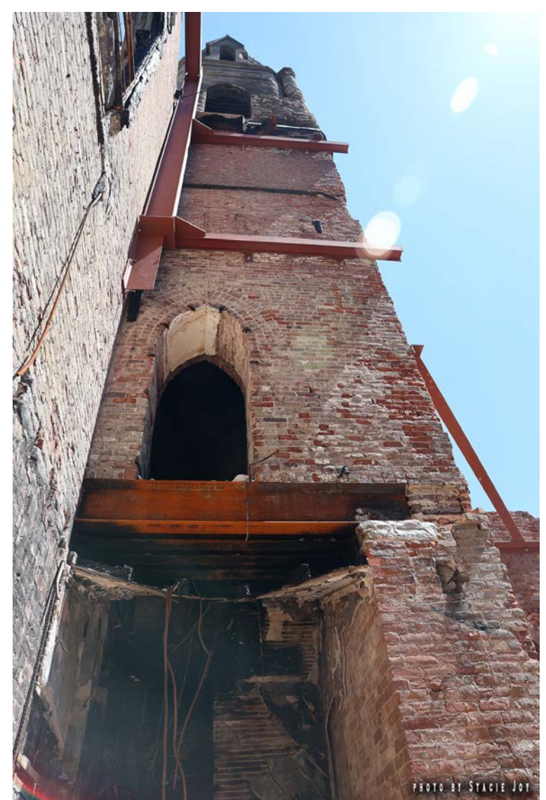
NORTH TOWER BRACING
