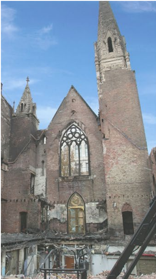
FACADE AFTER FIRE
