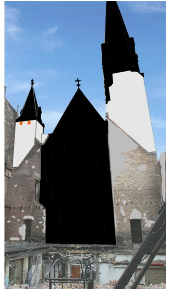
MINIMUM OF MATERIALS DAMAGED OR TO BE REMOVED FOR SAFETY
