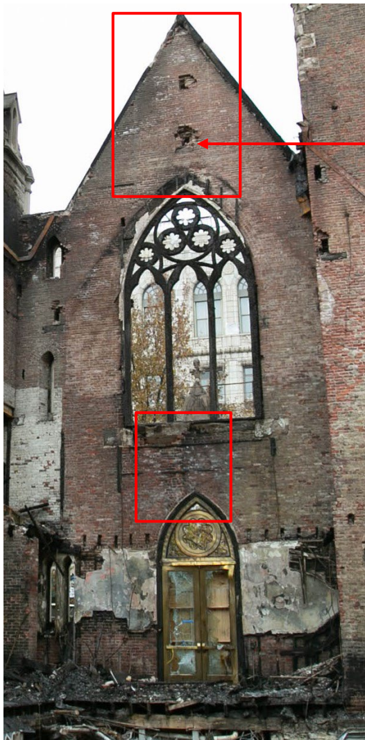
GABLE – BACK OF FACADE
