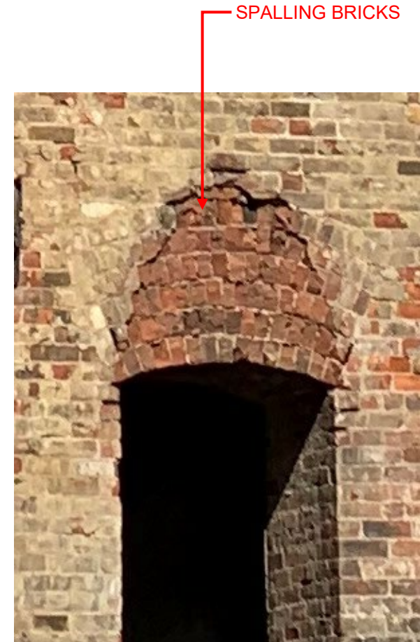
DETERIORATED MASONRY
