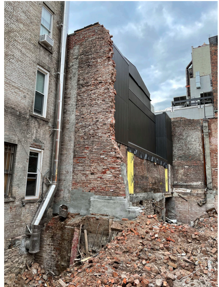
EAST WALL REMOVED PER DOB ORDER
