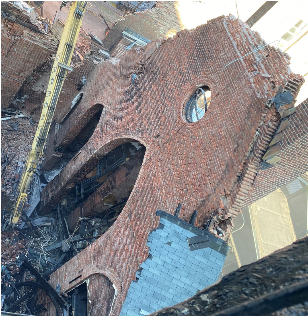
EAST WALL - POST FIRE
