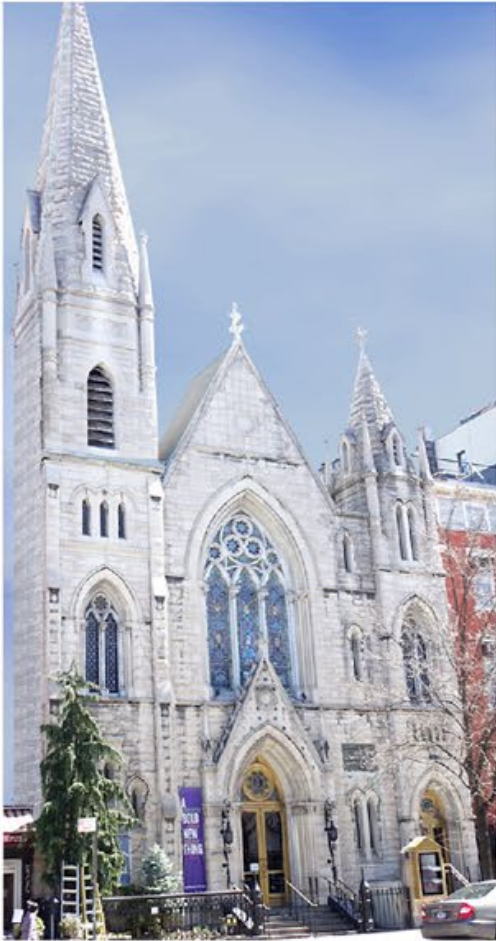
FACADE BEFORE FIRE
