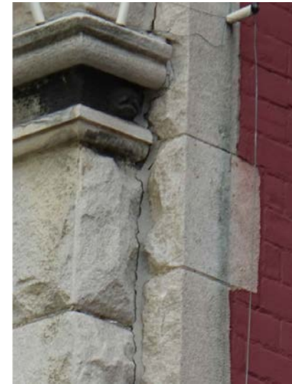
8. SOUTH TOWER – CRACK ENLARGED
