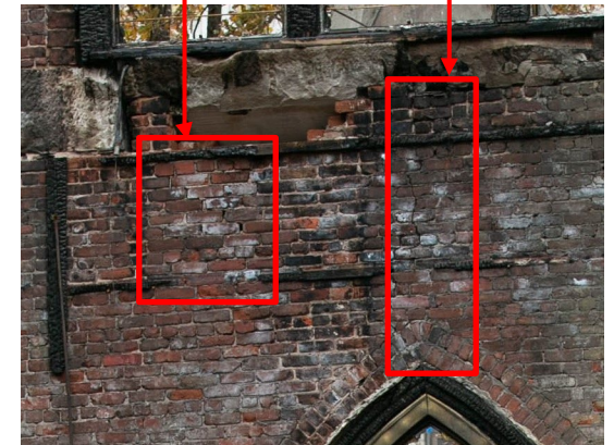
GABLE MASONRY CRACKS
