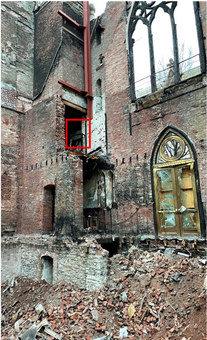
SOUTH TOWER BRACING
