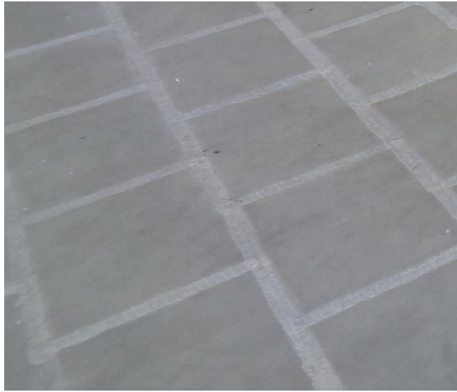
Flat seam metal roofing
