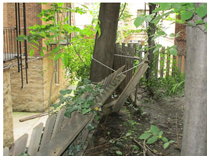
Collapsing fence at Hessian Hut area
