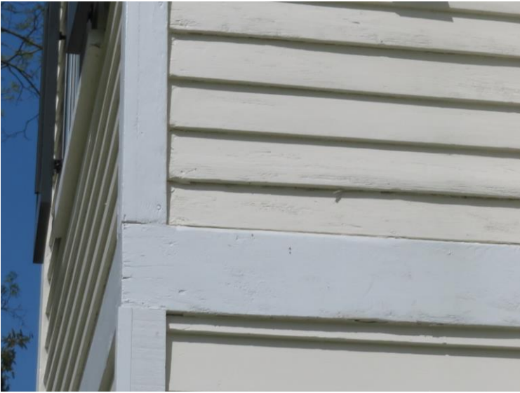
Wood siding and trim
