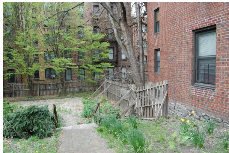
Deteriorated wood perimeter fence at northwest corner
