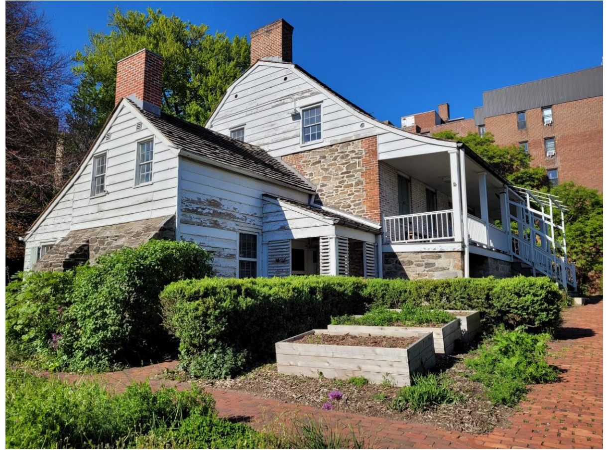
View from the southeast
