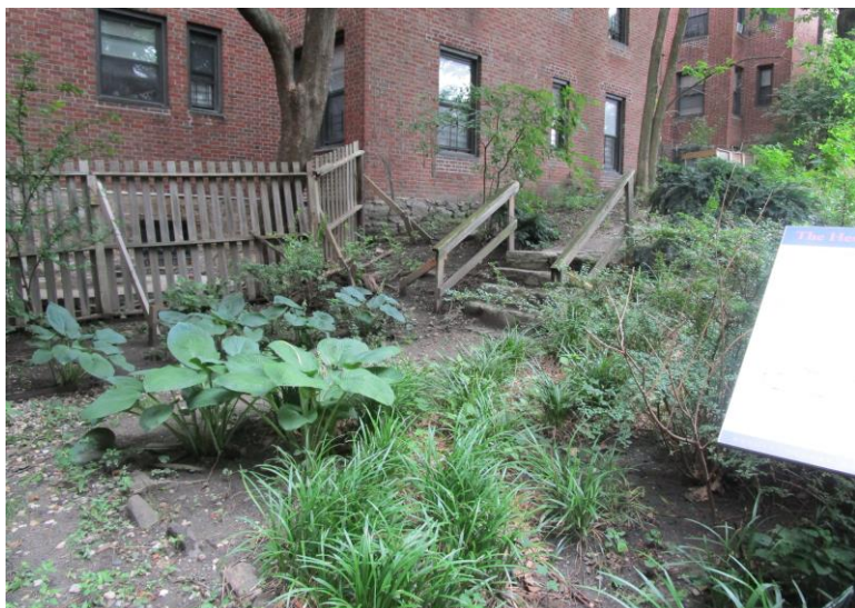
Deteriorated steps and railing at Hessian Hut
