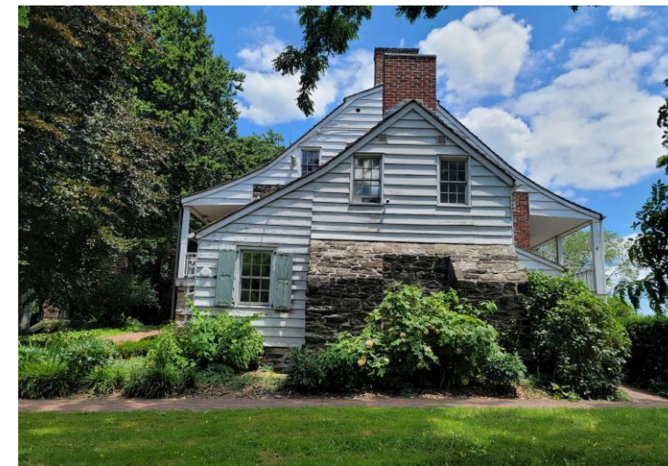
Overgrown plantings at the south side
