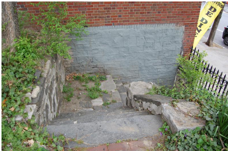
Abandoned north entrance on Broadway
