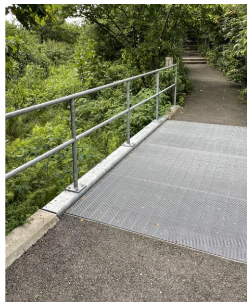
Grate Ramp Surface
