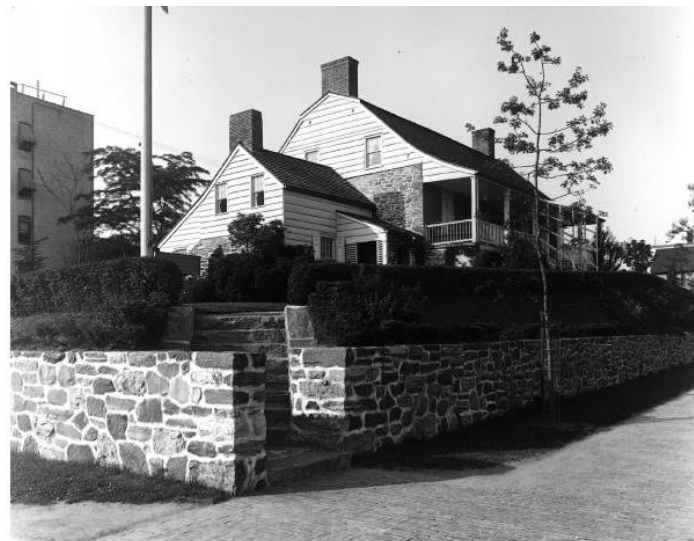
Southeast Corner from sidewalk
