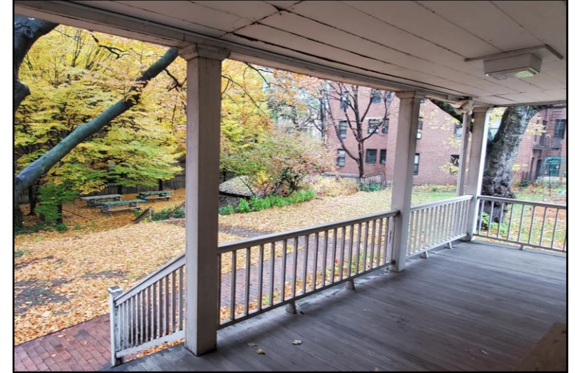
The Hessian Hut looking northwest from the west porch
