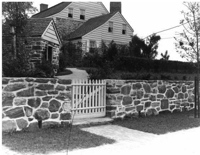
Southwest corner from sidewalk
