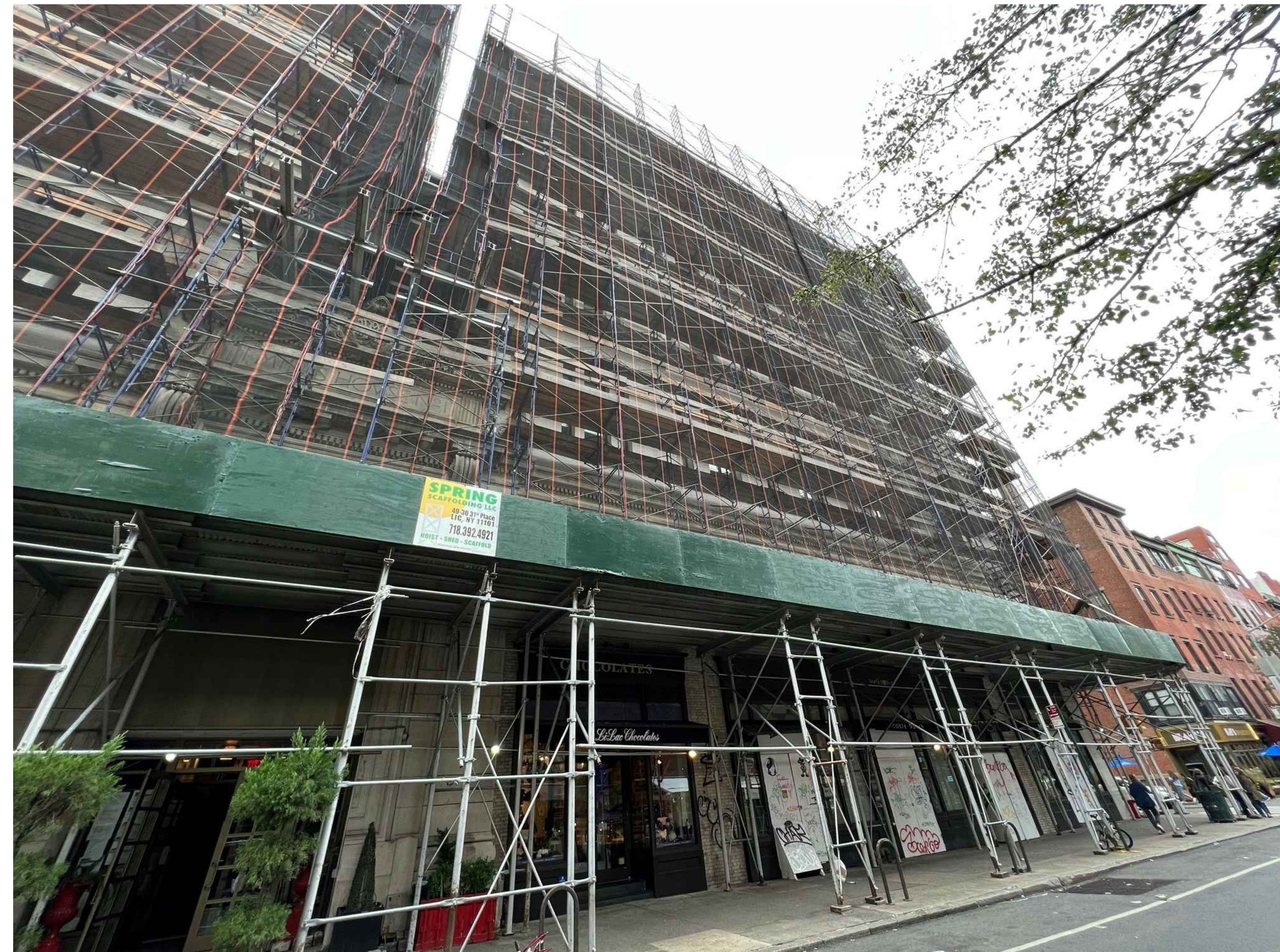
160 BLEECKER STREET LOOKING SOUTHWEST
