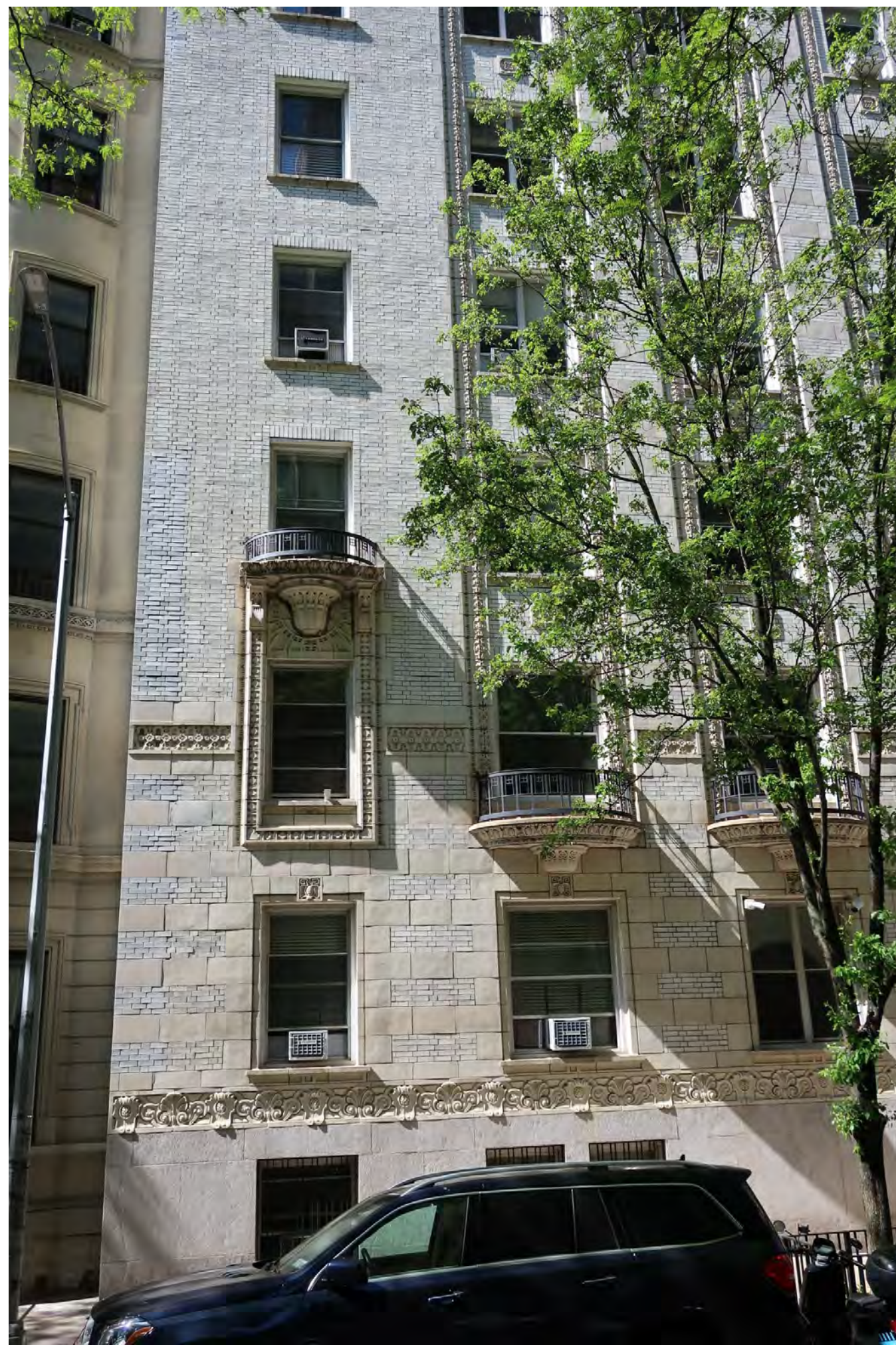
1. W. 98 STREET FACADE DETAIL
