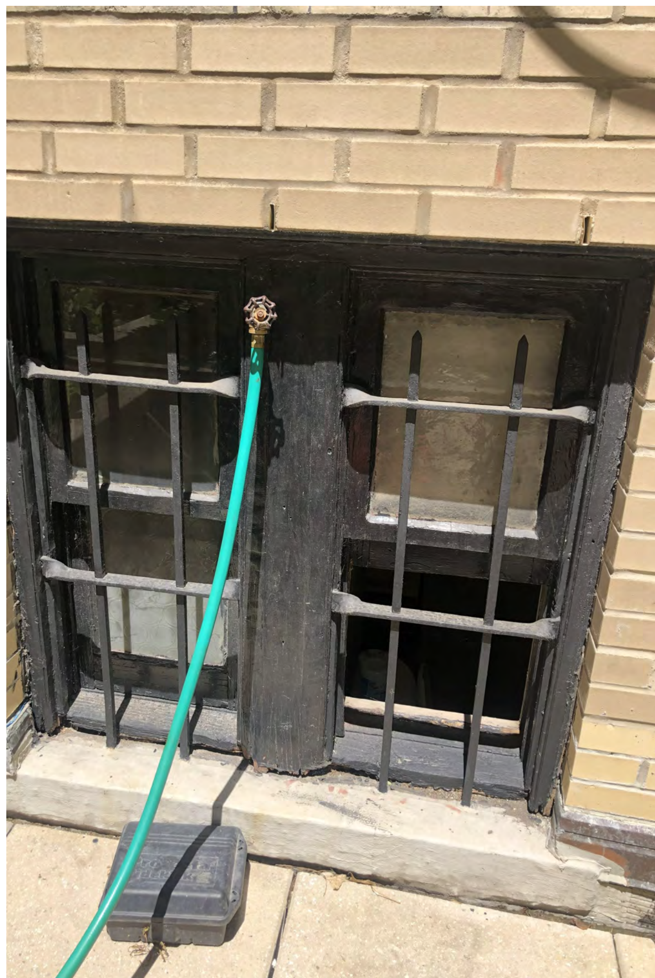
3. REMAINING WOOD WINDOW AR COURTYARD FACADE
