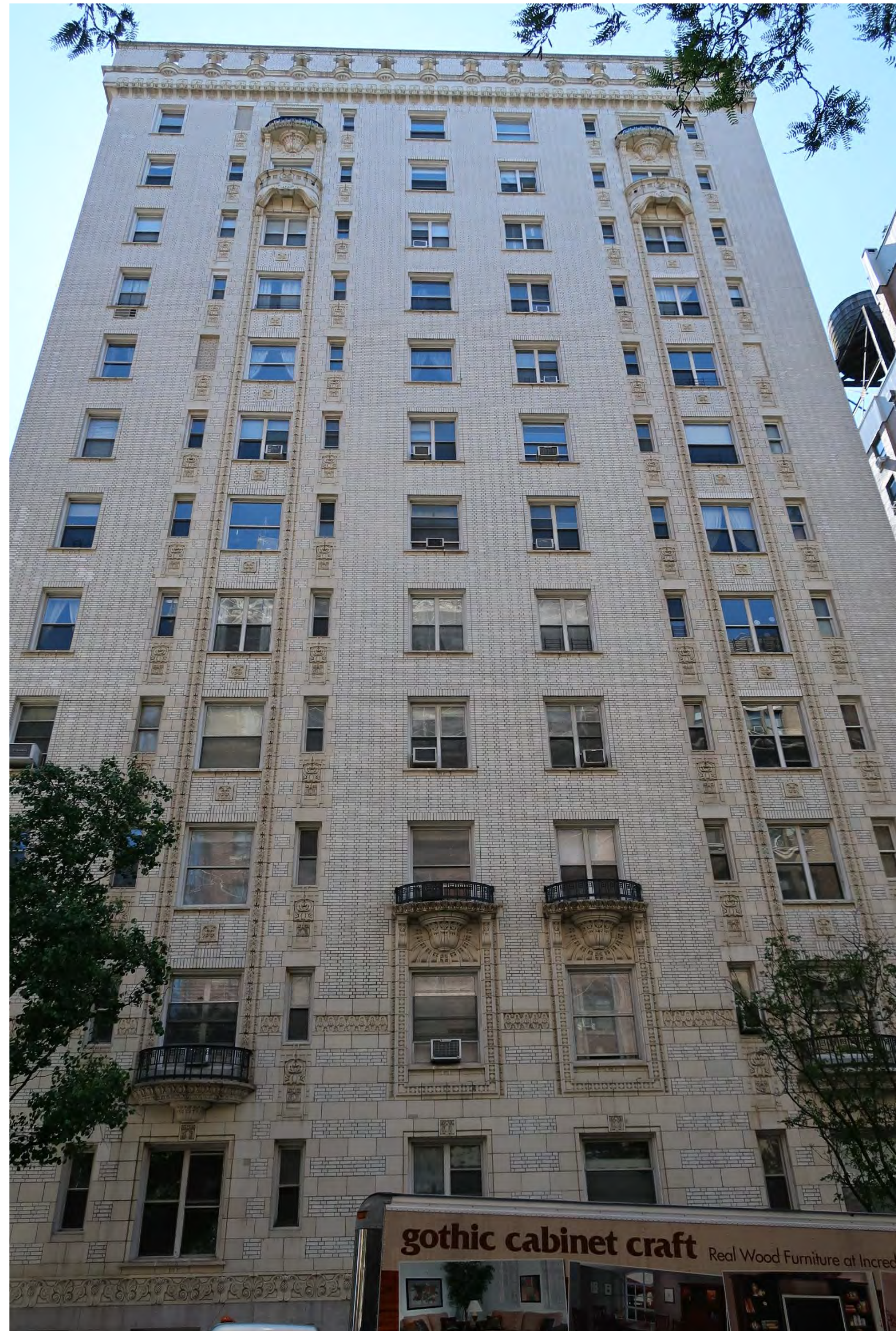
4. WEST END AVENUE FACADE
