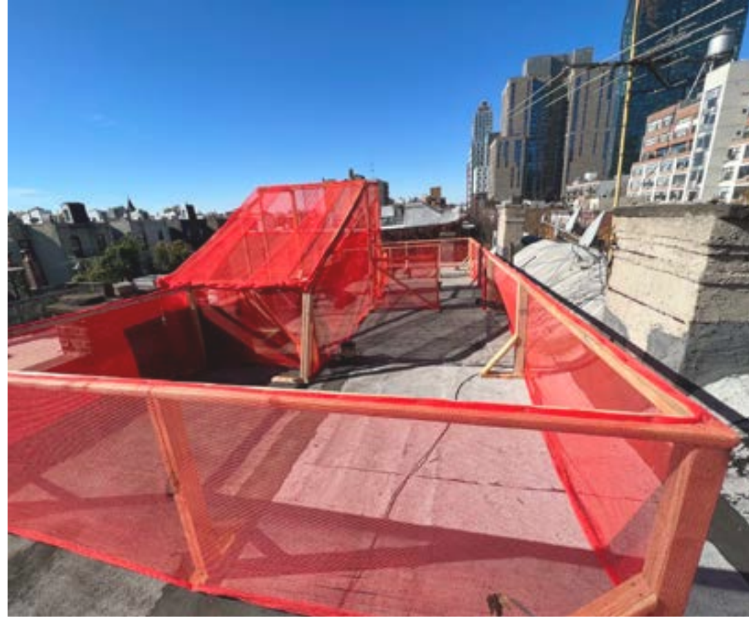
P2 - MOCKUP AT ROOF LOOKING W
