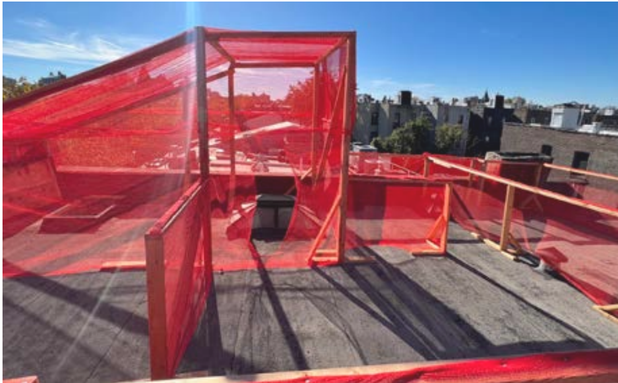
P3 - MOCKUP AT ROOF LOOKING NW
