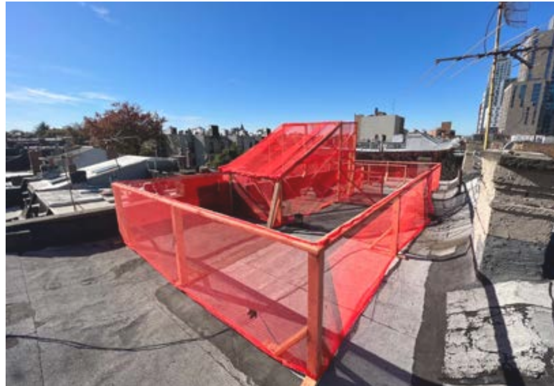
P4 - MOCKUP AT ROOF LOOKING S
