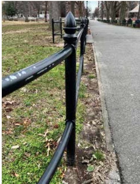
Pipe Rail Fence
