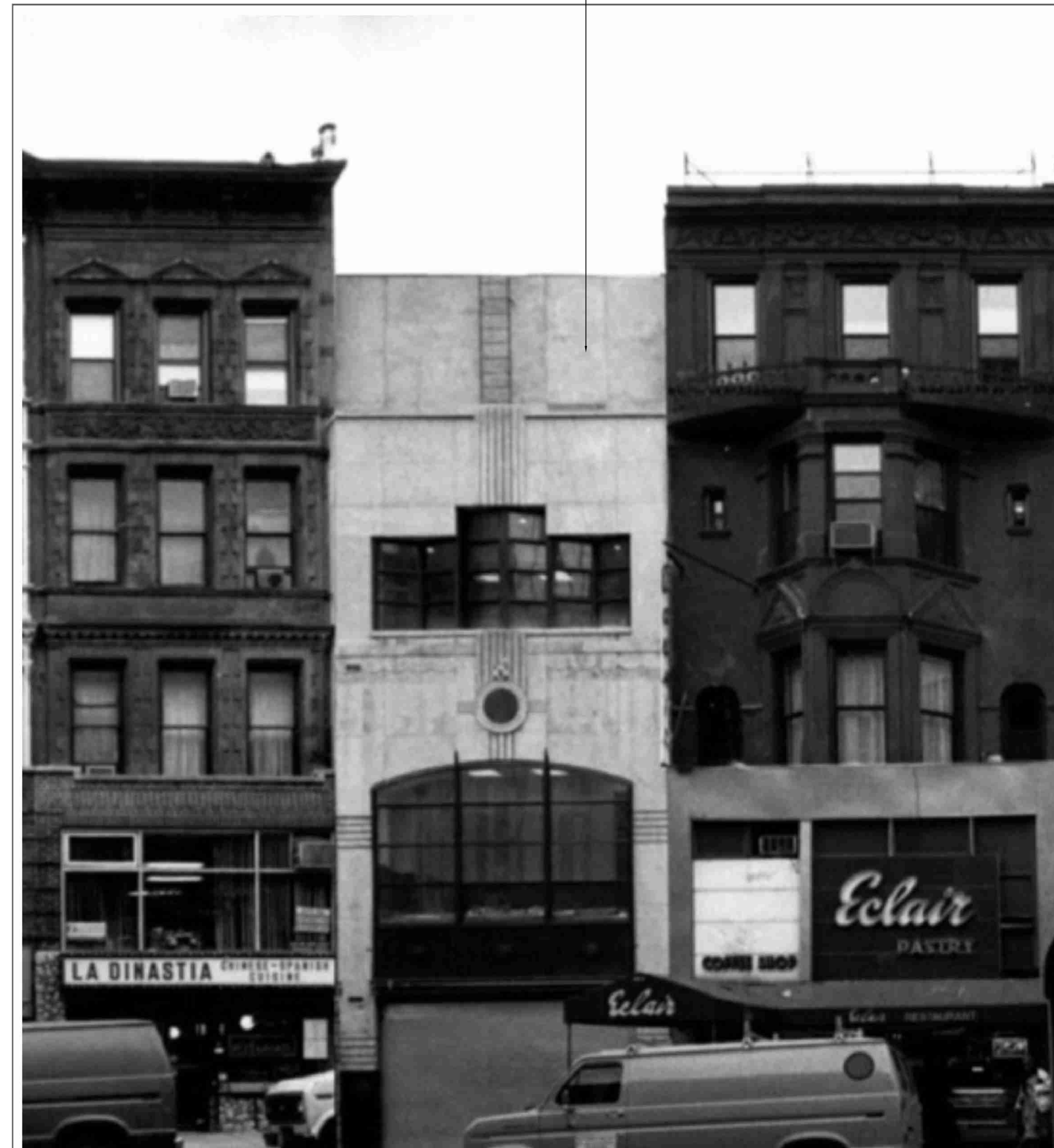
DESIGNATION PHOTO 1990 143 WEST 72 STREET
