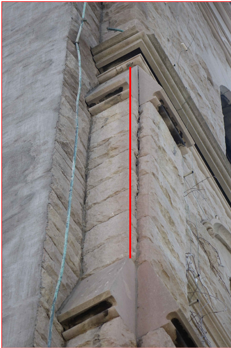
7. NORTH TOWER – EXTENT OF LIMESTONE CRACK
