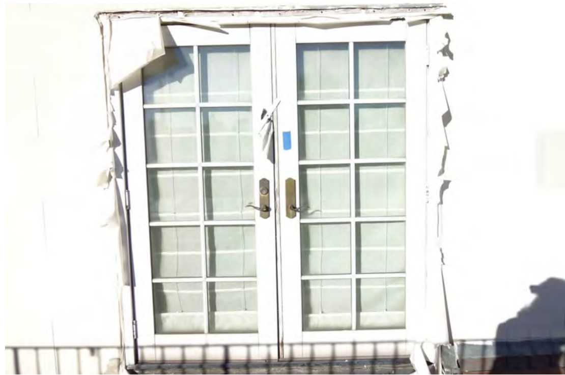
Typical Existing Door
