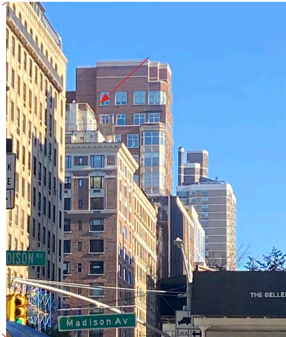
Limit of Visibility of Existing Chimney
