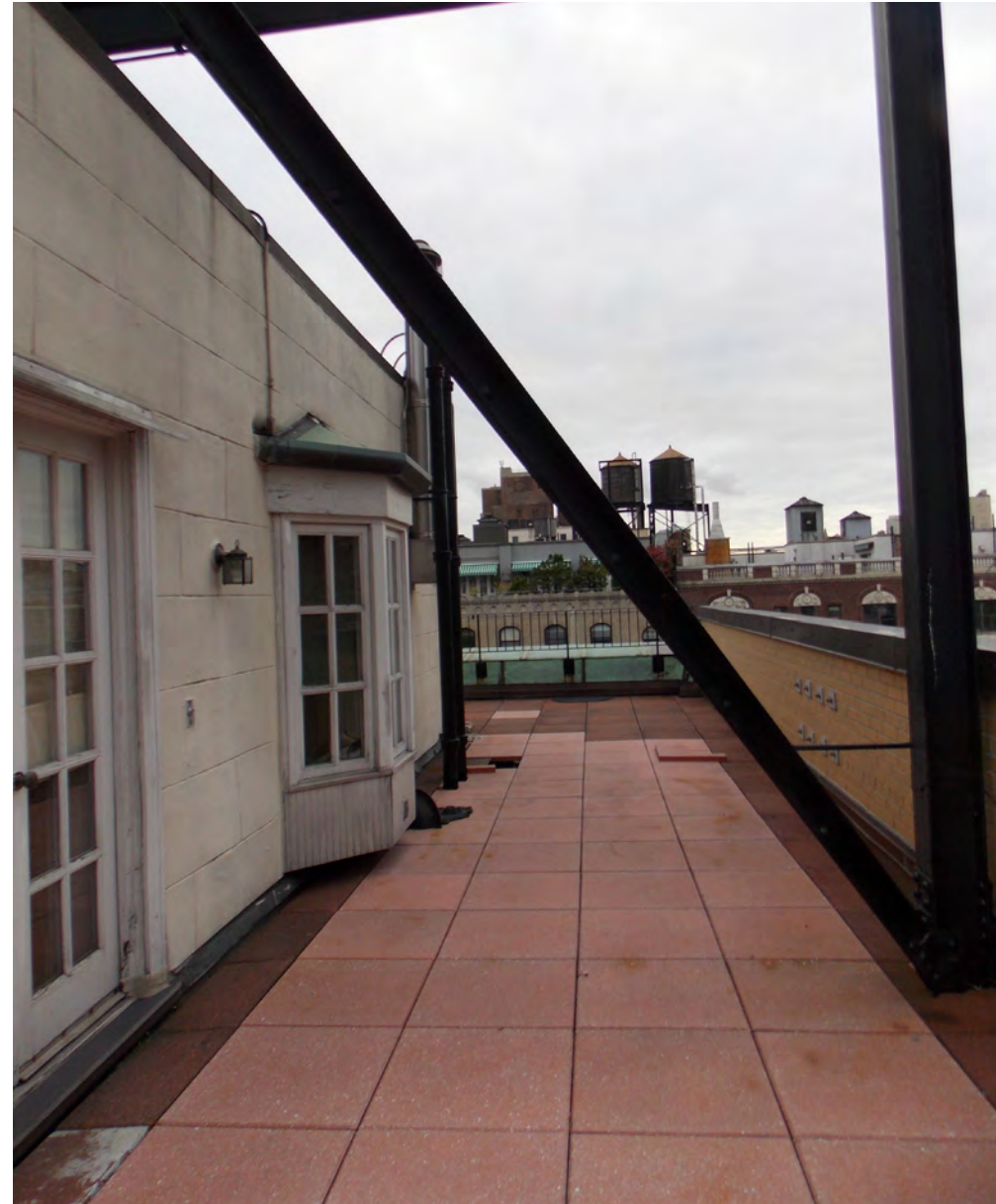
16th Floor North Terrace Looking West
