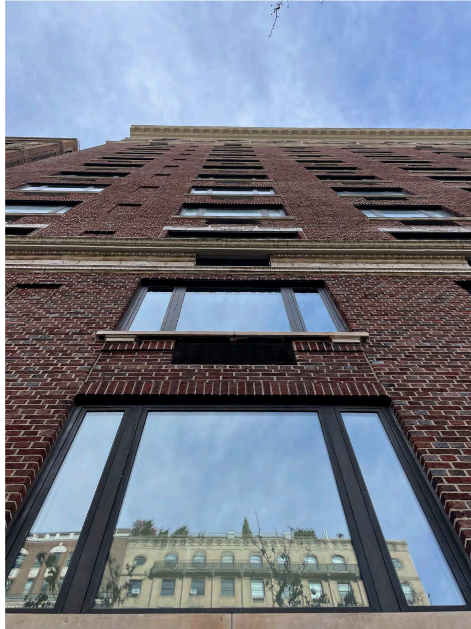
Existing Windows at Street Level
