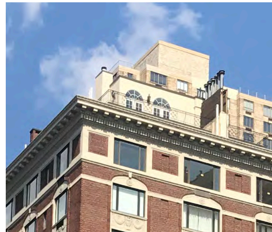
Existing View from South
