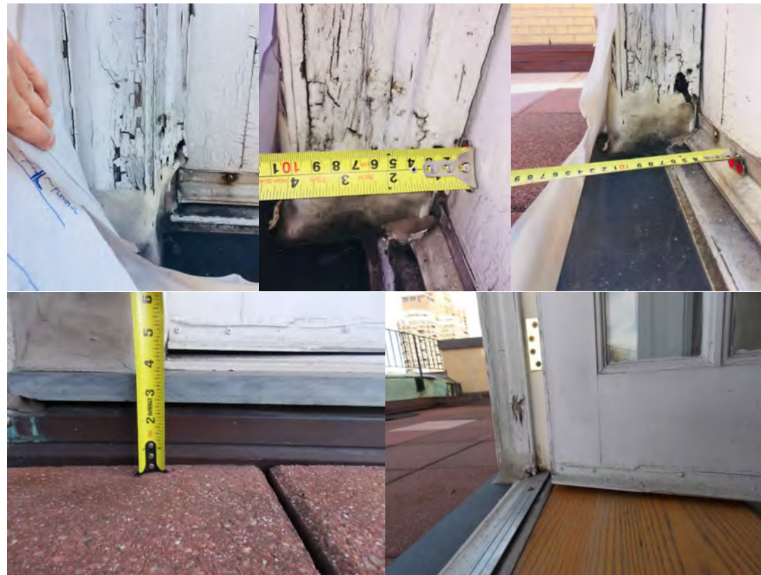
Existing Door Jamb and Sill Detail
