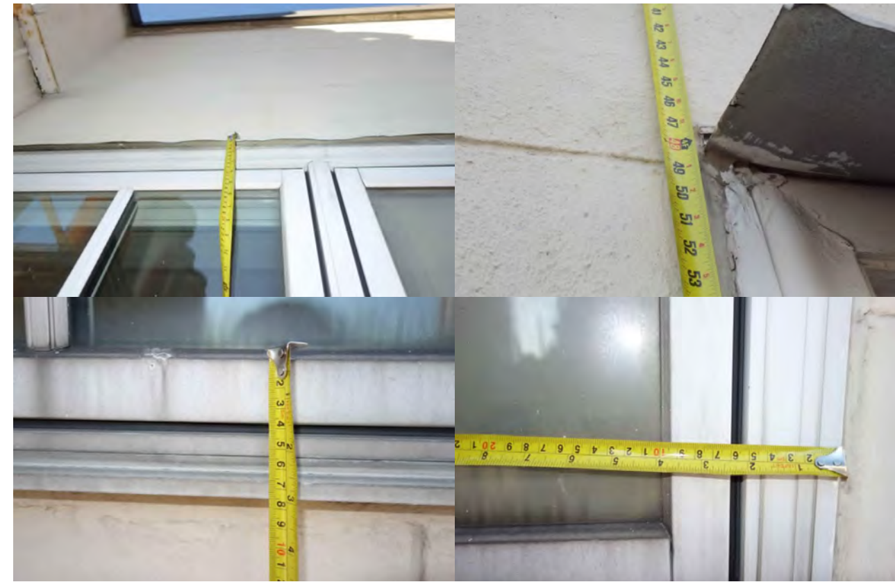
Existing Window Head and Jamb Detail
