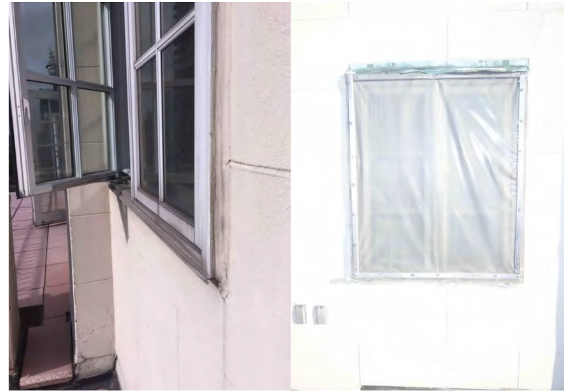
Typical Existing Window
