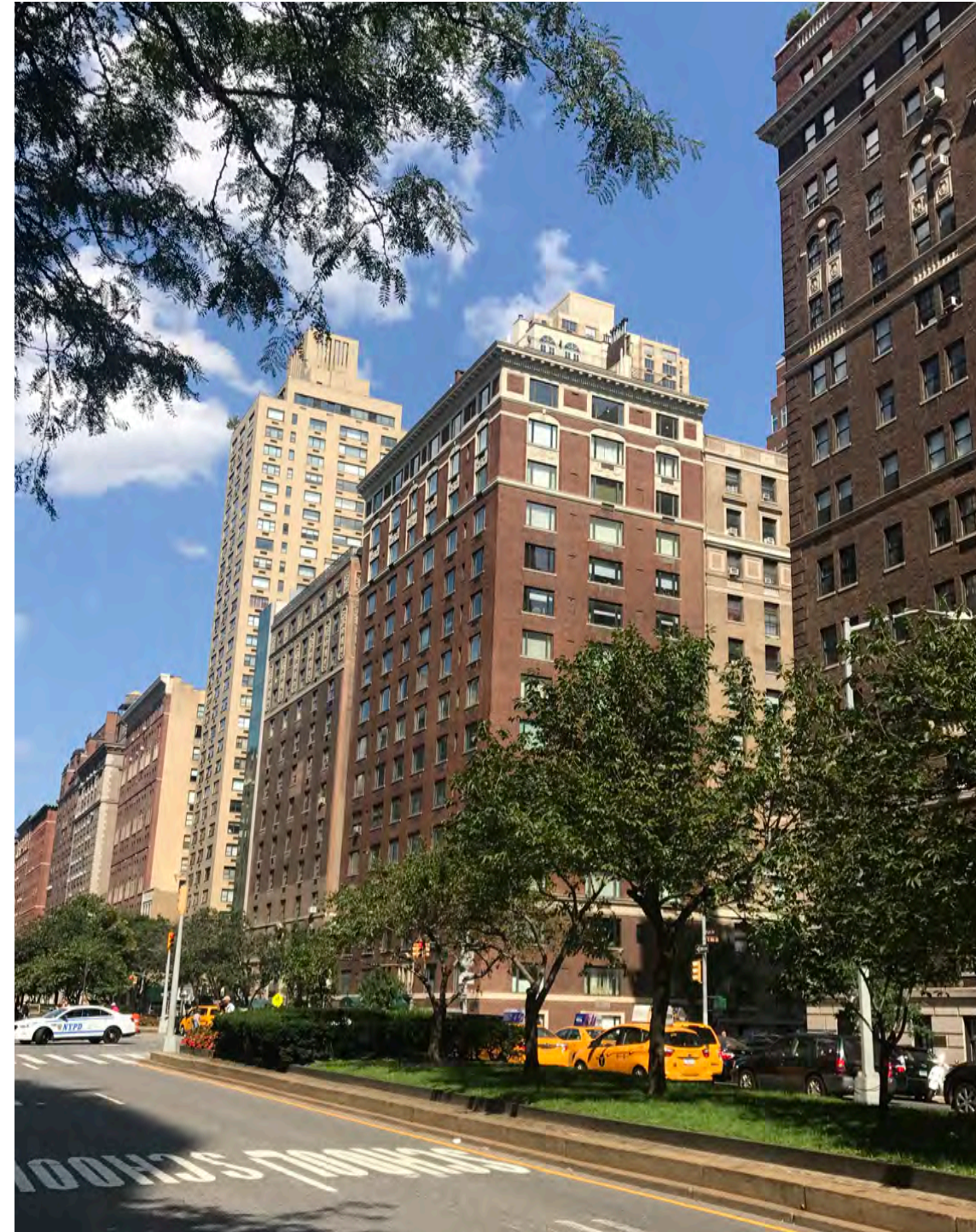
Park Avenue Between 86th and 85th Street Facing North
