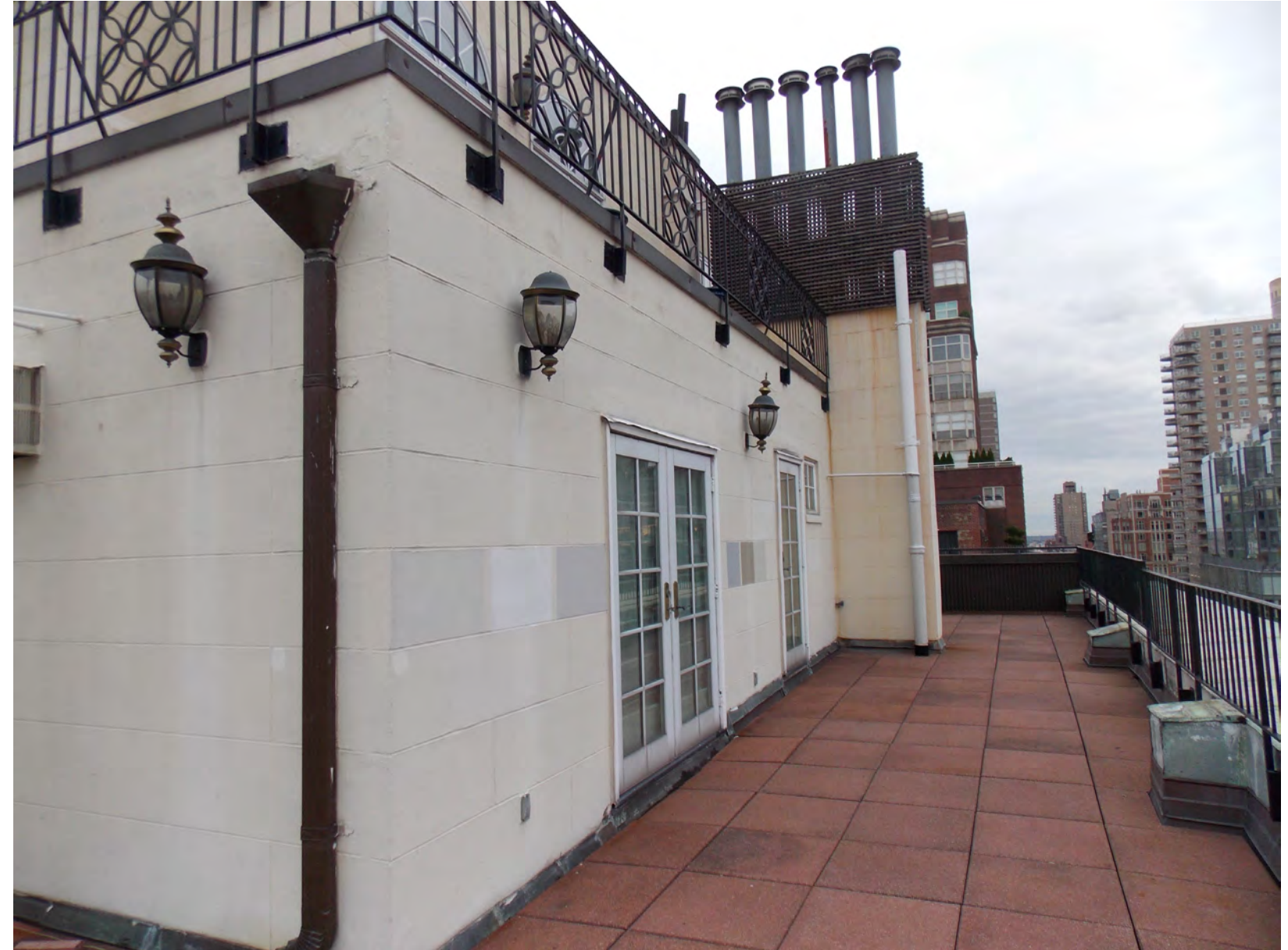
16th Floor South Terrace Looking East
