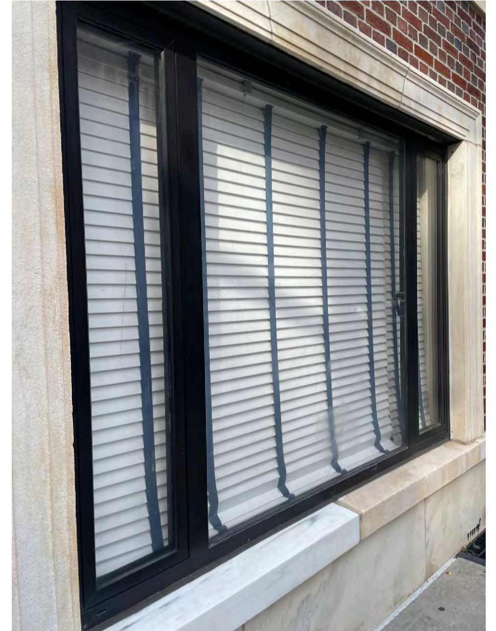
Existing Windows at Street Level
