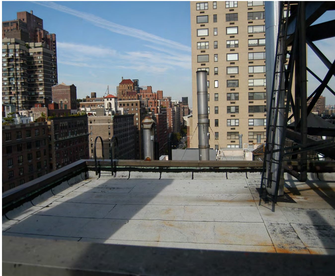
17th Floor North Terrace Looking North
