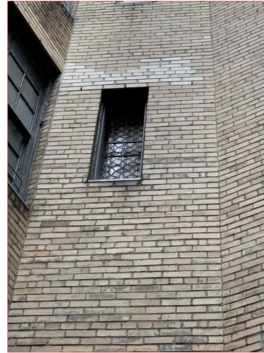
Steel casement interior insert which has leaded glass pattern Similar to steel casement inserts in the lobby
