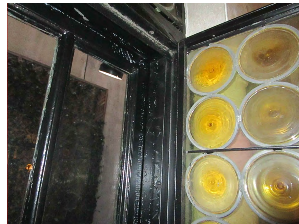
Interior photos of the lobby interior steel casement windows. This style matches the other areas where full height special glass has been installed.
