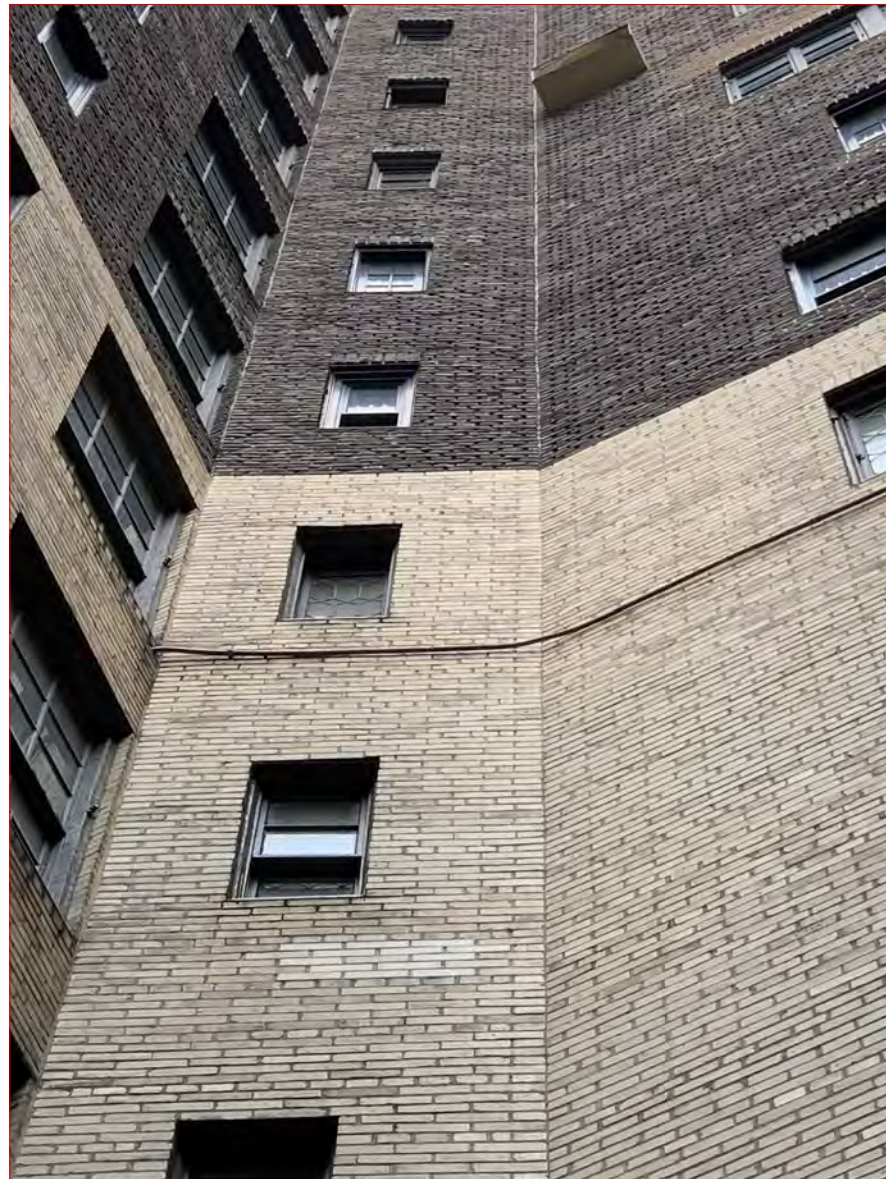
Steel casement interior insert which has leaded glass pattern on the 6th floor Similar to steel casement inserts in the lobby
