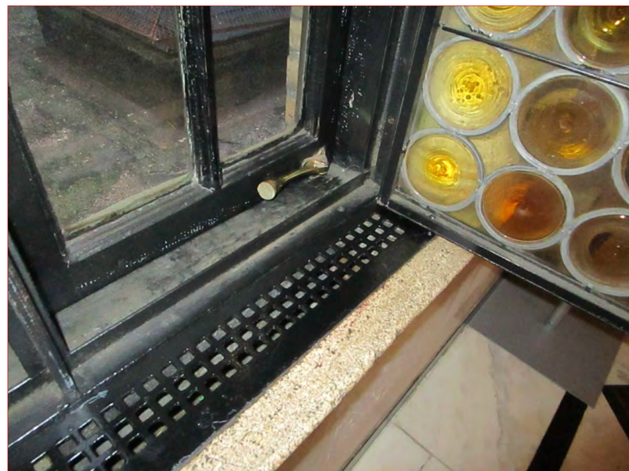
Interior photos of the lobby interior steel casement windows. This style matches the other areas where full height special glass has been installed.
