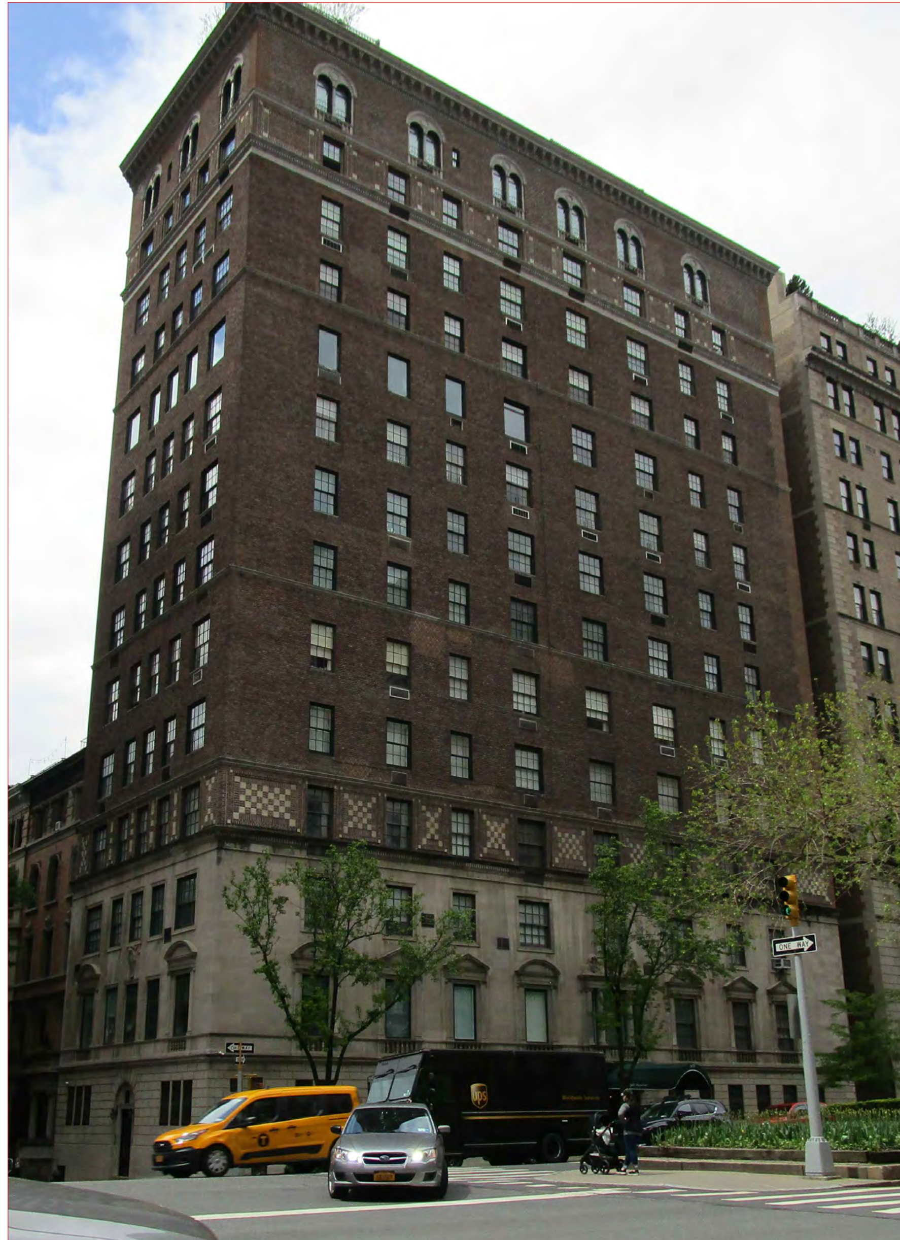
CURRENT BUILDING PHOTO
