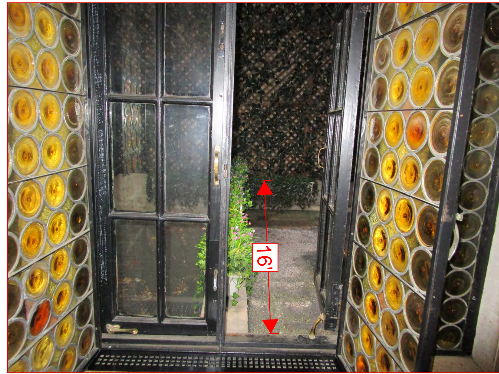
Existing Lobby to adjacent building wall
