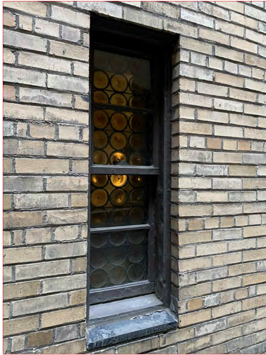
Historic double hung window with interior steel casement insert which has leaded glass pattern
