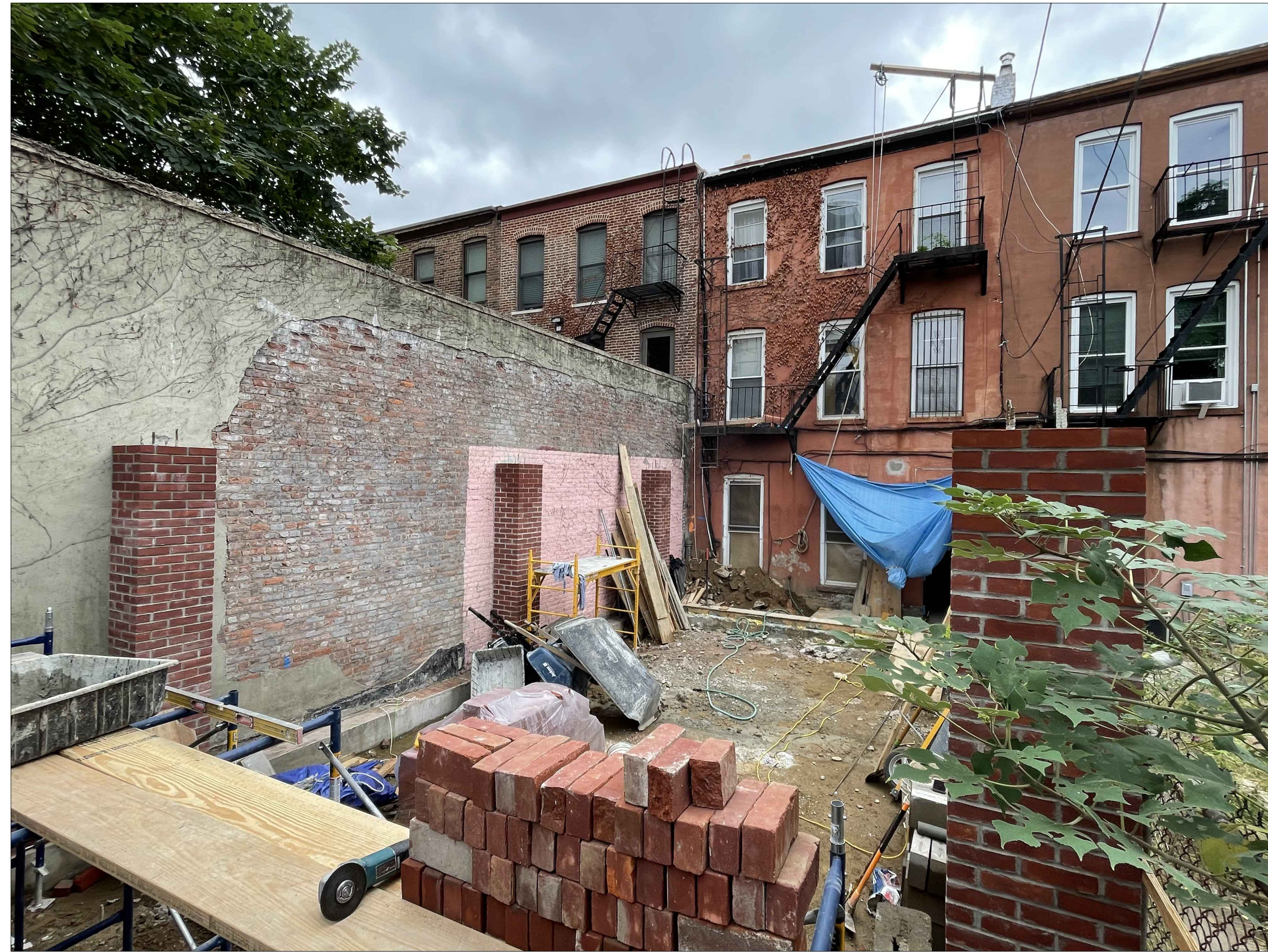
EXISTING REAR YARD (LOOKING WEST)
