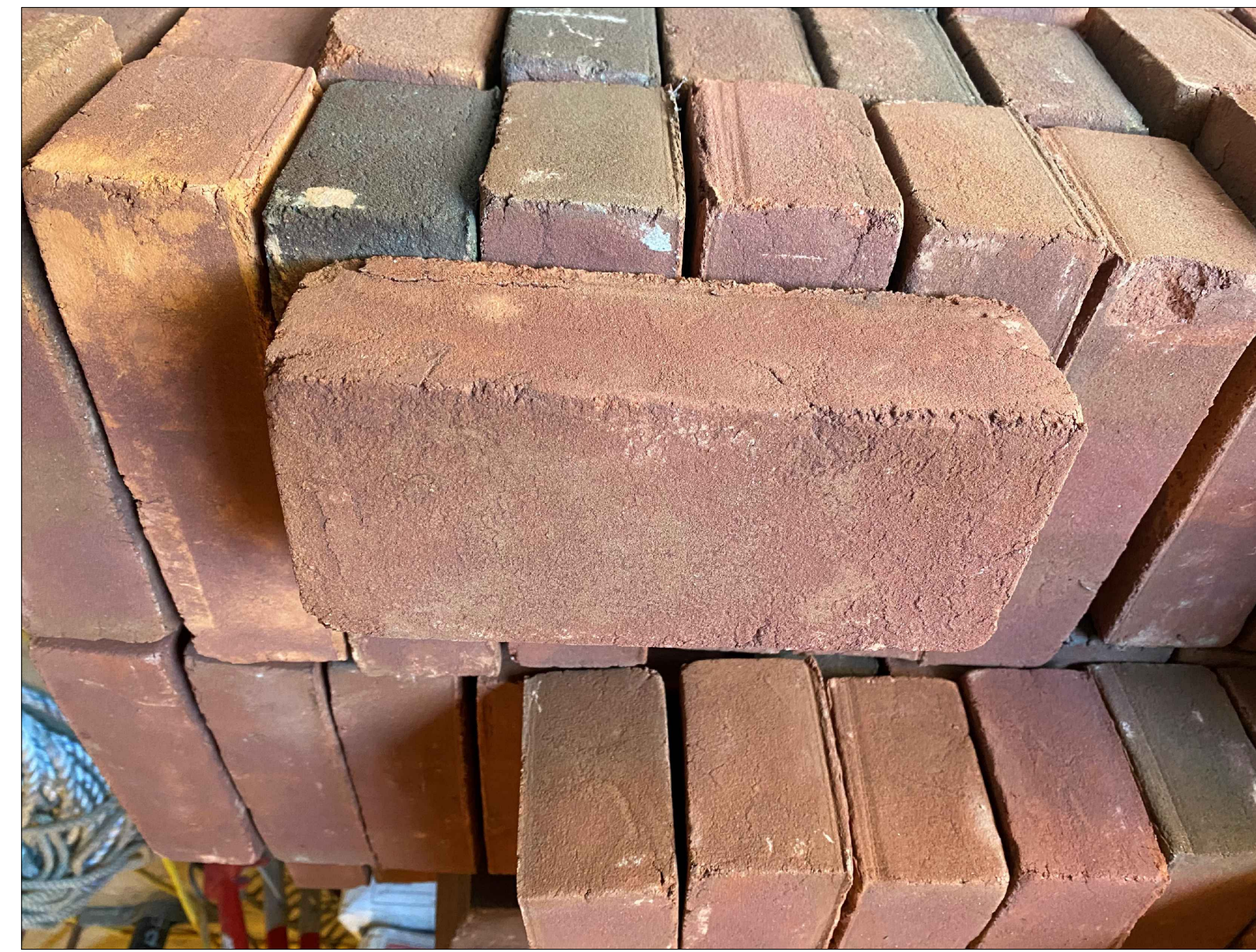
BRICK WALLS & COLUMNS (REAR YARD)
