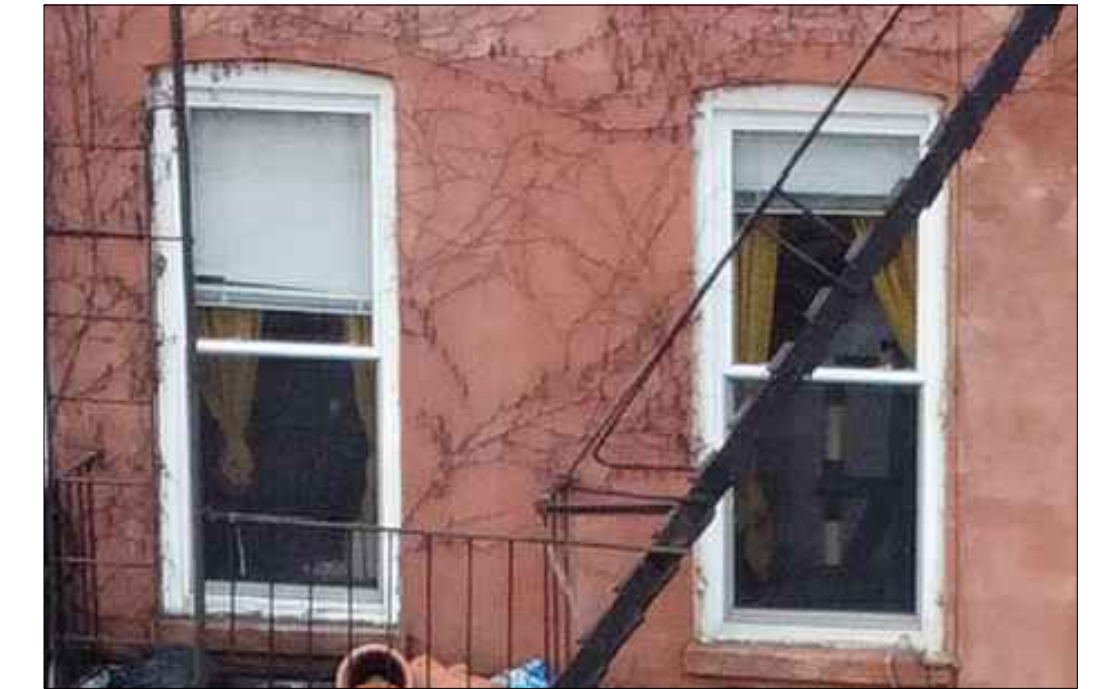
1/2" STUCCO WALL TO MATCH EXISTING BUILDING FACADE
