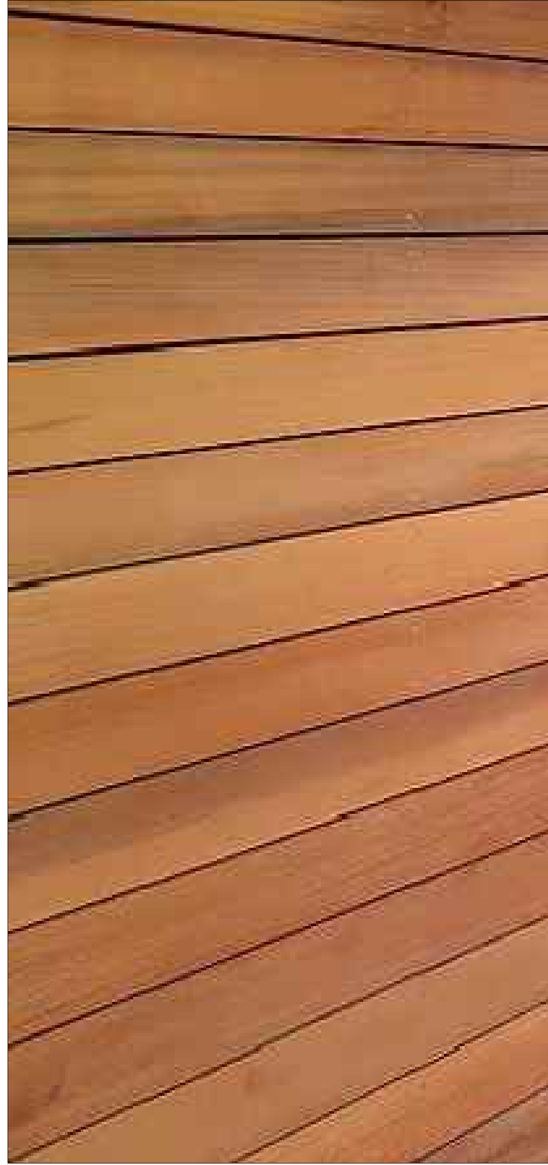
REAR YARD INTERIOR WALLS
