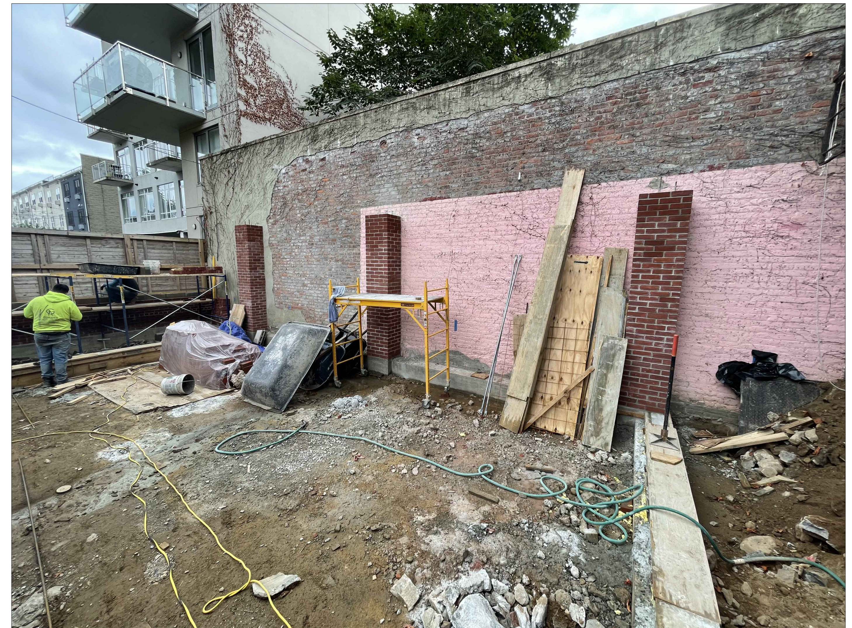
EXISTING REAR YARD (LOOKING EAST)
