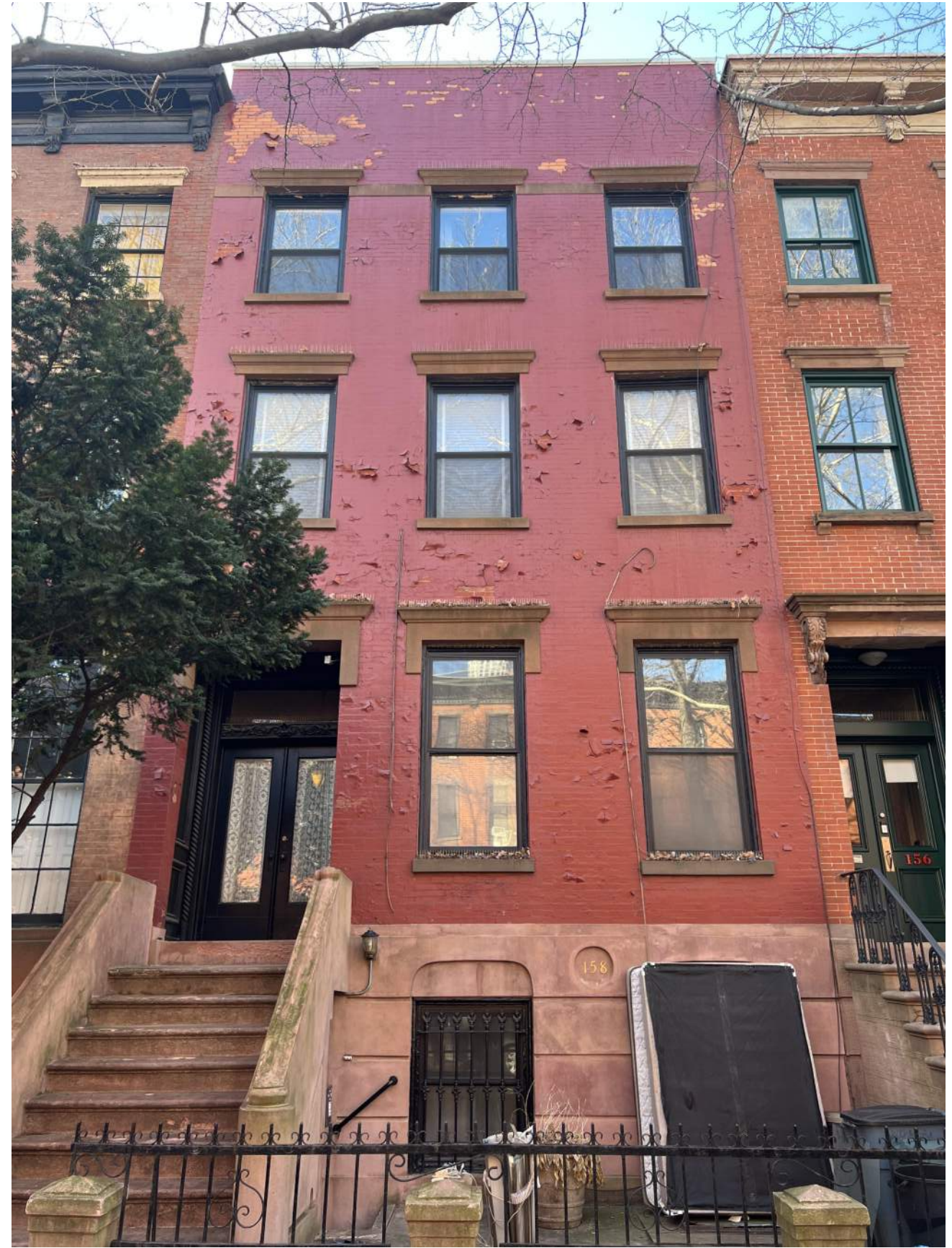
158 BERGEN STREET - EXISTING FRONT FACADE (2/10/2022)
