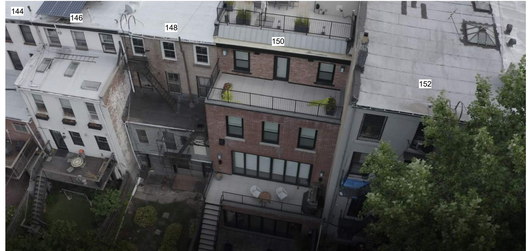
AERIAL PHOTO - 144, 146, 148, 150 & 152 BERGEN STREET
