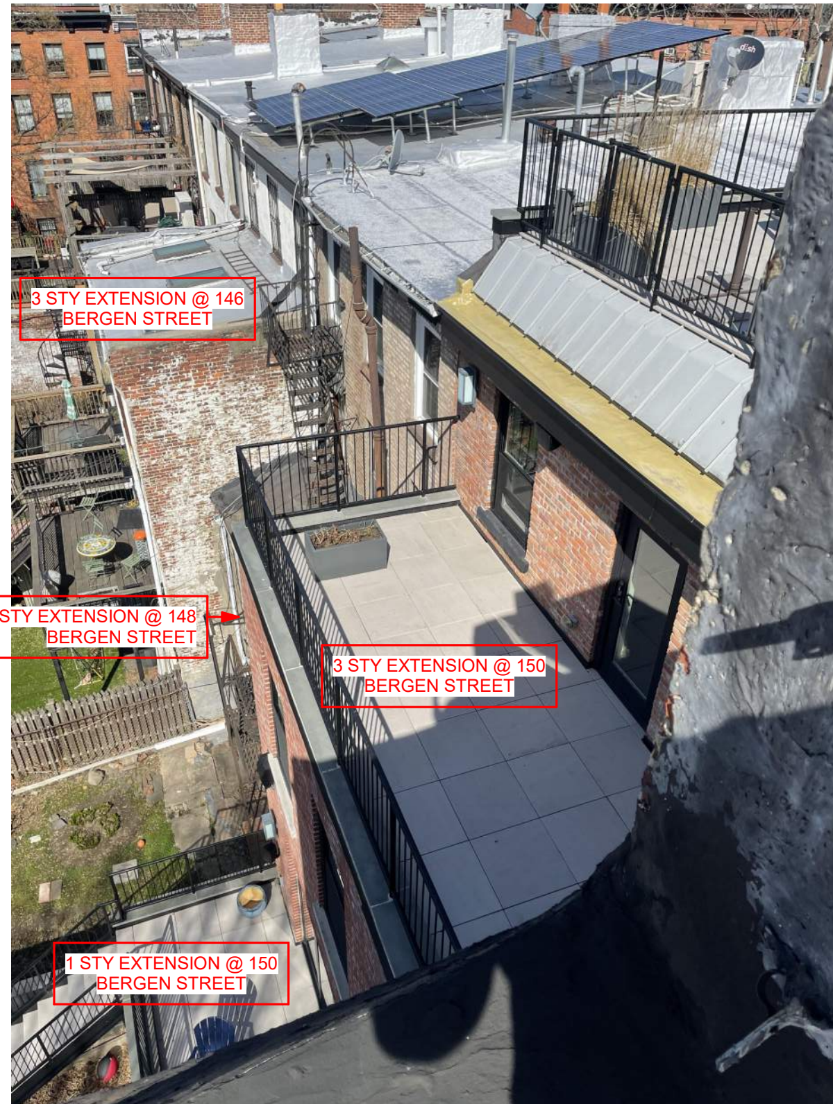
PRECEDENT PHOTO - EXISTING REAR FACADE OF 146, 148 & 150 BERGEN STREET
