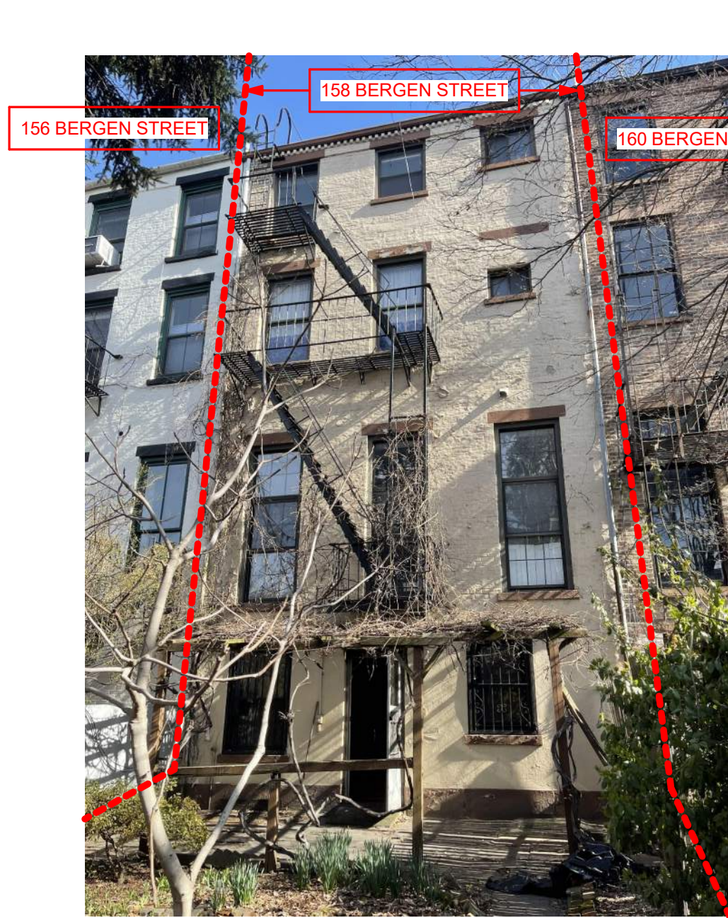
EXISTING REAR FACADE OF 158 BERGEN STREET
