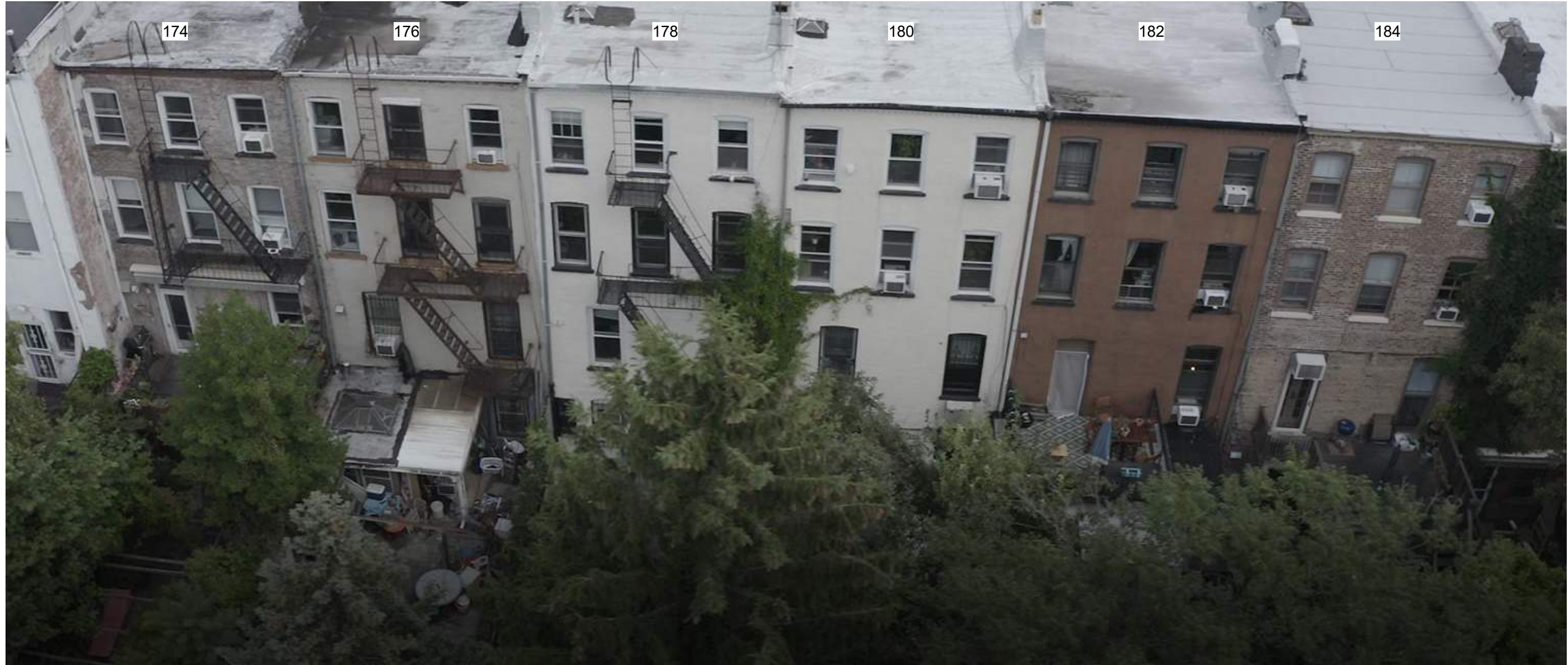
AERIAL PHOTO - 160, 162, 164, 166, 168, 170 & 172 BERGEN STREET
