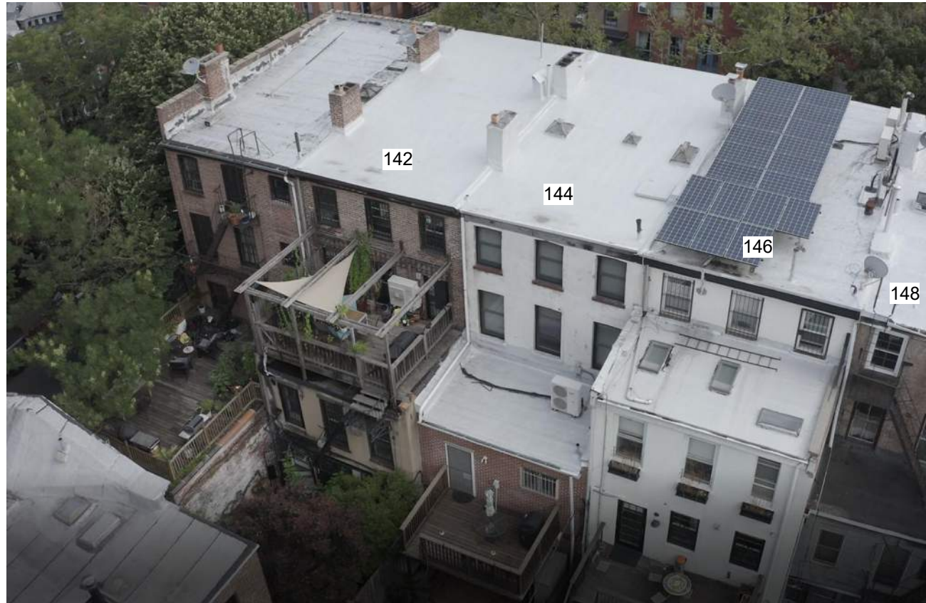
AERIAL PHOTO - 142, 144, 146 & 148 BERGEN STREET
