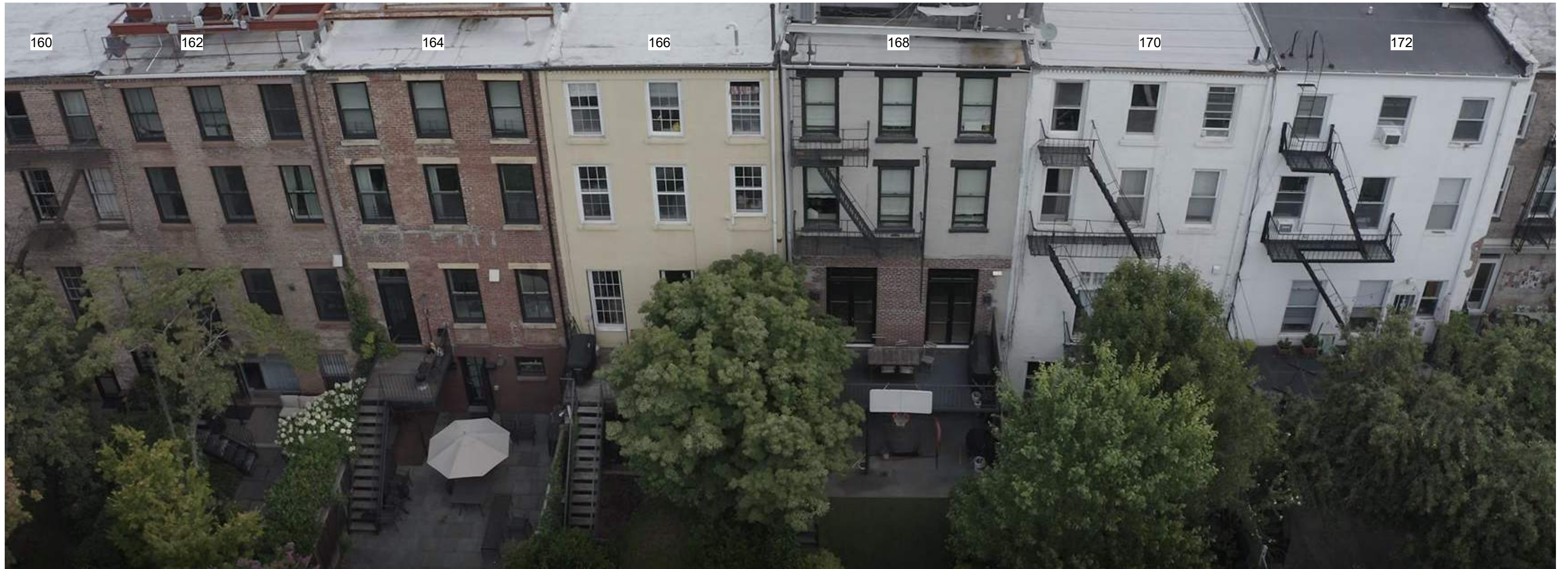
AERIAL PHOTO - 160, 162, 164, 166, 168, 170 & 172 BERGEN STREET
