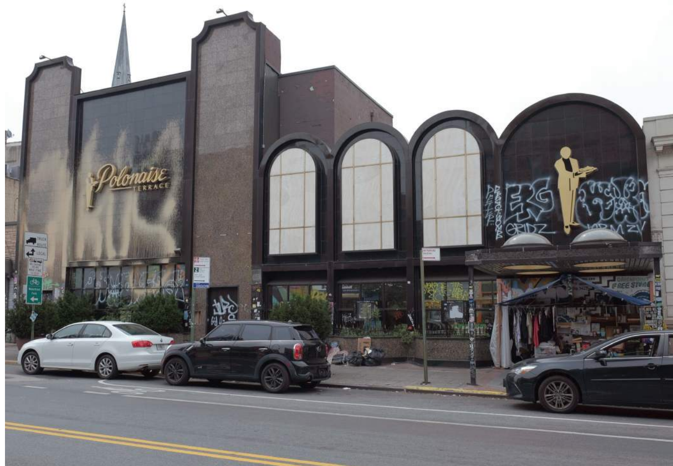
2021 PHOTO OF EXISTING BUILDING
