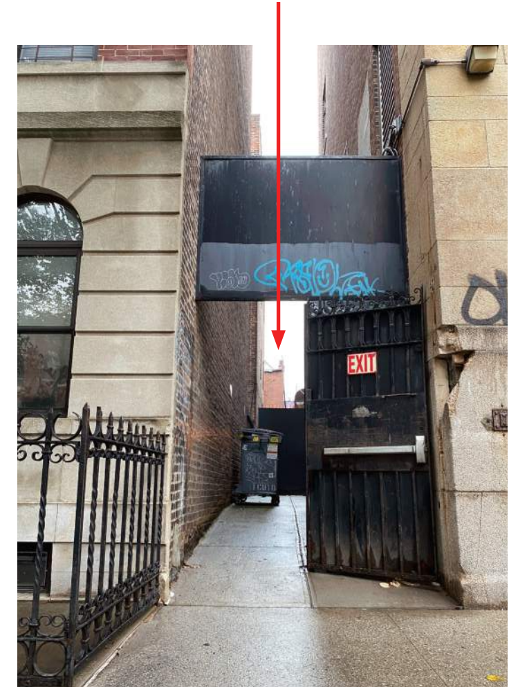
VIEW LOOKING DOWN ALLEYWAY AT 163 MILTON FROM NORTH SIDE OF MILTON STREET.
