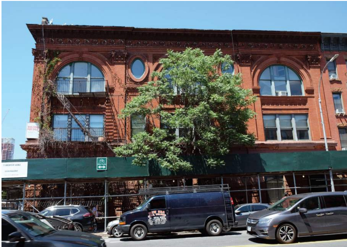
144 FRANKLIN ST, SOUTH VIEW
