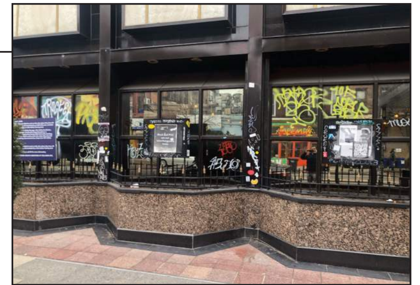
EXISTING PLANTERS AT ONE STORY PORTION
