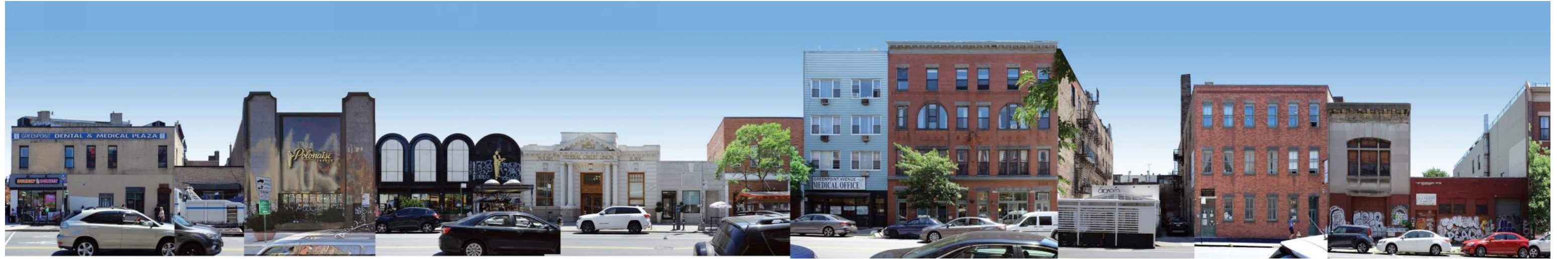
GREENPOINT AVENUE ELEVATION LOOKING SOUTH - EXISTING
