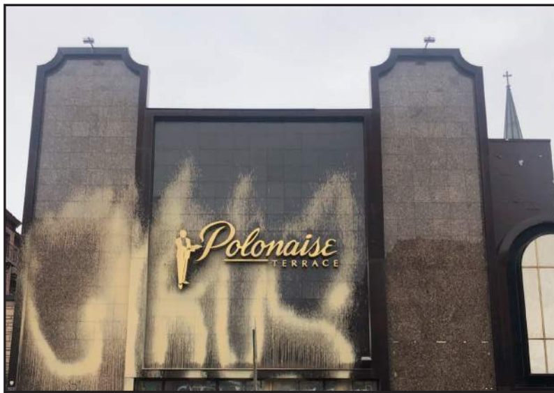
EXISTING FACADE AT TWO STORY PORTION
