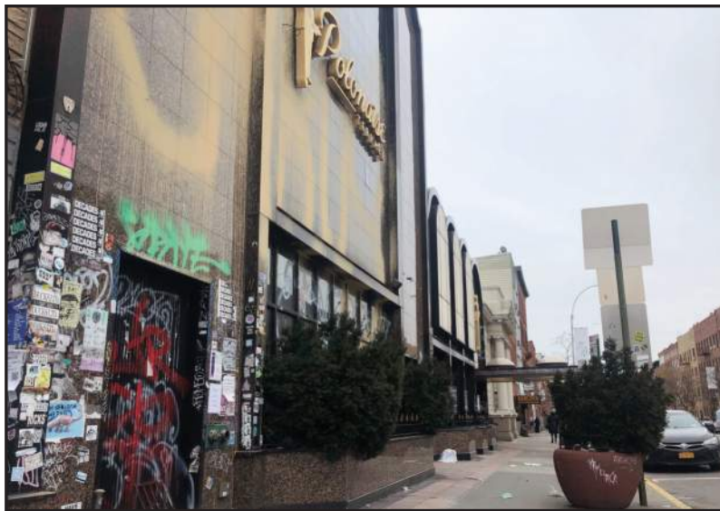
EXISTING ENTRY AT TWO STORY PORTION
