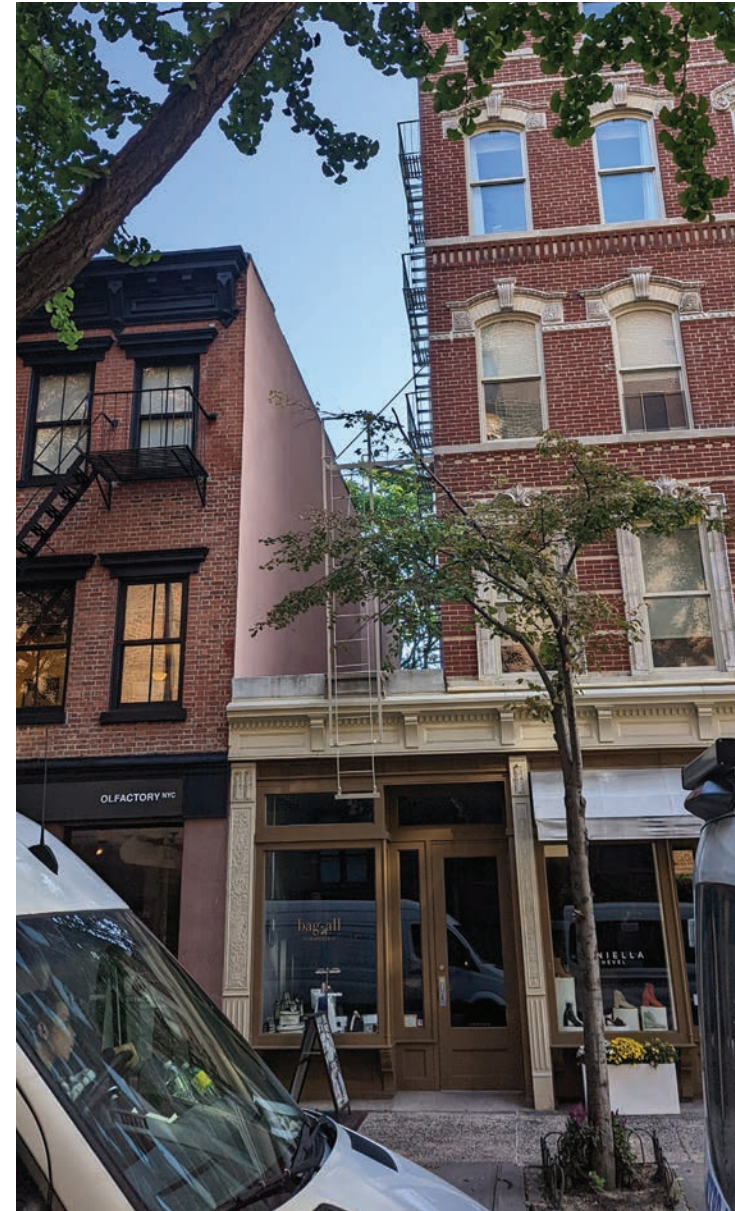
06. THROUGH VIEW FROM 355 BLEECKER STREET
