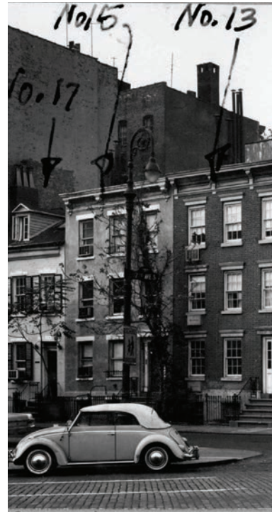
15 Commerce Street at designation District: Greenwich Village Built: 1826. Finish: White smooth coat stucco over brick
