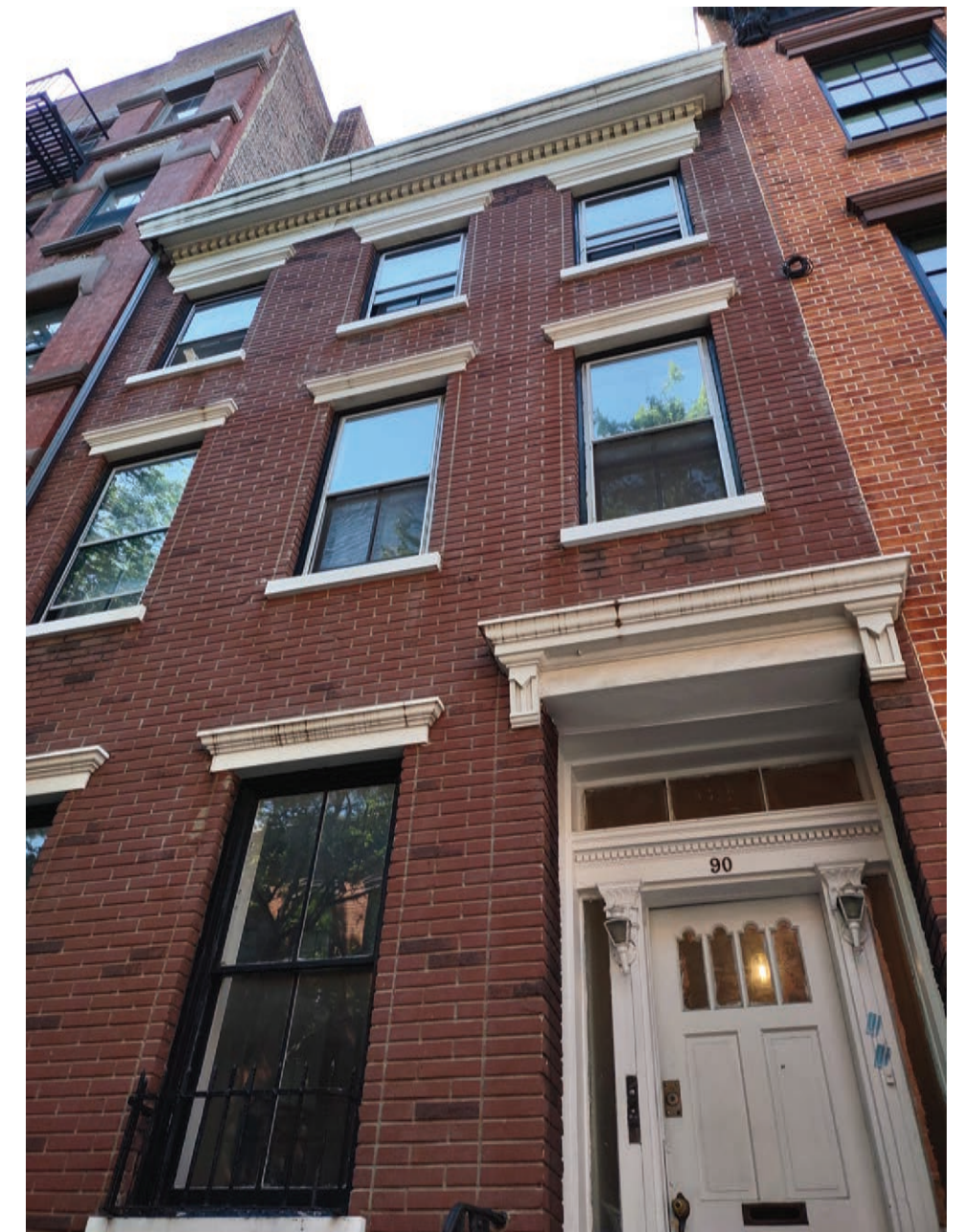
EXISTING FRONT FAÇADE PHOTO
