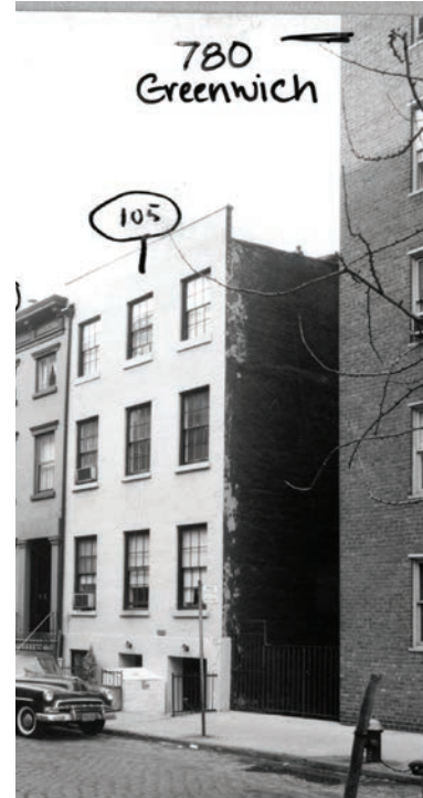
105 Bank Street at designation District: Greenwich Village Built: 1846. Finish: White smooth coat stucco over brick
