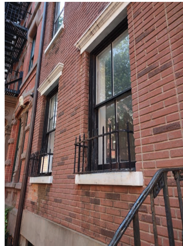
EXISTING FRONT FAÇADE PHOTO
