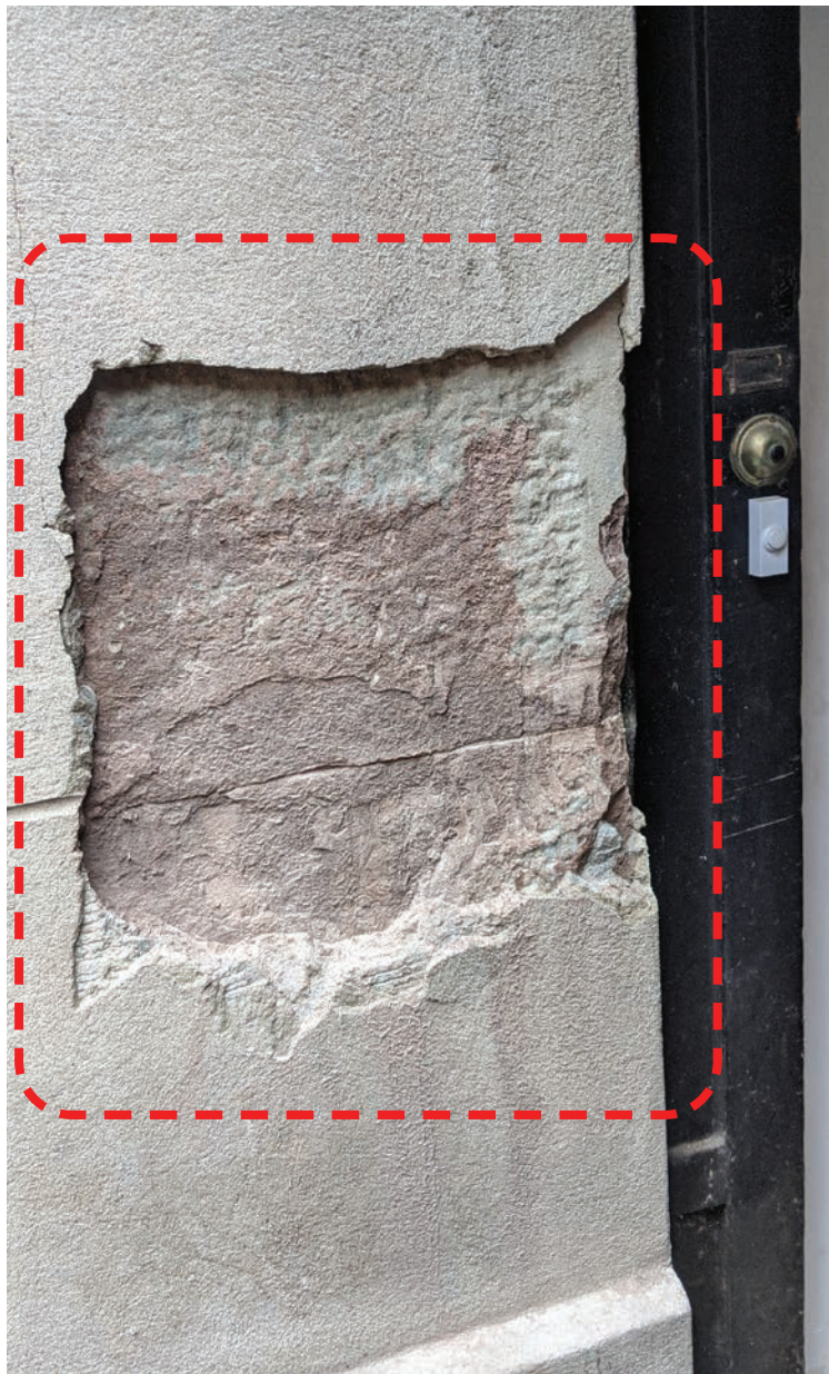
FRONT FACADE BROWNSTONE PROBE
