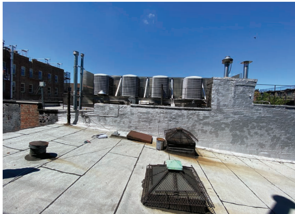
02. EXISTING ROOF TOP LOOKING WEST
