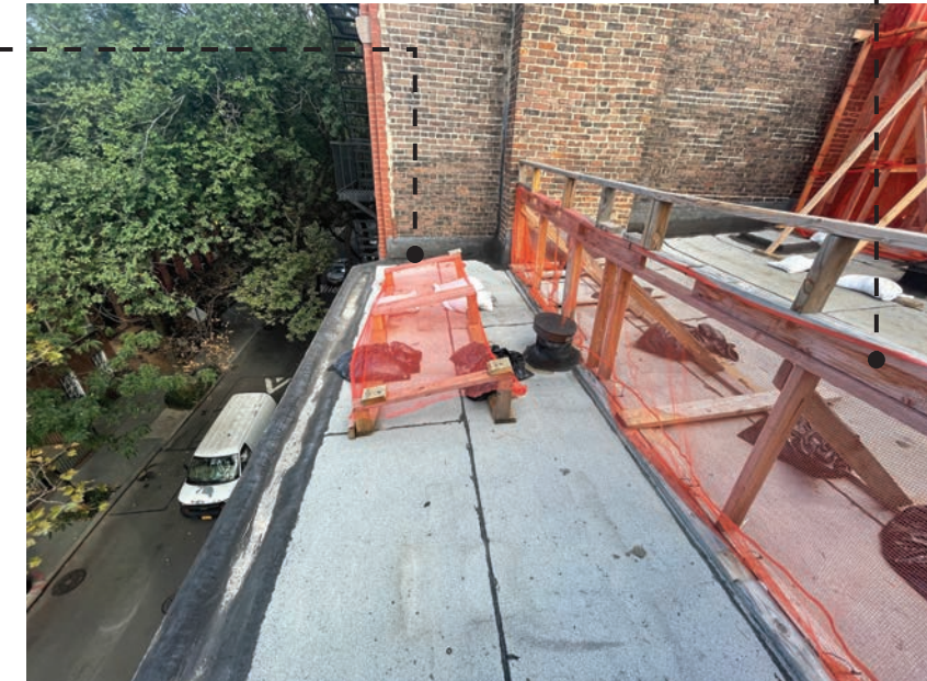
3RD FLOOR SKYLIGHT AND GUARD RAILING MOCK-UP
