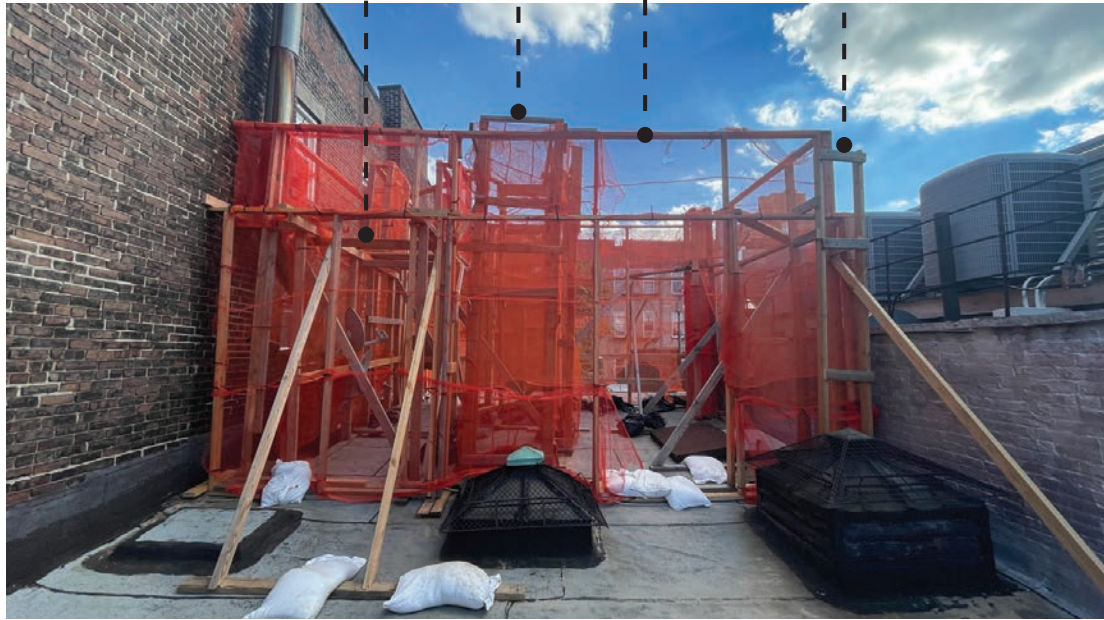
ROOFTOP ADDITION MOCK-UP FROM NORTH
