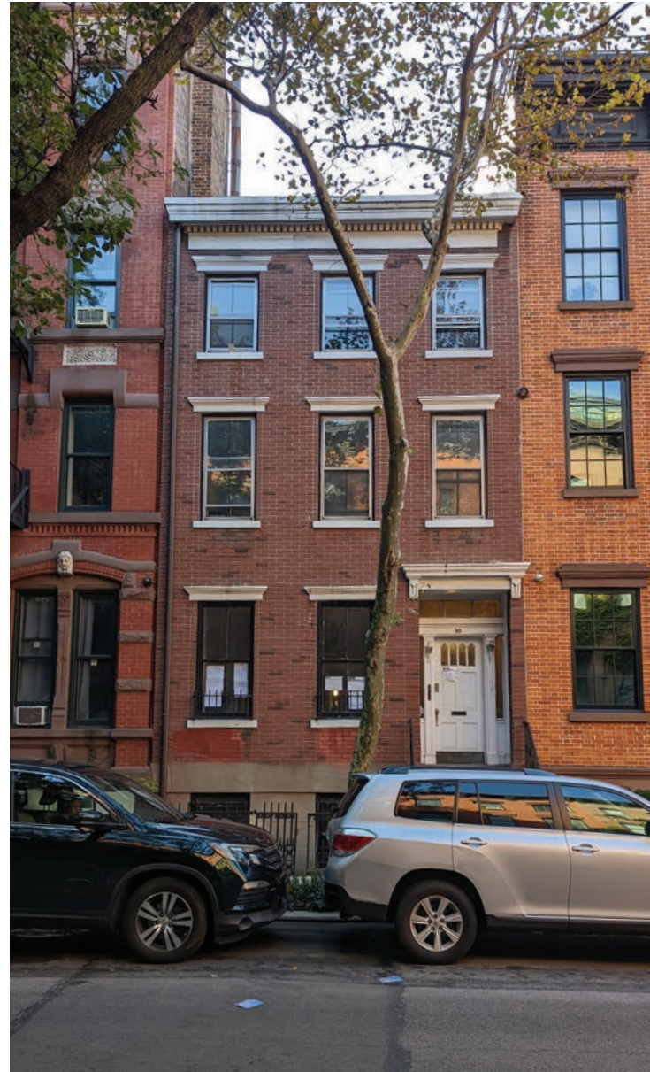
02. 90 CHARLES STREET FRONT FACADE (NORTH)
