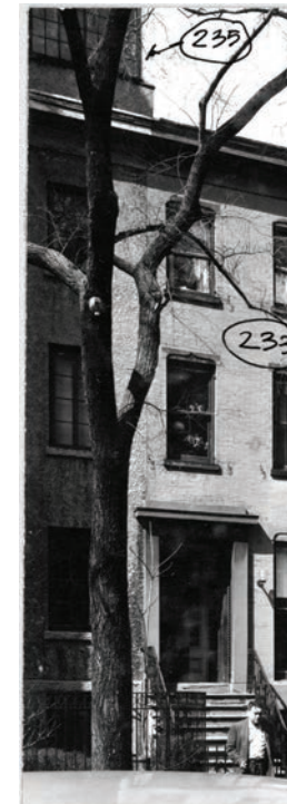
235 West 11th Street at designation District: Greenwich Village Built: 1844. Finish: Brown rough stucco over brick
