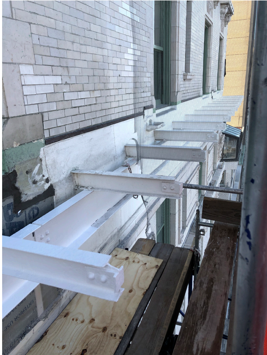
Existing Balcony Structure: C-Channel and Outriggers
