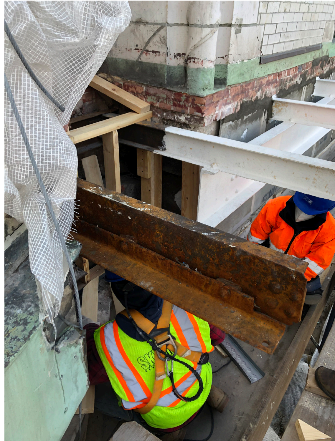
Existing Balcony Structure: C-Channel and Outriggers
