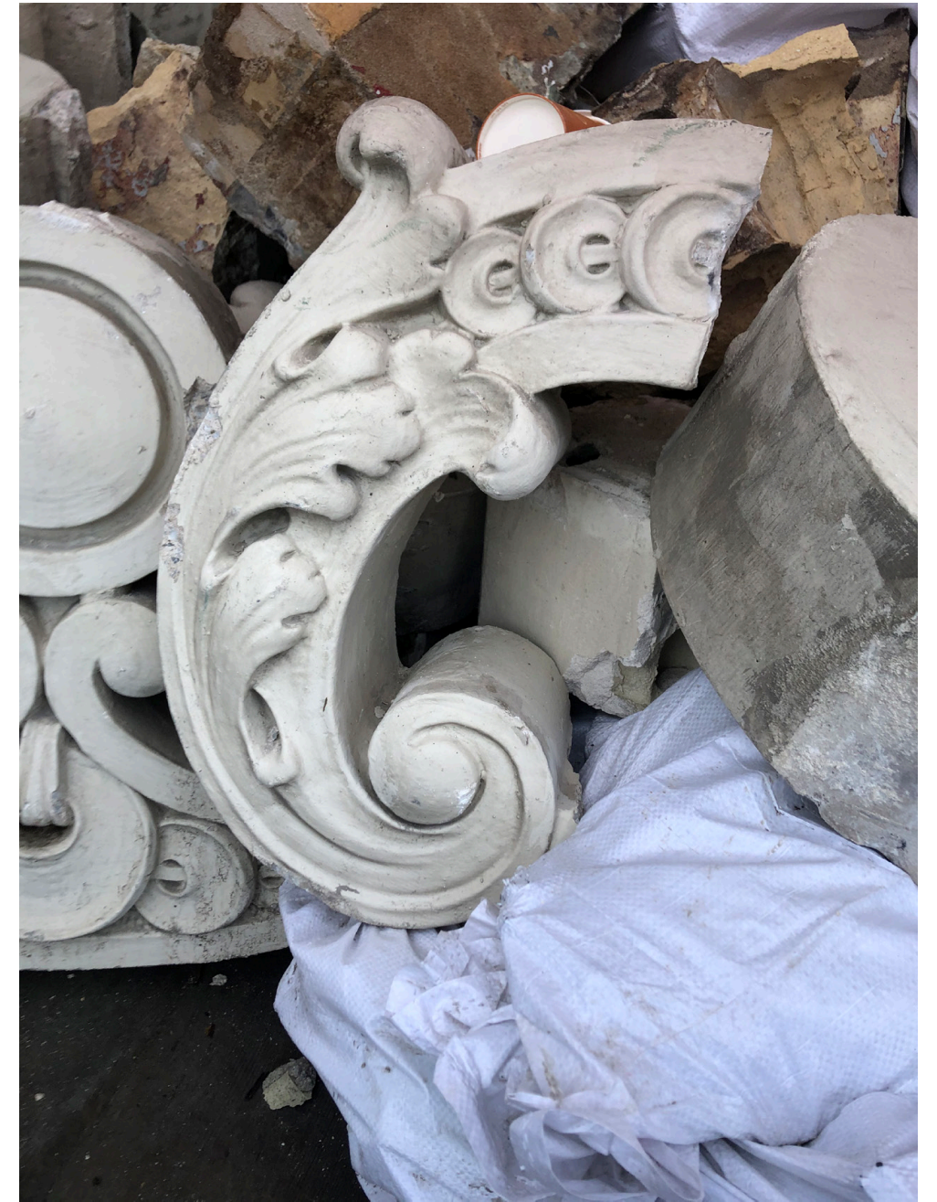
Examples of Retained Original Terracotta Pieces for Casting
