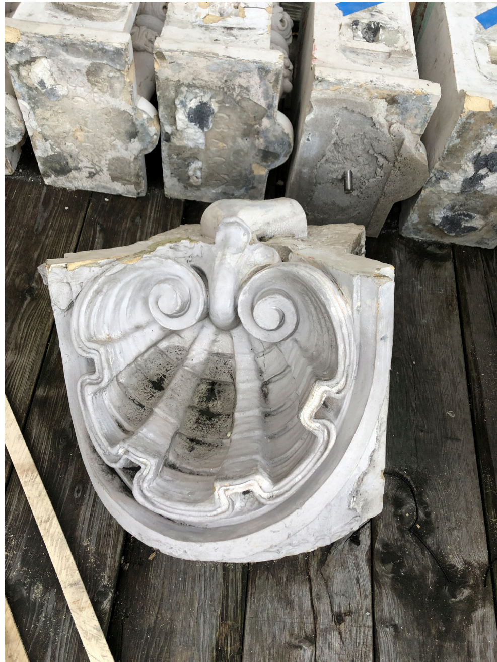
Examples of Retained Original Terracotta Pieces for Casting
