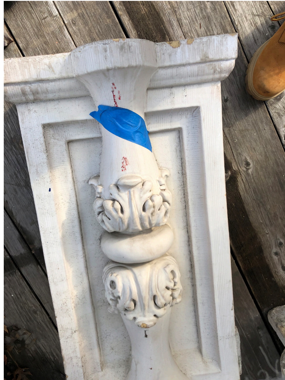
Examples of Retained Original Terracotta Pieces for Casting
