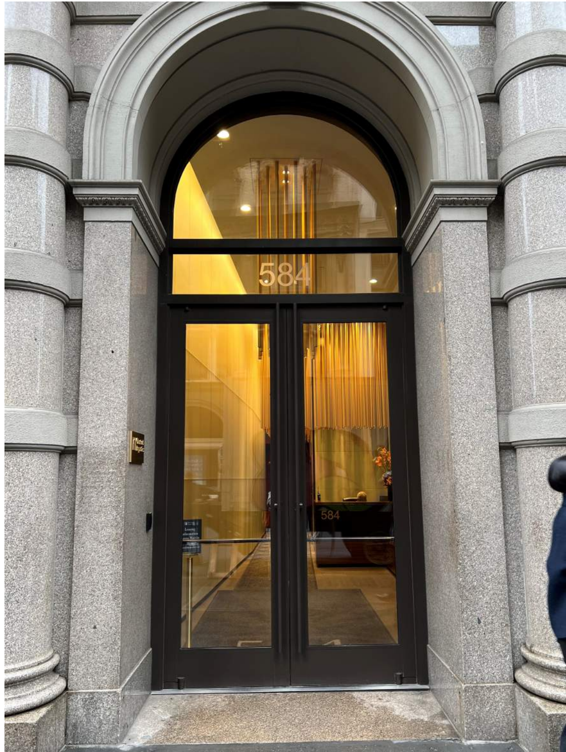
Entry Door at Neighboring 584 Broadway (Approved for 584 and 588 Bway at 2014 Public Hearing)
