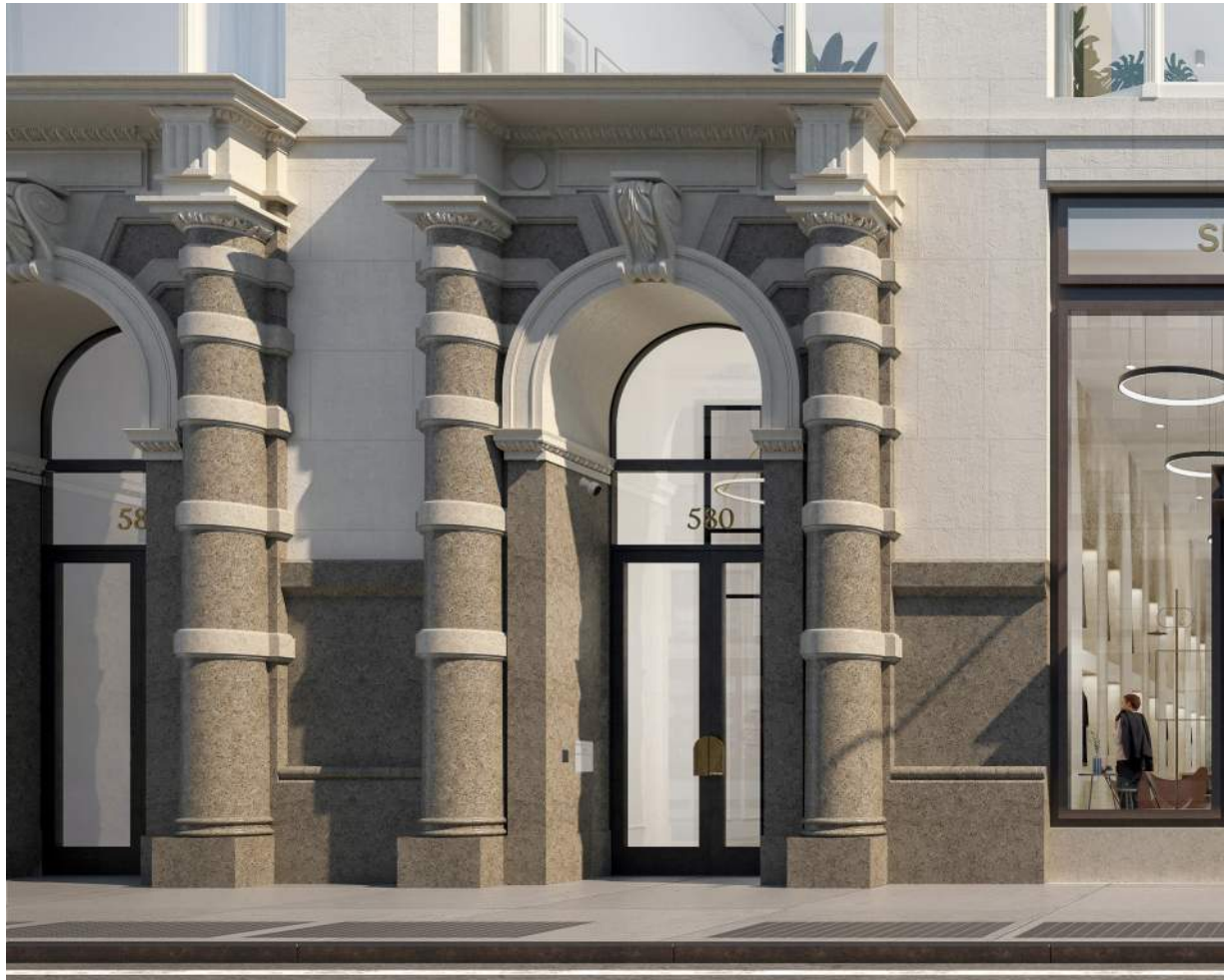
Broadway Entry Door Replacement
