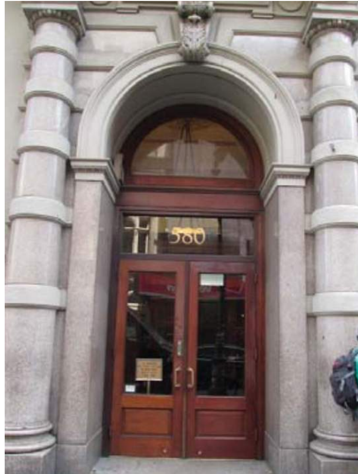
Existing Condition at 580 Broadway
