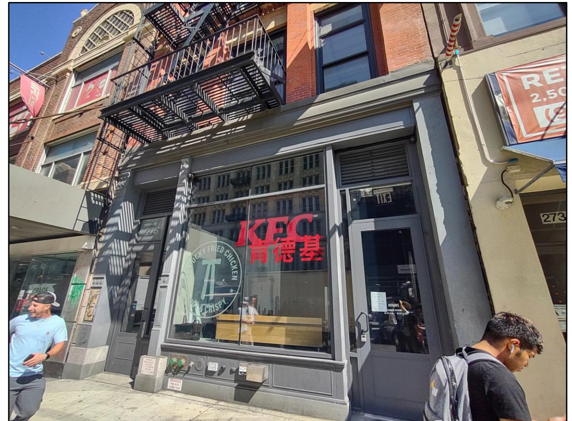
275 Canal Street, storefront alteration per CofA 19-25667. (September 2022)
