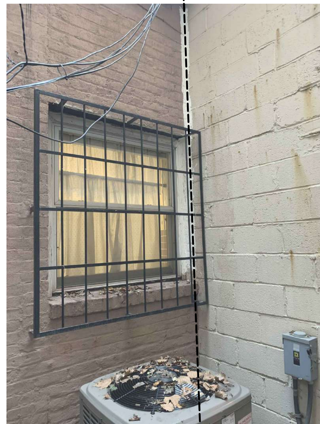
253 HICKS STREET 2 GRACE COURT ALLEY
