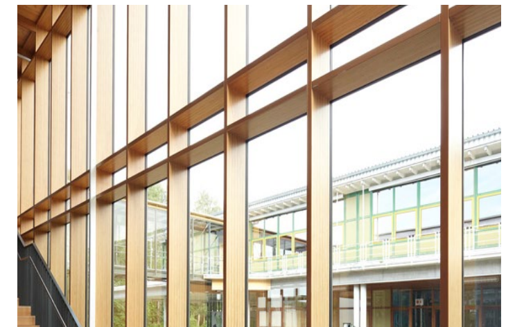
Wood Framed Atrium
