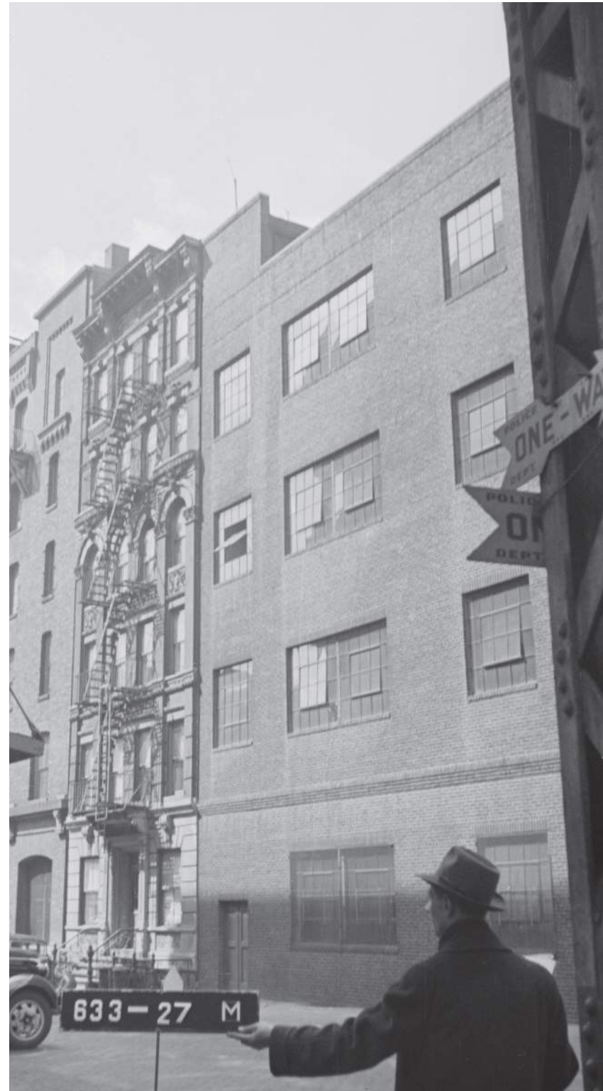
1940 TAX PHOTO, PERRY STREET ELEVATION (MUNICIPAL ARCHIVES)
