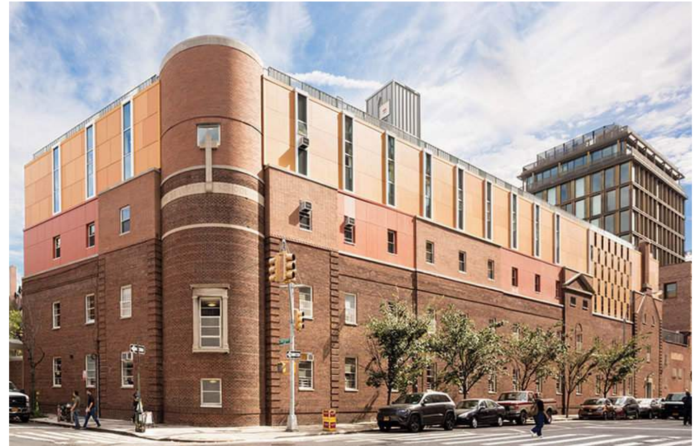
ST. LUKE'S SCHOOL (ANDREW BARTLE ARCHITECTS)
