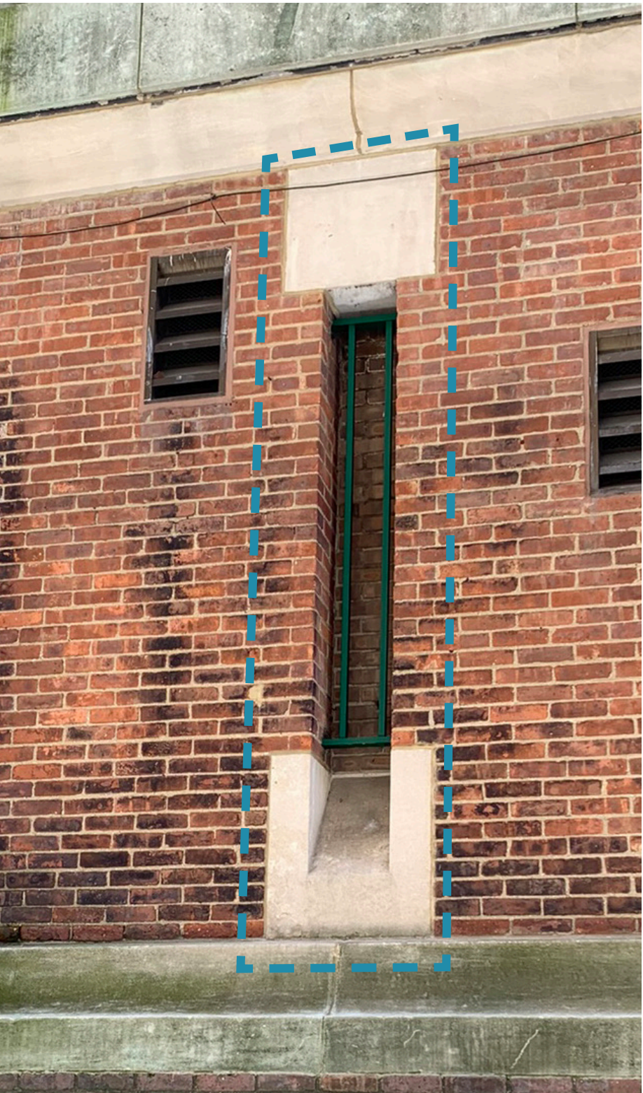
EXISTING DRILL HALL WINDOWS ARE BLOCKED WITH BRICK
