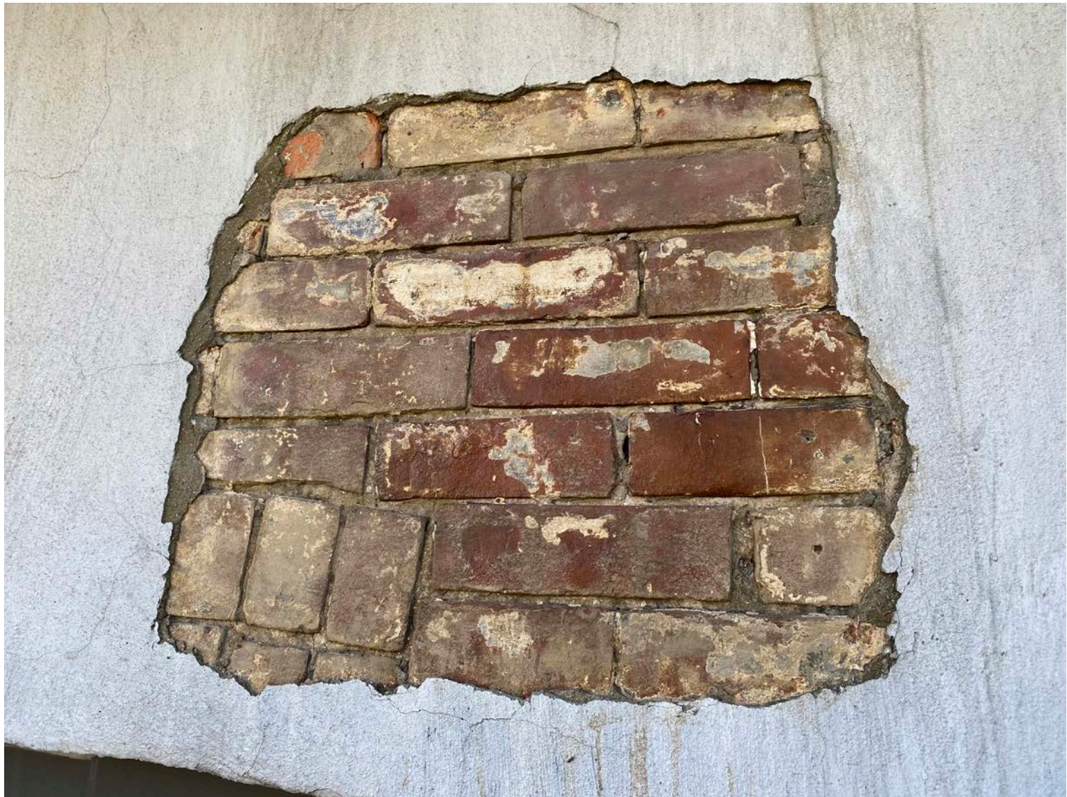
ZOOM ON THE STUCCO REMOVAL SAMPLE
