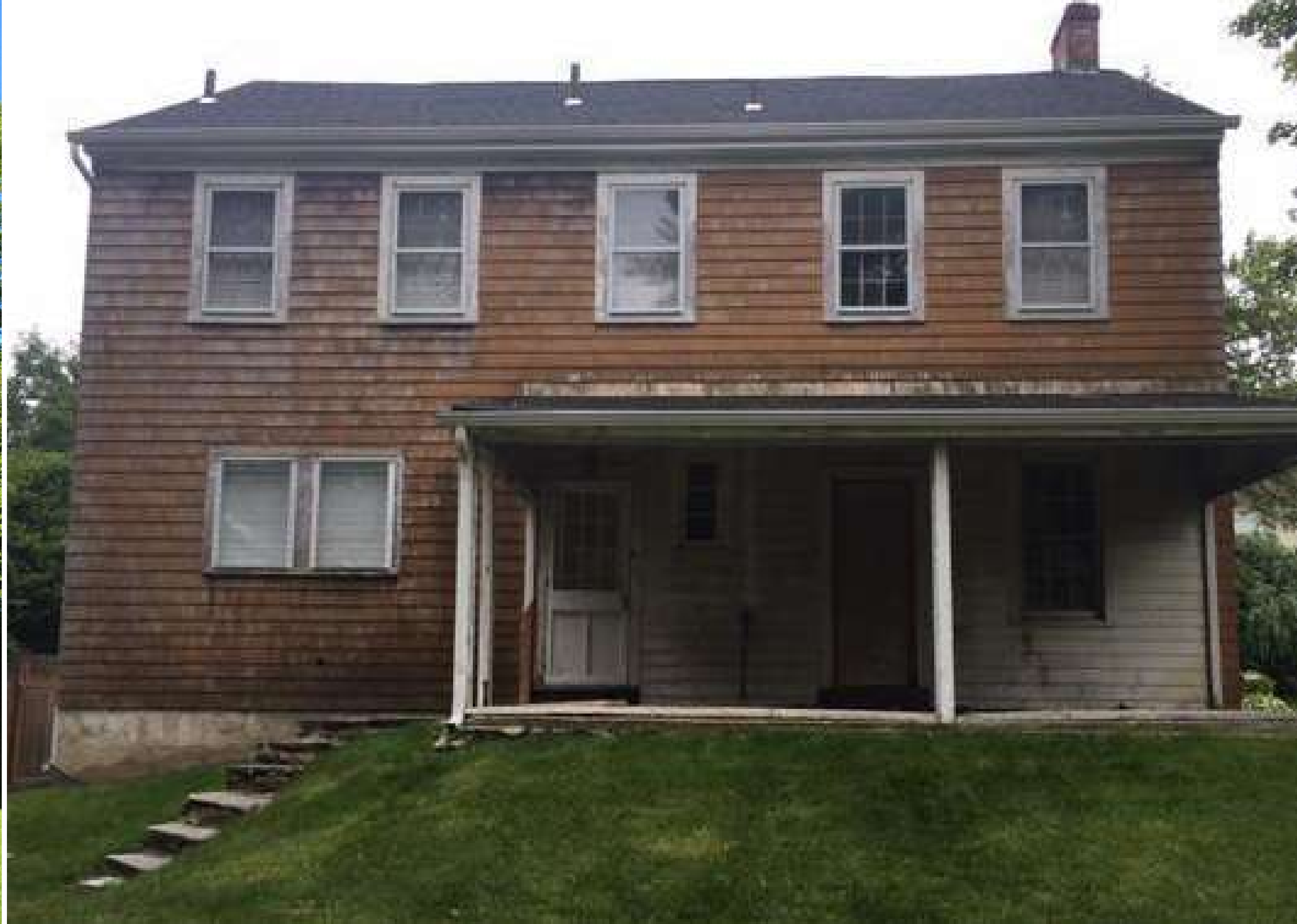
EXISTING NORTH (BACK) FACADE
