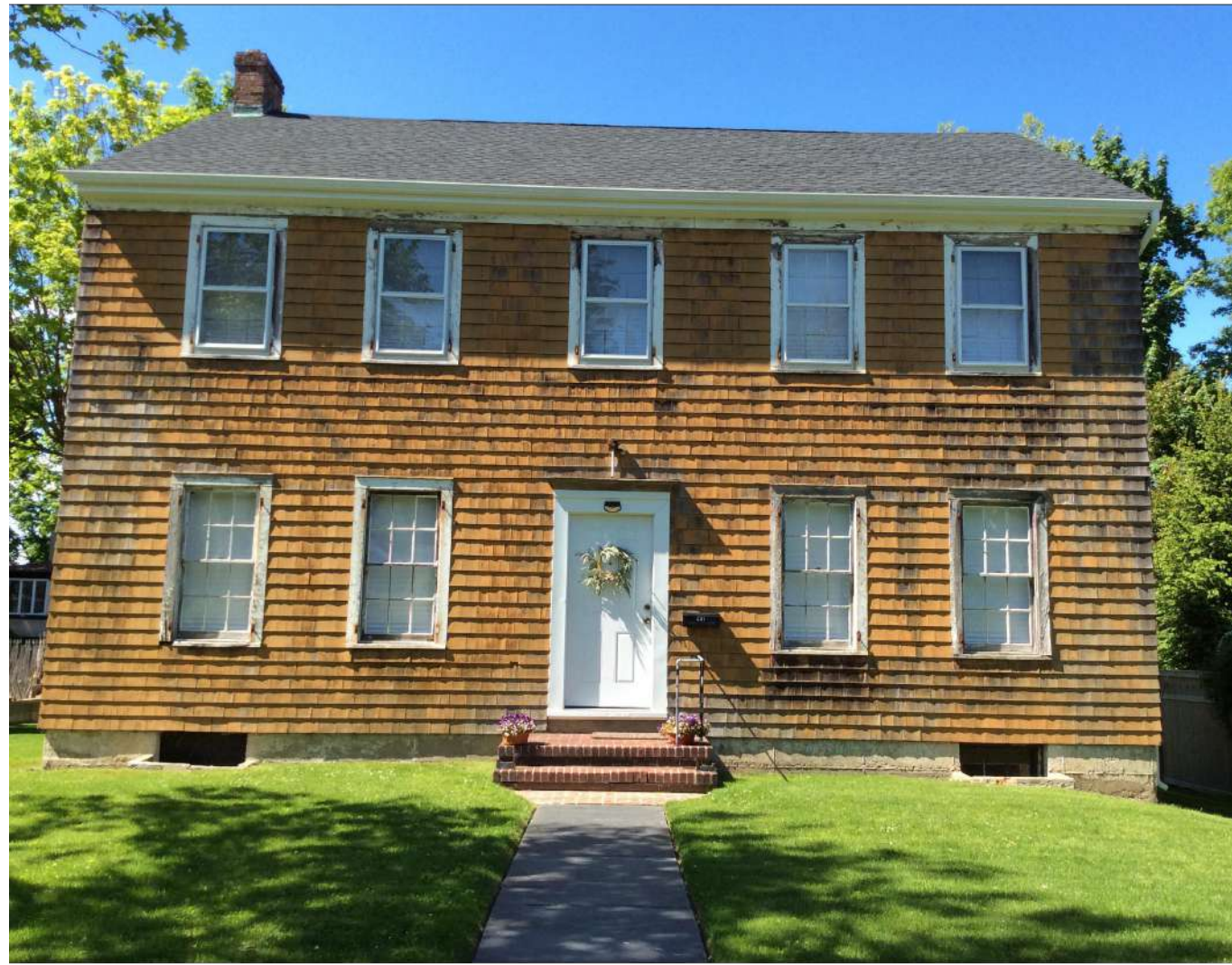
EXISTING SOUTH FACADE
