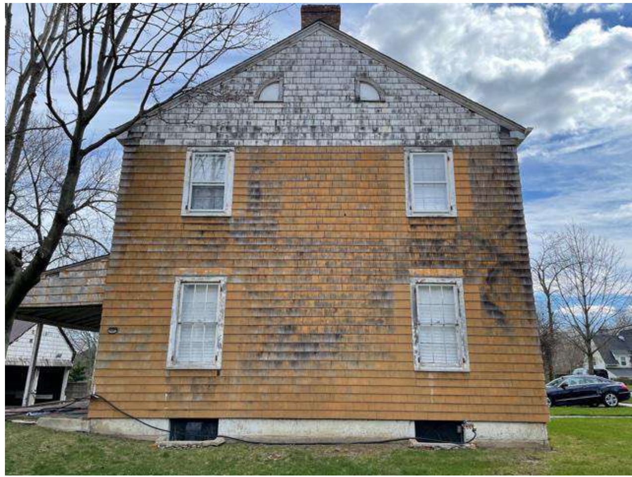
EXISTING EAST FACADE
