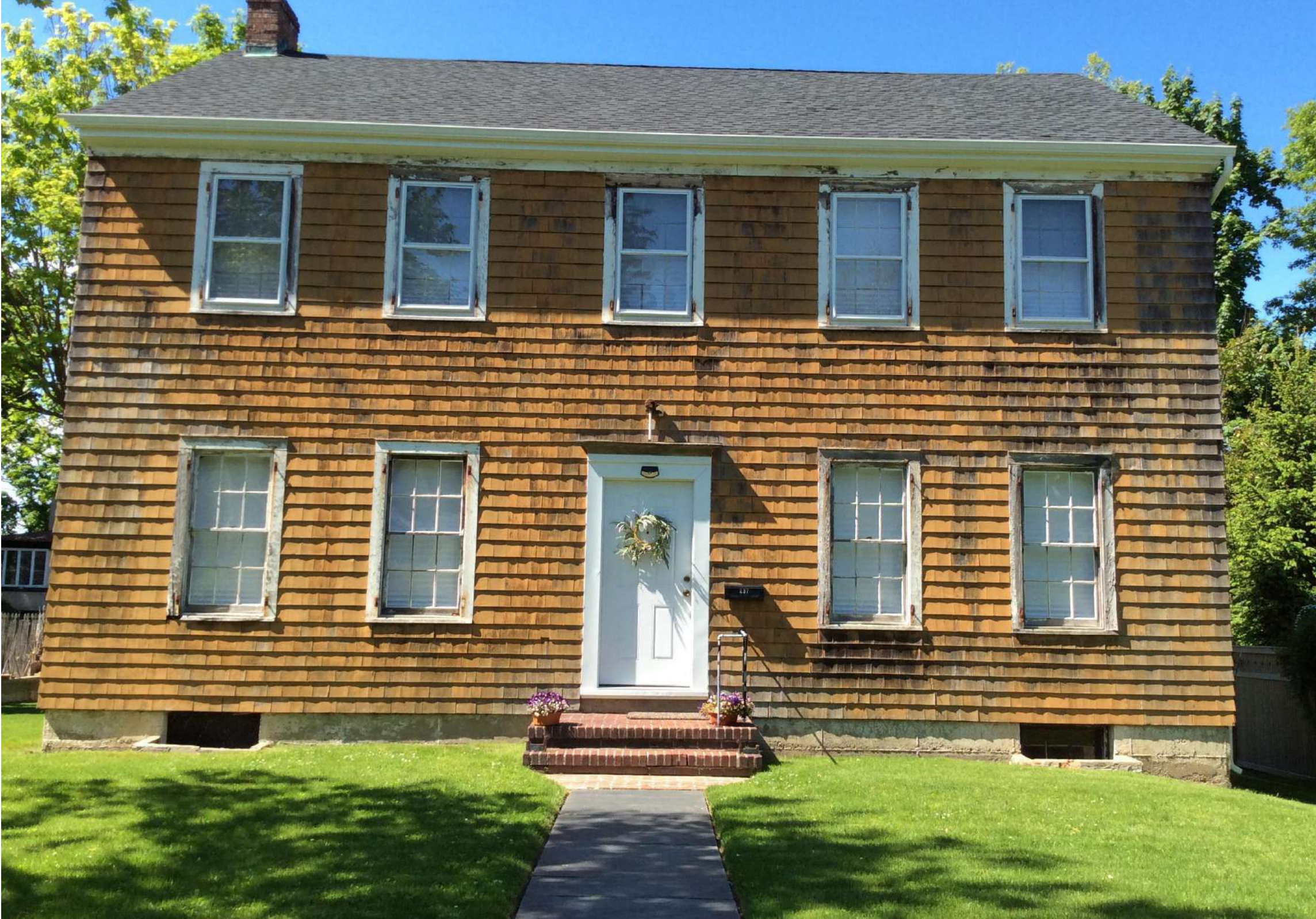
EXISTING SOUTH (FRONT) FACADE
