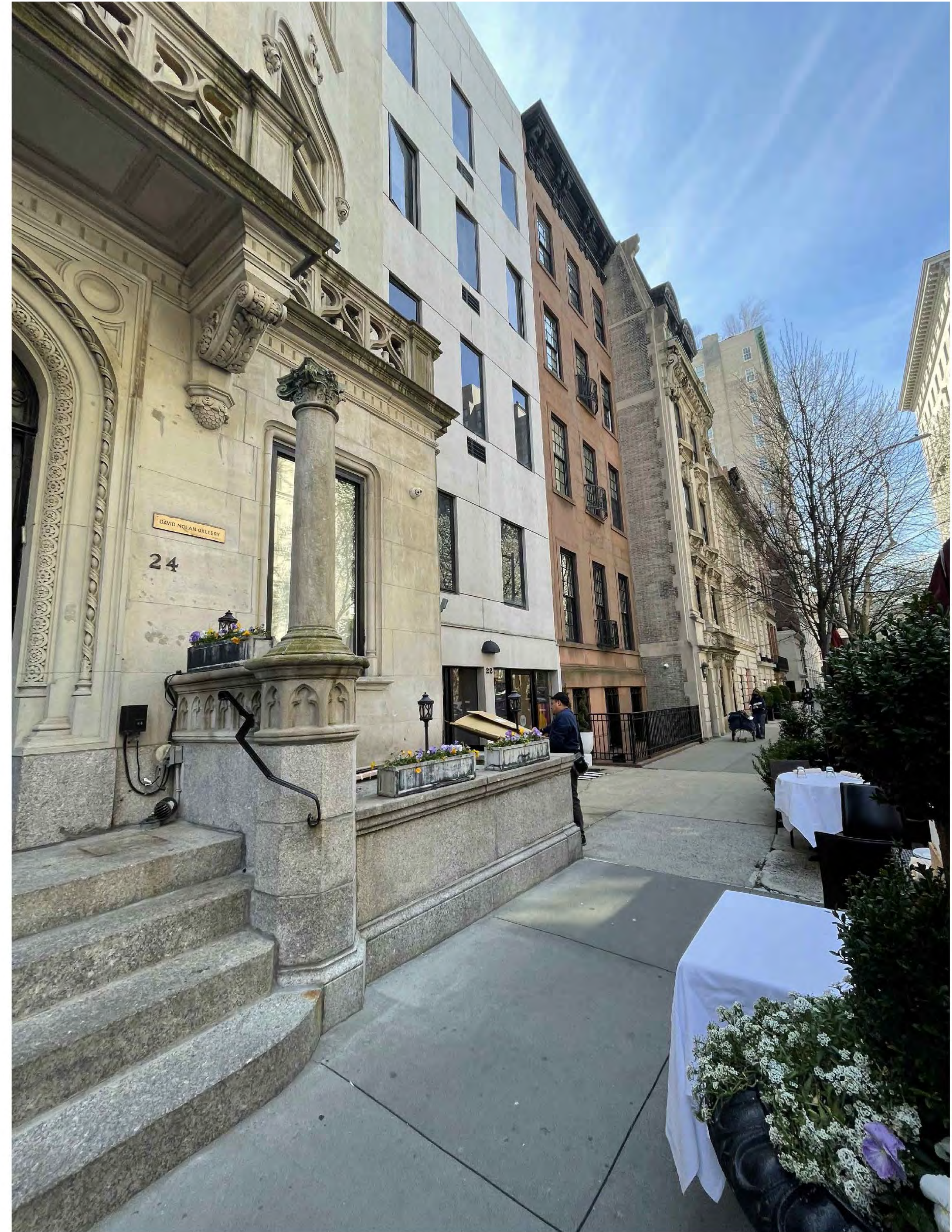
22 E 81ST ST - EXISTING PHOTO Scale N.T.S.
