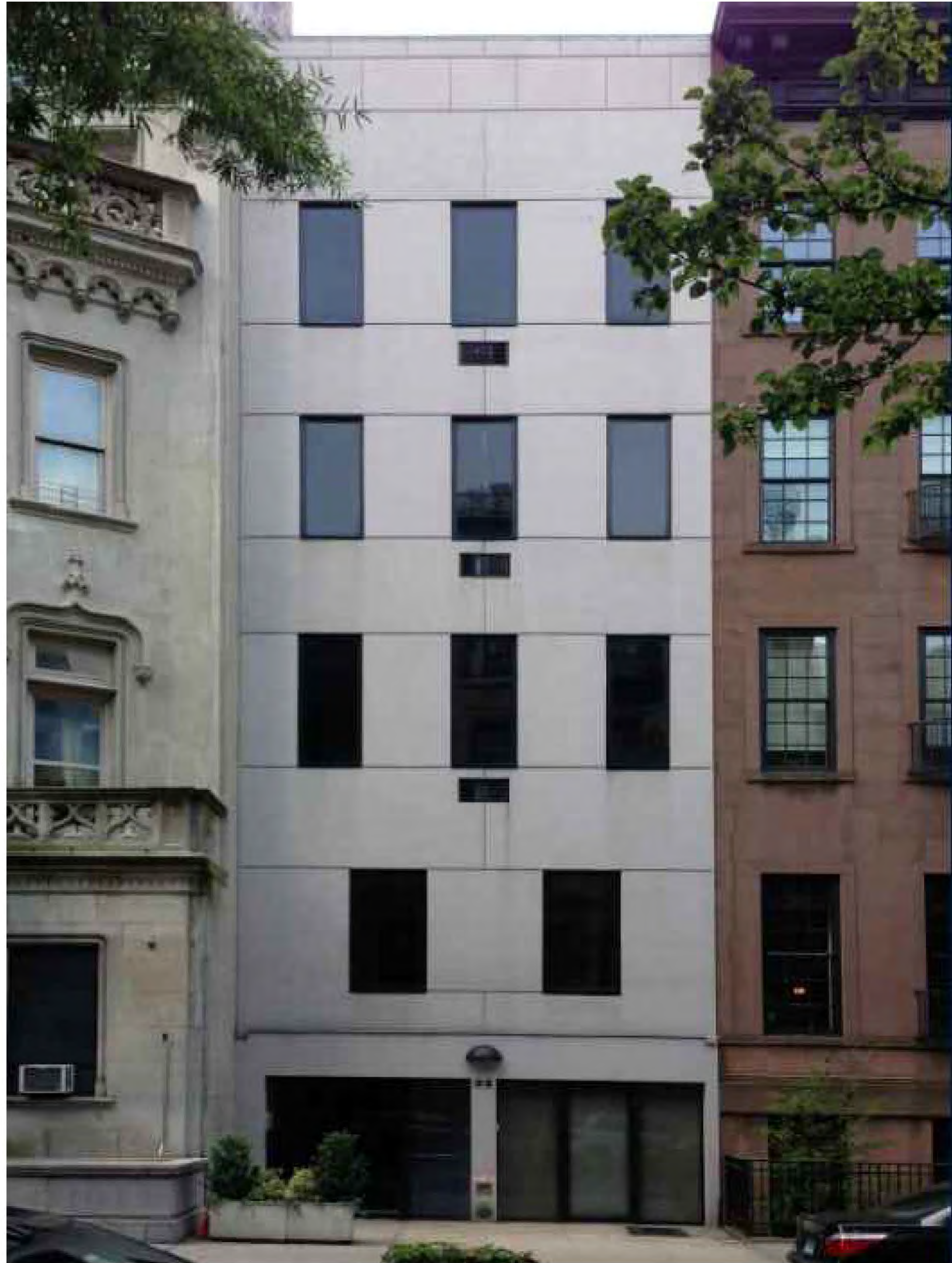
22 E 81ST ST - EXISTING PHOTO Scale N.T.S.
