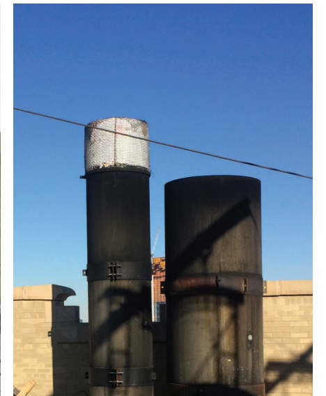
② EXISTING VENT STACK LOOKING SOUTH
