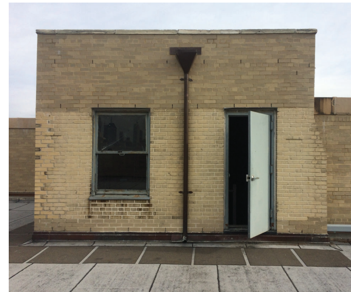
① EXISTING BULKHEAD LOOKING EAST
