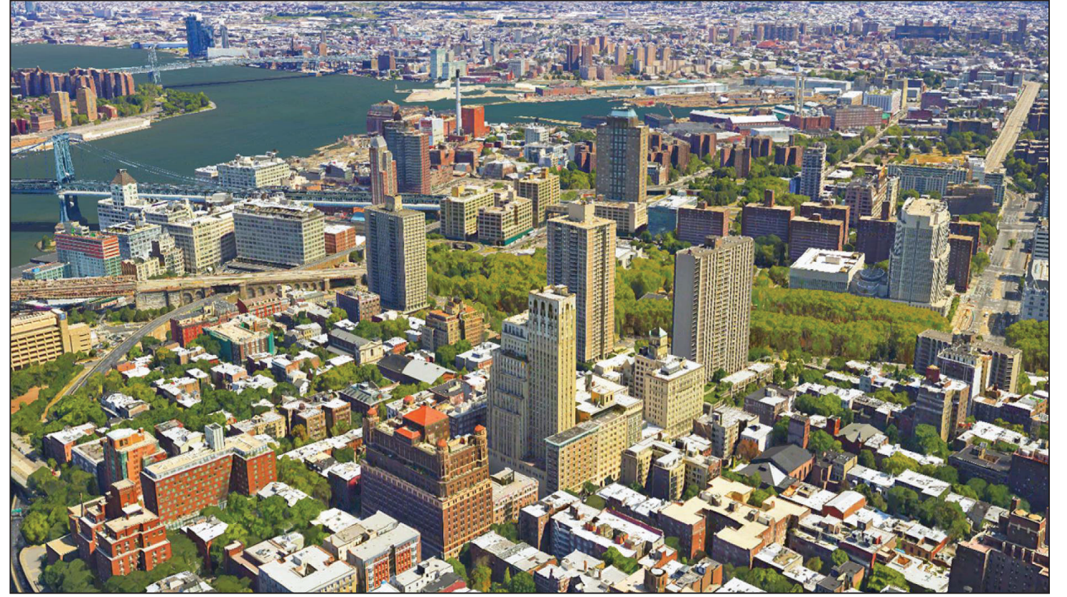
View from west
