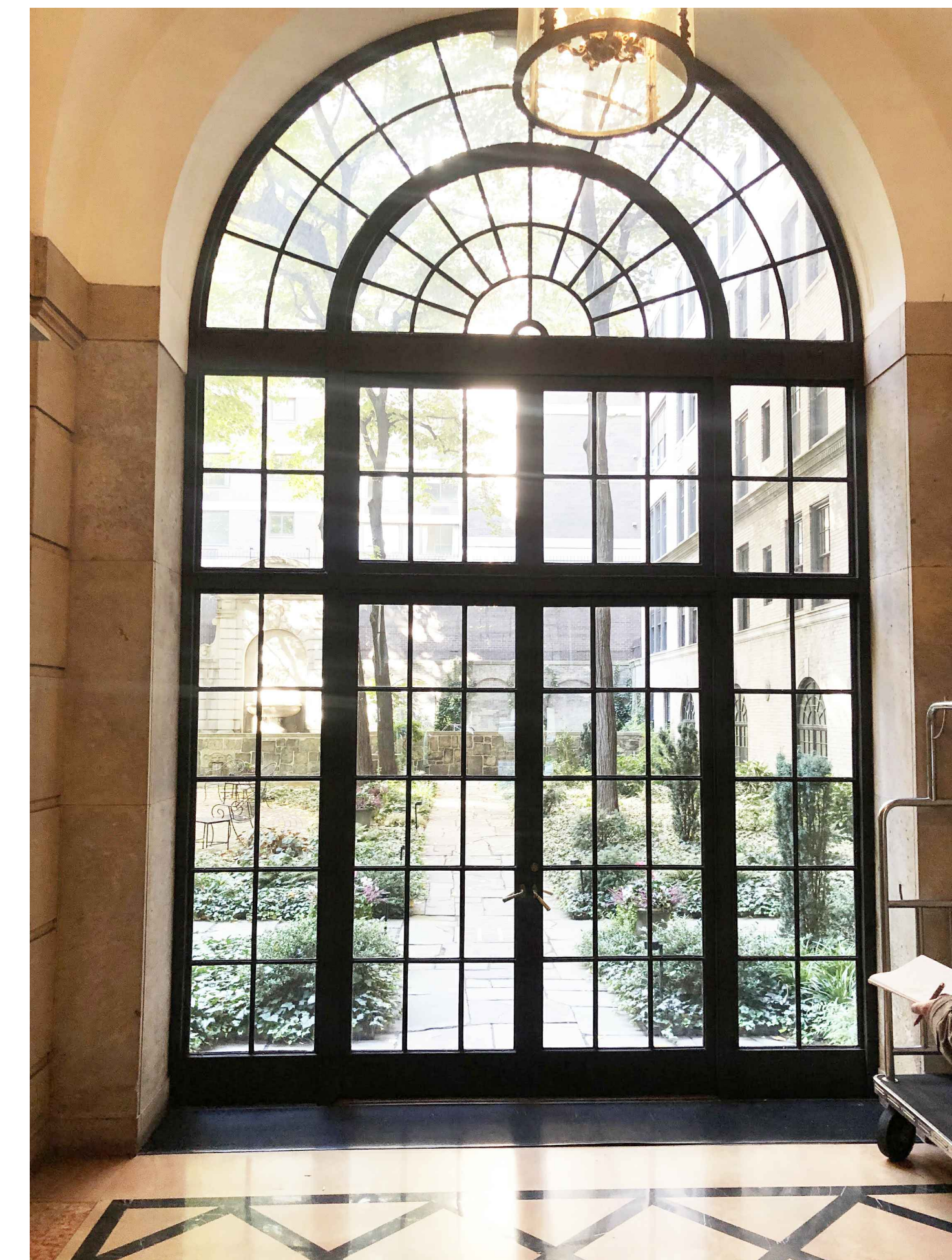
03 VIEW OF DOORS FROM LOBBY TO COURTYARD NOT TO SCALE
