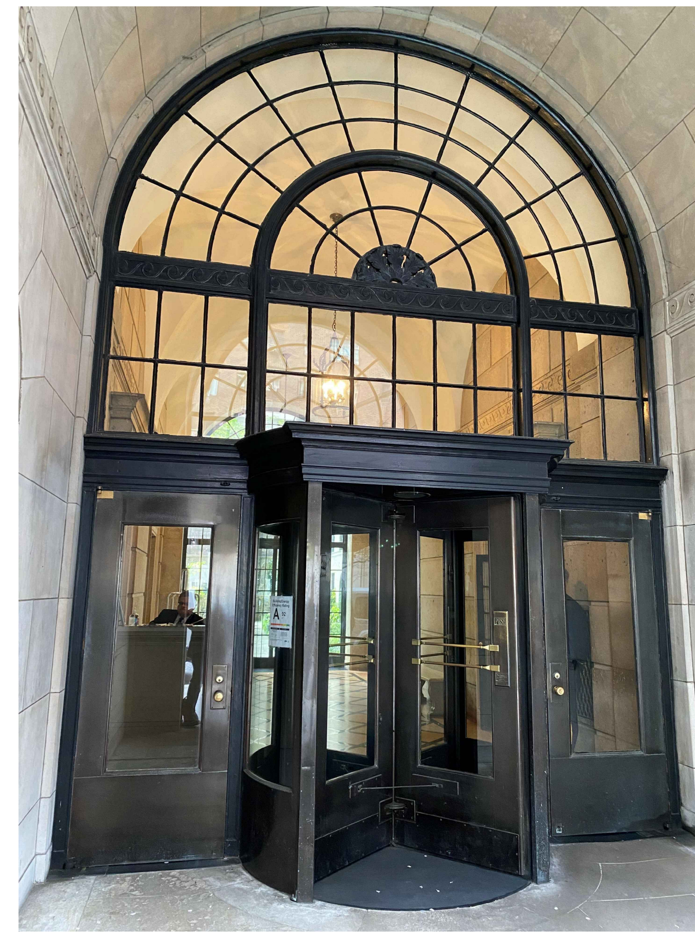
05 VIEW FROM VESTIBULE OF EXISTING ENTRY DOORS NOT TO SCALE
