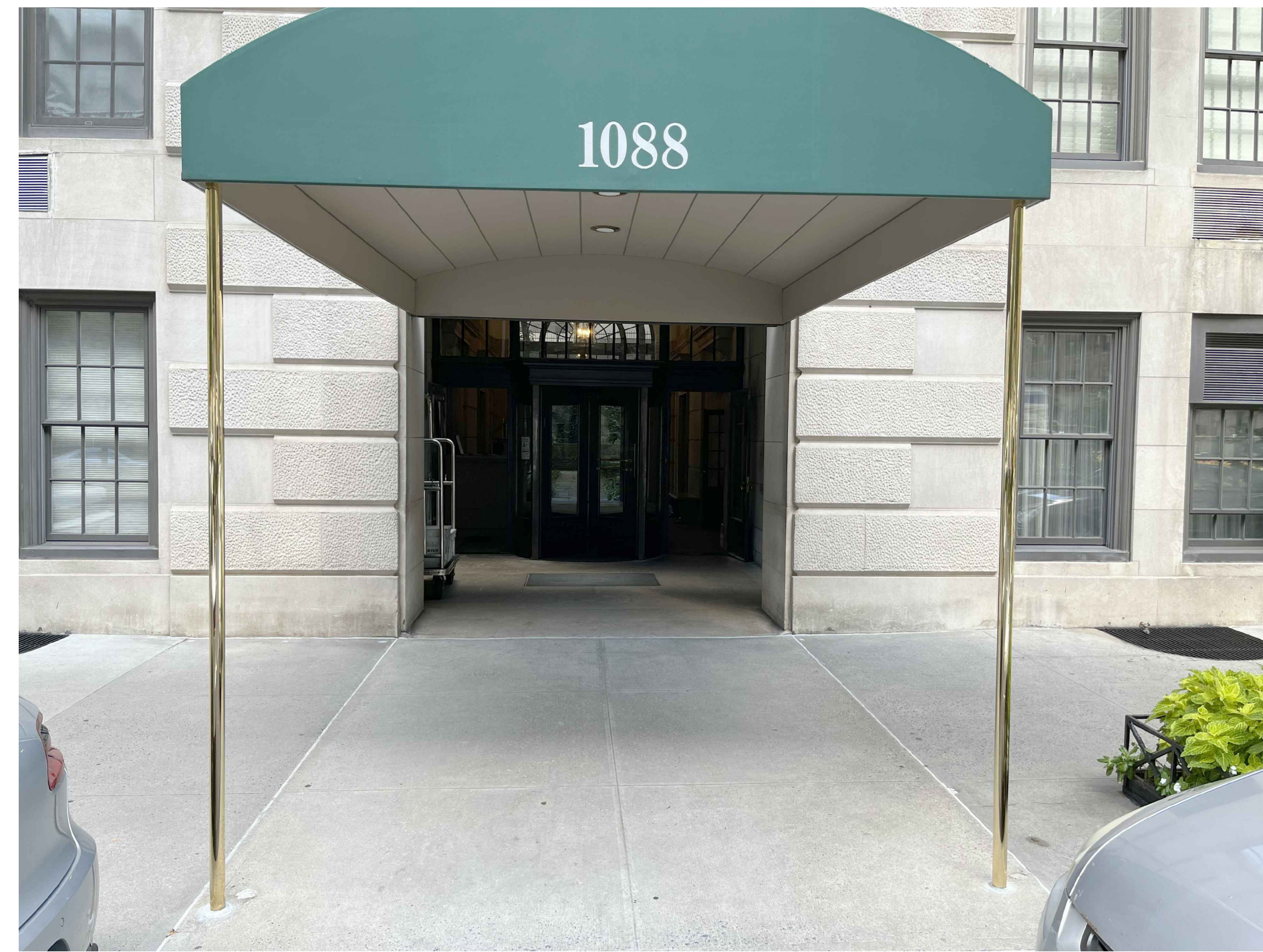
07 VIEW FROM SIDEWALK OF EXISTING ENTRY DOORS NOT TO SCALE
