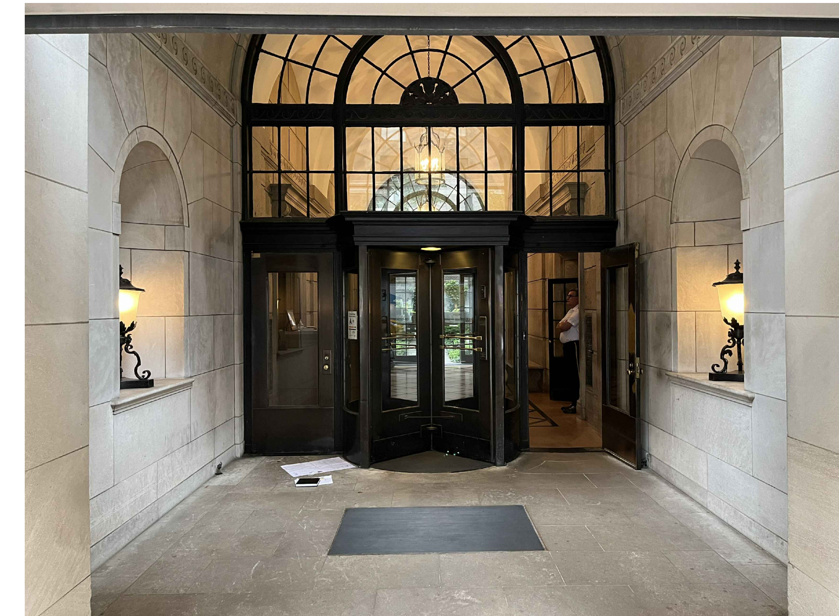
09 OVERALL VIEW OF ENTRY DOORS FROM VESTIBULE NOT TO SCALE
