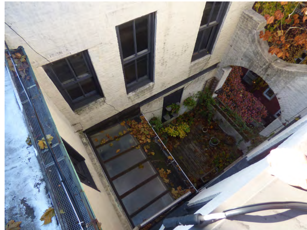
VIEW OF THE INTERIOR COURT LOOKING DOWN FROM THE ROOF
