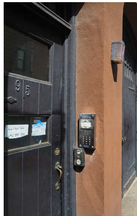
CURRENT ENTRANCE DOOR (TO BE REPLACED)
