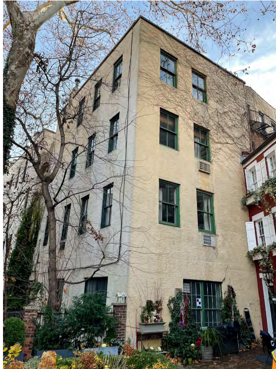
OVERALL VIEW OF THE REAR FROM GROVE COURT, A NON-PUBLIC ALLEY
