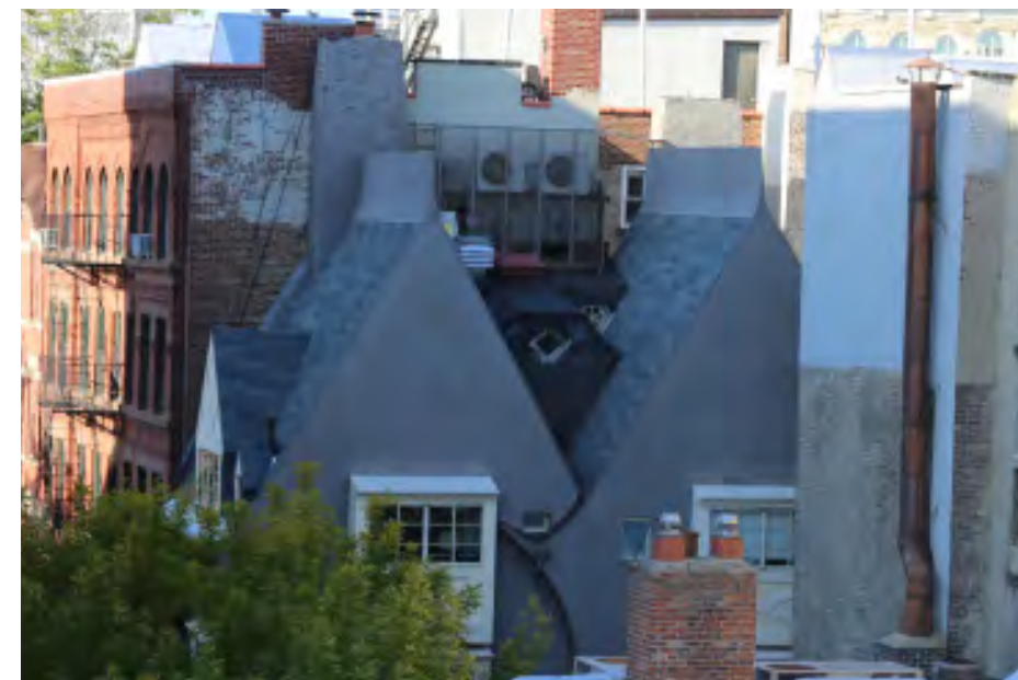
EXPRESSIVE ROOFS (AS SEEN FROM 95 BEDFORD ST)
