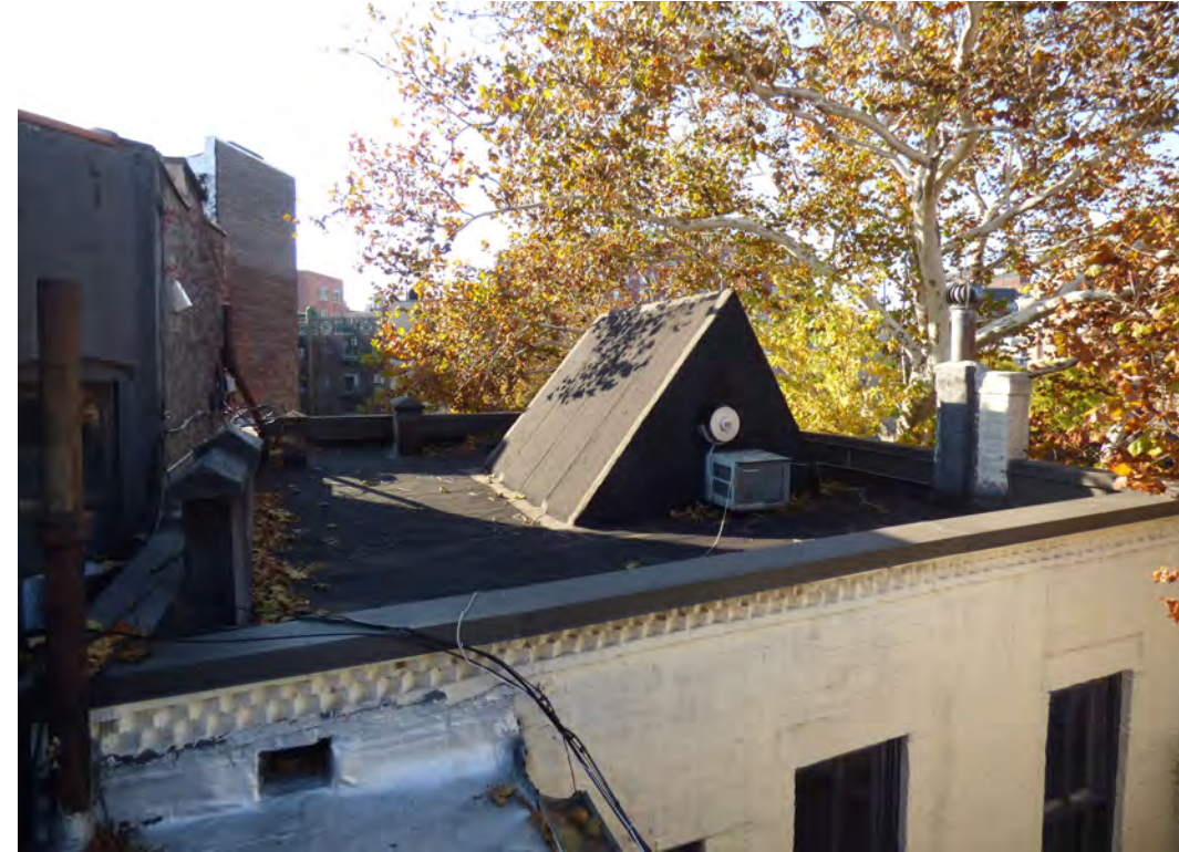
VIEW OF THE ROOF AT THE REAR SECTION OF THE BUILDING
