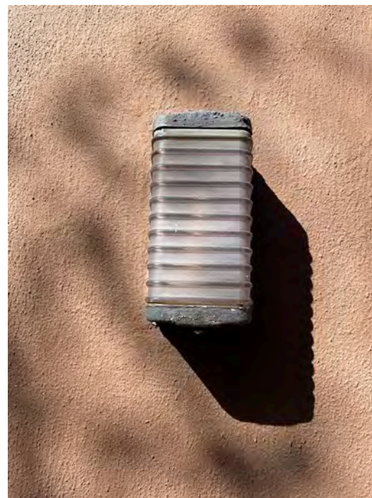
CURRENT LIGHT FIXTURE (TO BE REPLACED)
