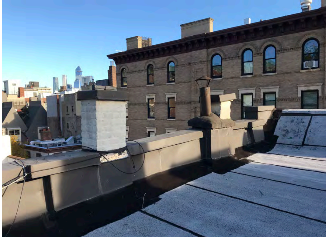
VIEW OF THE ROOF AT THE FRONT SECTION OF THE BUILDING
