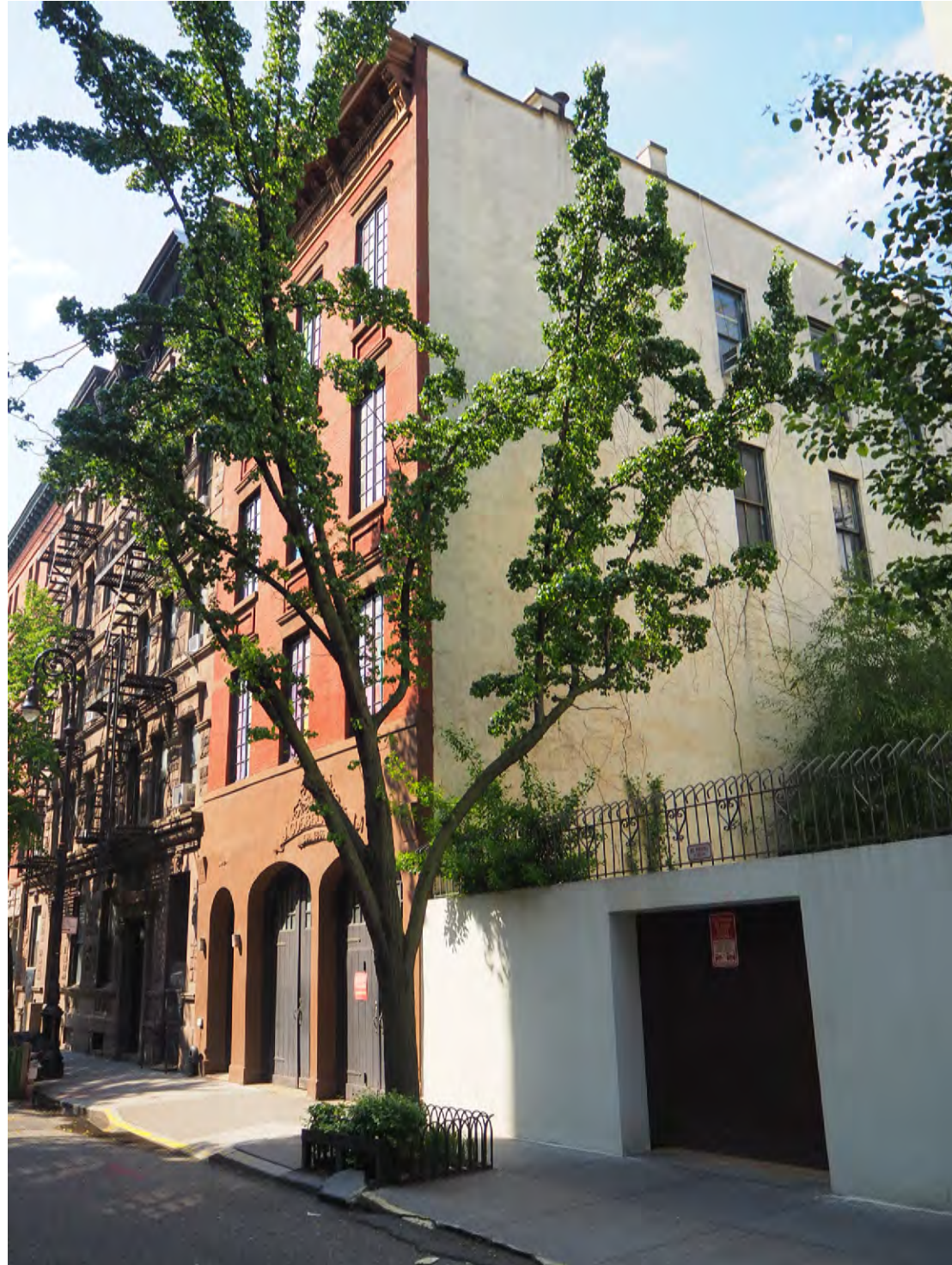
OVERALL VIEW OF THE BUILDING
