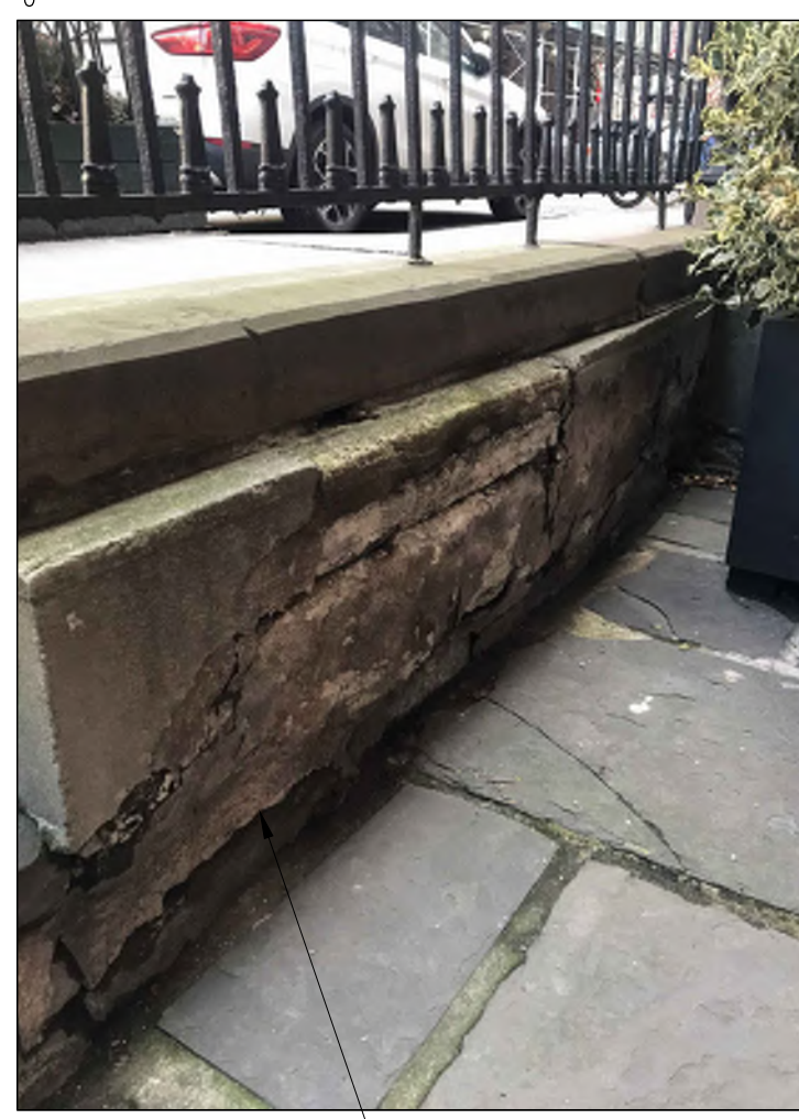
EXISTING AREAWAY WALL TO BE REPLACED WITH BROWNSTONE COLORED STUCCO FINISH CONCRETE
