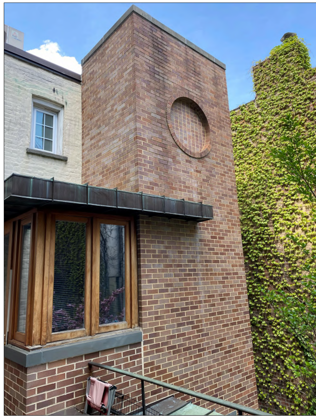
02 CURRENT PHOTO: REAR FACADE L-001 N.T.S.
