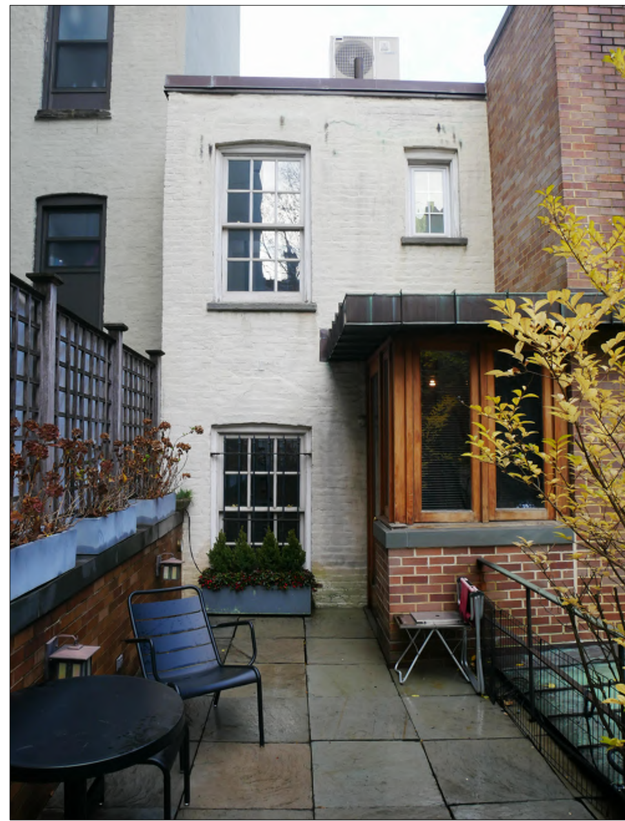
01 CURRENT PHOTO: REAR FACADE L-001 N.T.S.
