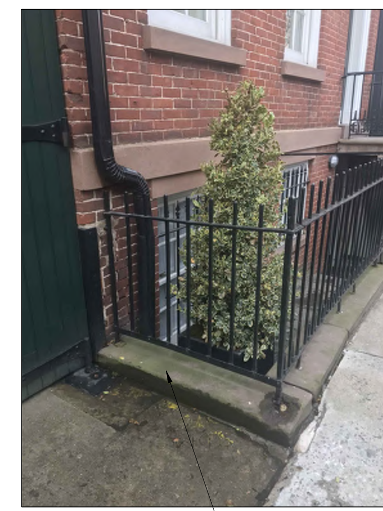
EXISTING BROWNSTONE COPING STONES TO BE REINSTALLED ON NEW BROWNSTONE FINISH AREAWAY WALL
