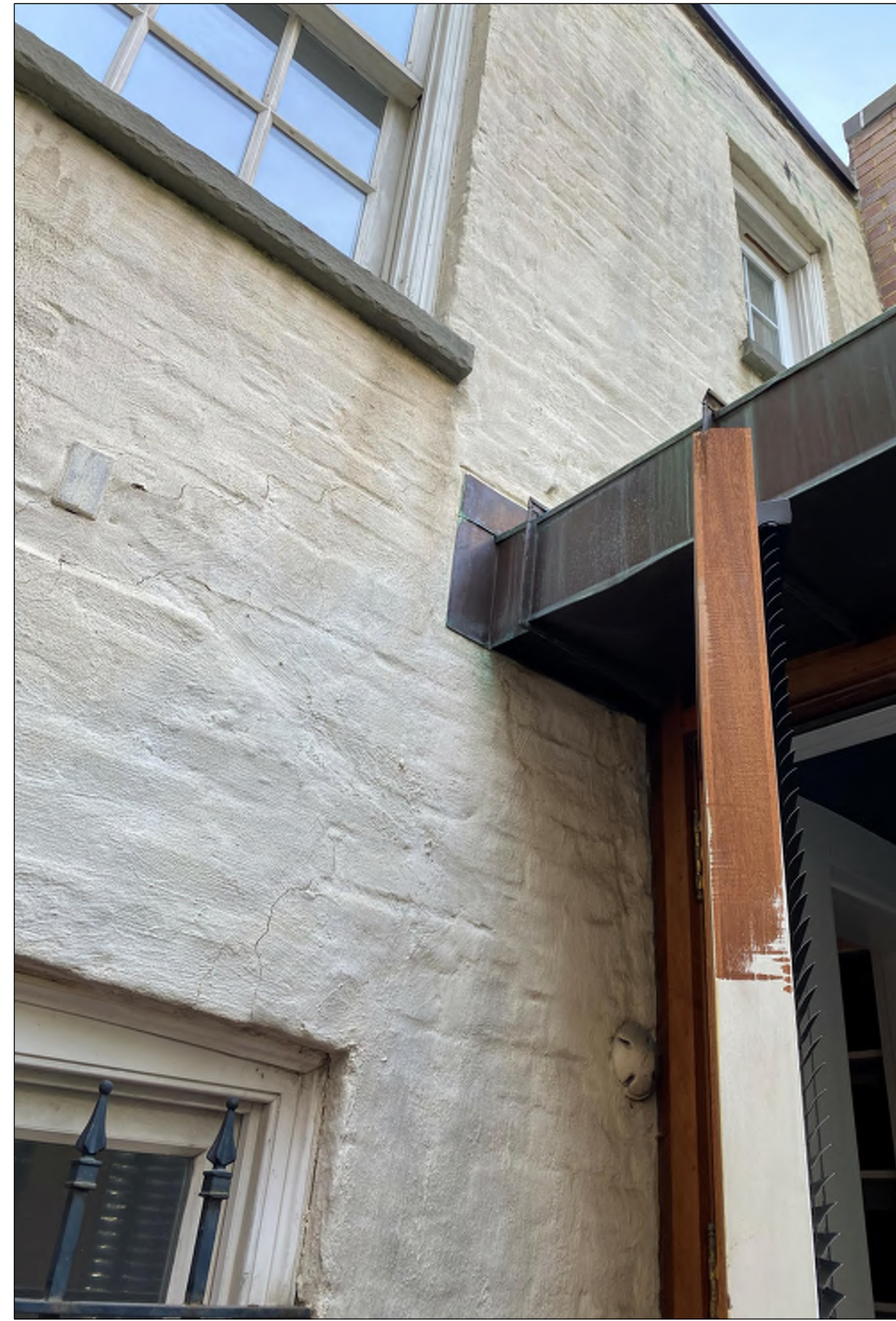
05 CURRENT PHOTO: REAR FACADE L-001 N.T.S.
