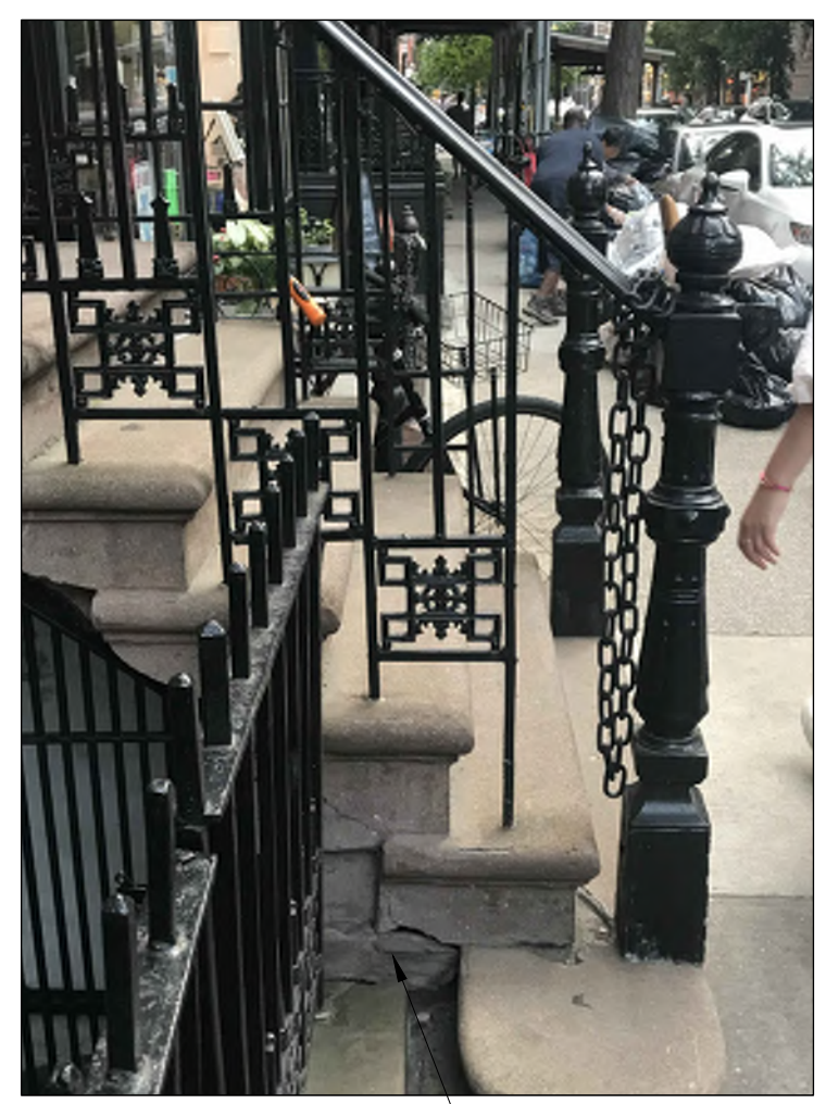
EXISTING CRACKED AND DETERIORATED STUCCO
