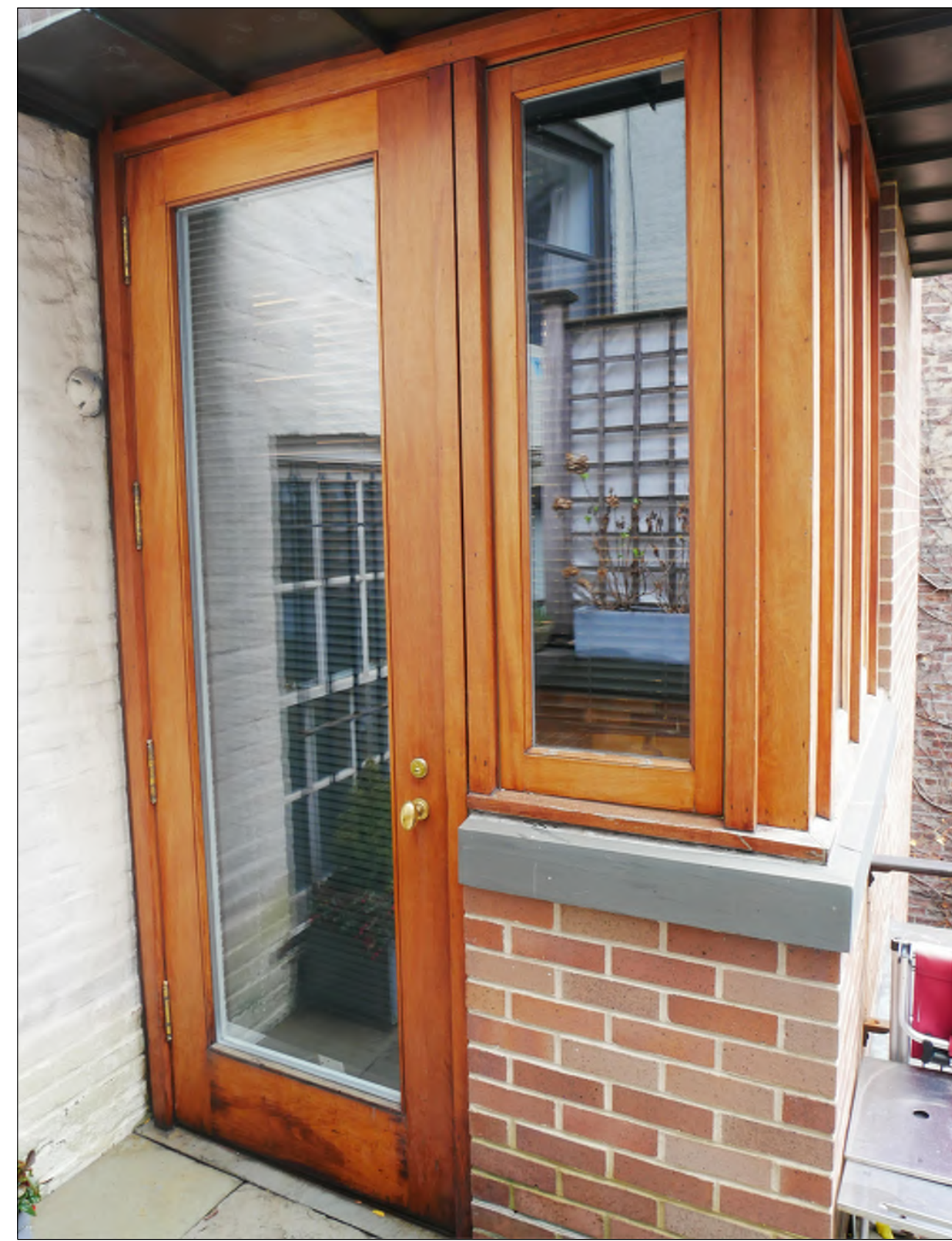
04 CURRENT PHOTO: REAR FACADE L-001 N.T.S.
