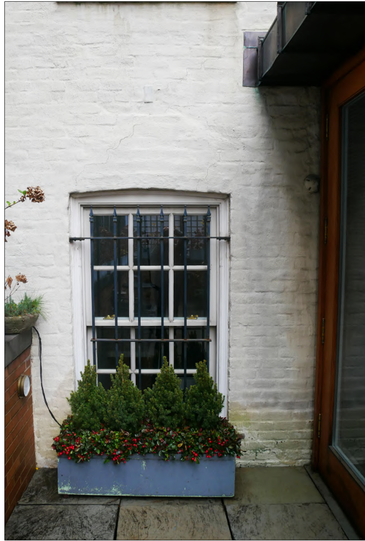
06 CURRENT PHOTO: REAR FACADE L-001 N.T.S.
