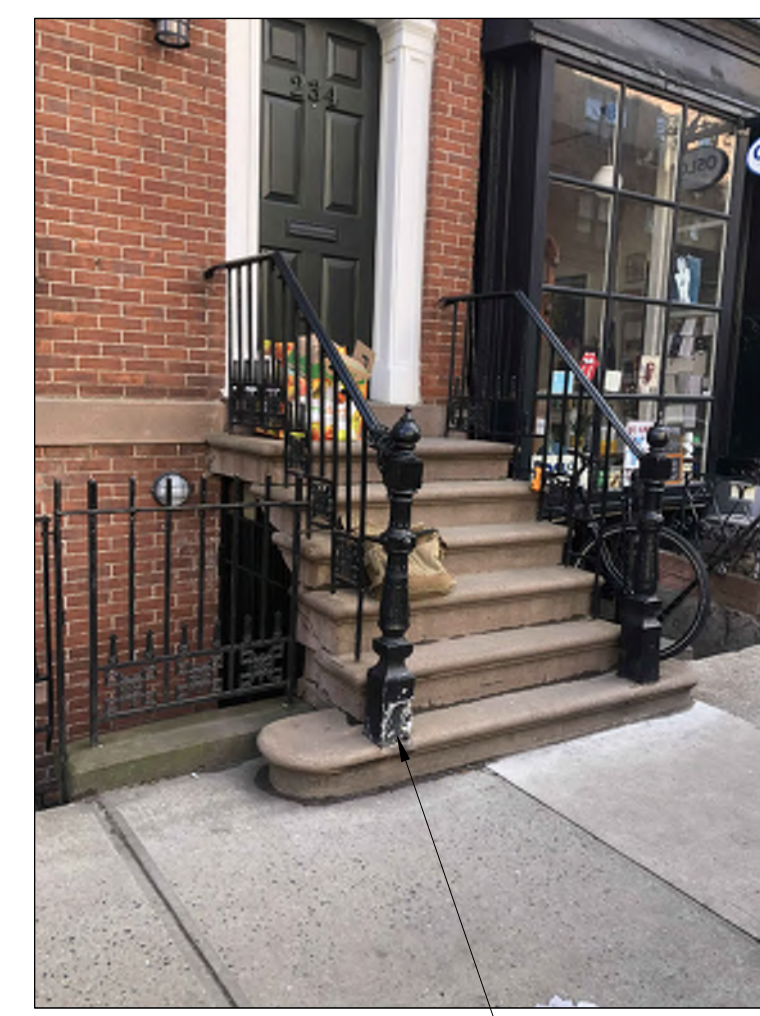
EXISTING DAMAGED NEMEL POST TO BE RESTORED, PAINTED, AND REINSTALLED ON NEW STOOP MATCHING EXISTING IN CONFIGURATION AND FINISH
