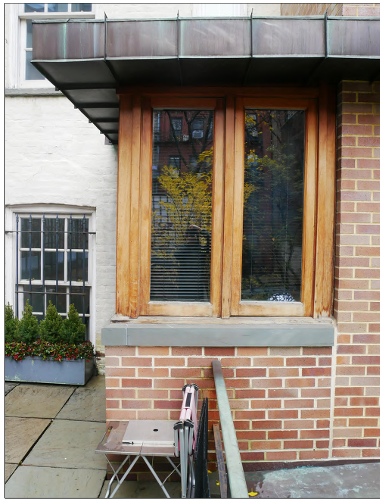
03 CURRENT PHOTO: REAR FACADE L-001 N.T.S.
