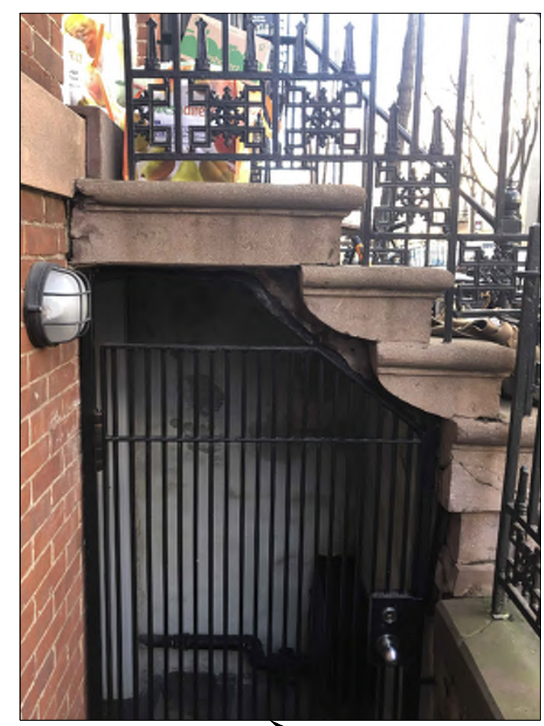
EXISTING DAMAGED NEMEL POST TO BE RESTORED, PAINTED, AND REINSTALLED ON NEW STOOP MATCHING EXISTING IN CONFIGURATION AND FINISH
