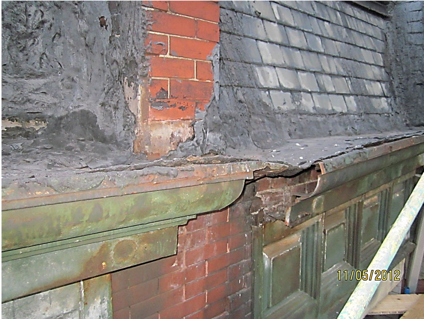
231 West 75 th Street (Severe deterioration of underlying brick at Mansard and Turret Roof Differential Façade Settlement visible at misaligned gutters.)
