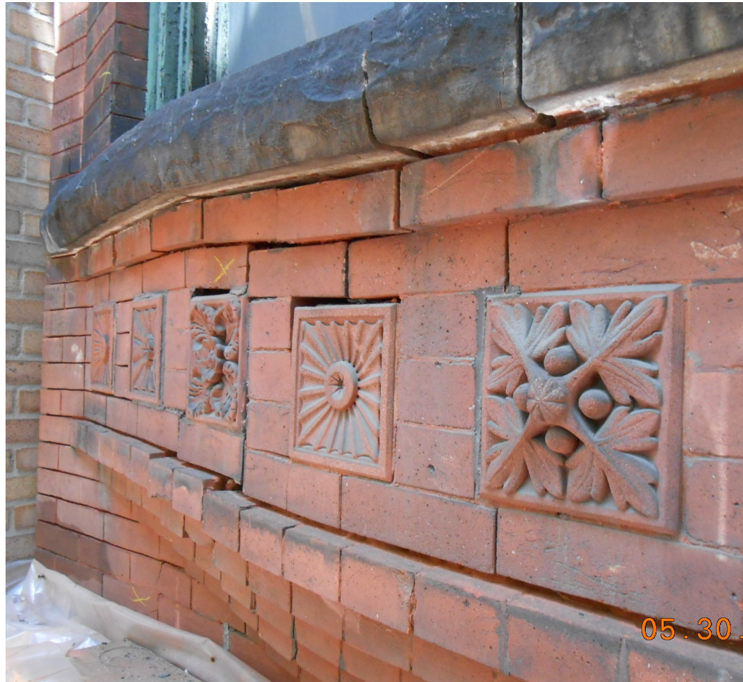
233 West 75 th Street (Projecting bow window. masonry severely displaced vertically and horizontally from settlement of the facades) Photos taken 2012
