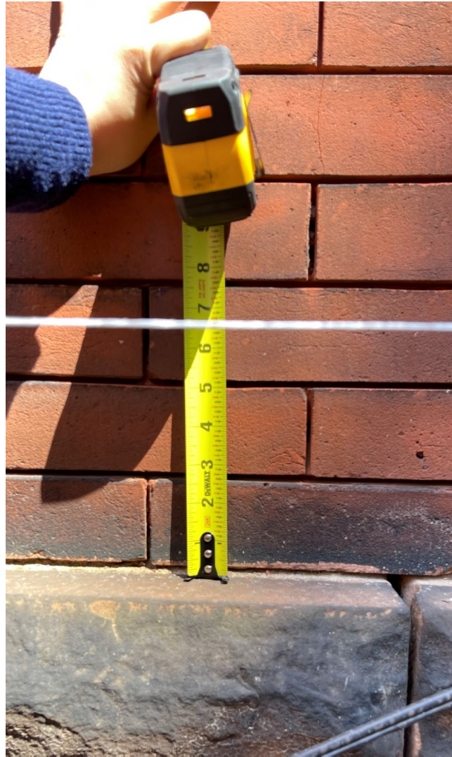
String Level indicates that portion of building adjacent to party wall between (2) buildings has settled close to 3 inches relative to West end of 233 and East end of 231.) Photos taken 2022
