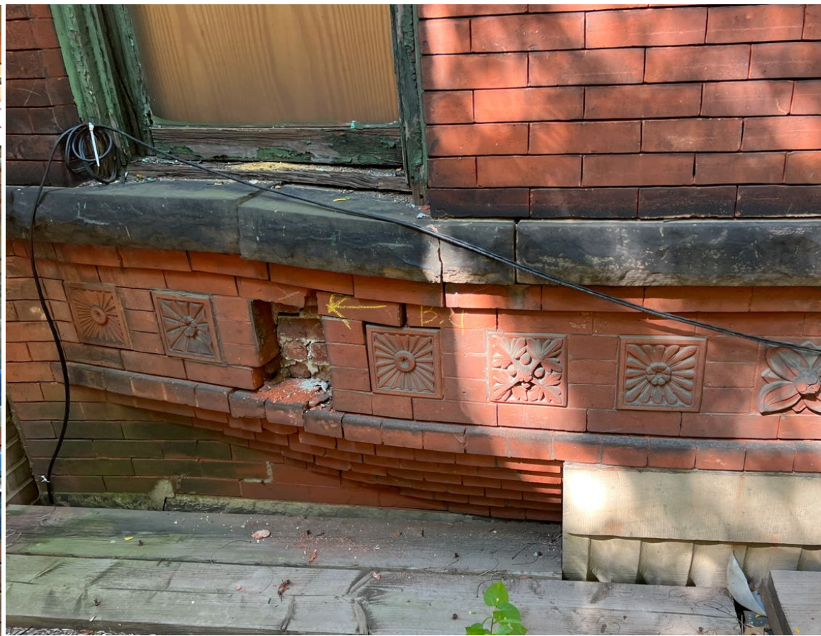
Photo taken 2022 shows increased lateral displacement of the corbelled brick base of the bow window at 233.
