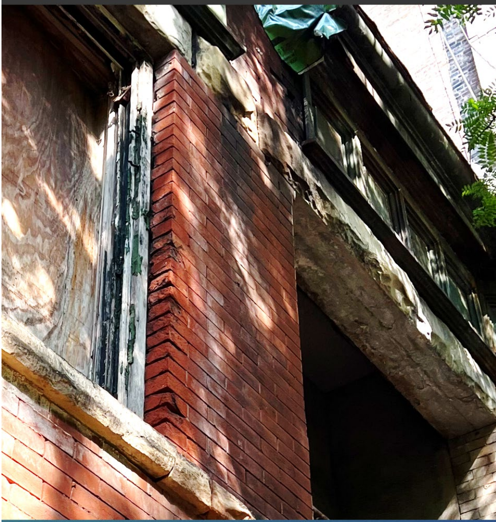
Pier between 233 & 231 exhibits lateral displacement – it is leaning towards the street
