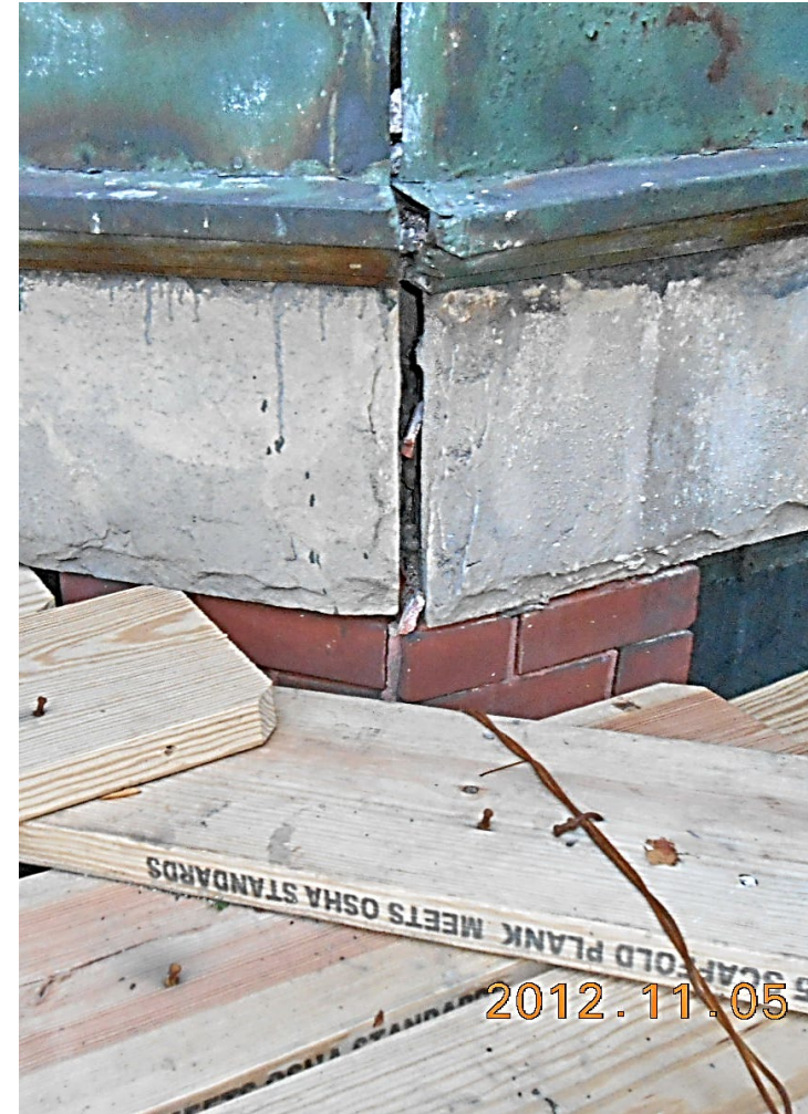
231 West 75 th Street (Differential Façade Settlement visible where bay window segments pulling apart) Photos taken 2012
