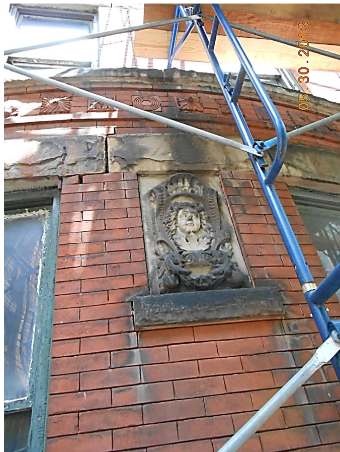
Photo taken 2012 shows separation and lateral displacement at the top the bow window at 233
