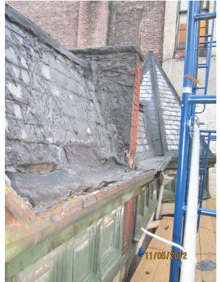
233 West 75 th Street (Severe deterioration of Mansard and Gable Roofs and Integral gutter) Photos taken 2012
