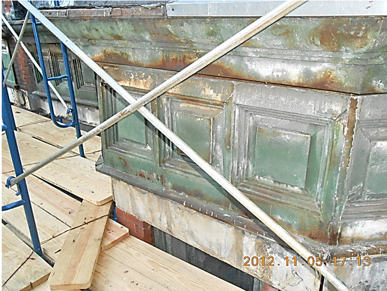
231 West 75 th Street (Differential Façade Settlement visible where bay window segments pulling apart) Photos taken 2012
