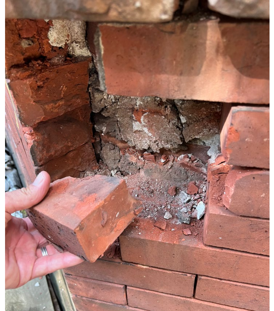
Mortar at facebrick throughout has lost its tensile strength and is easily dislodged making restoration infeasible and reconstruction necessary.
