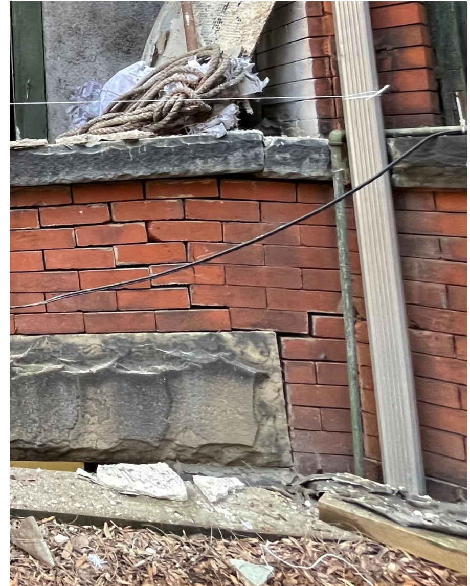
231 West 74 th Street (Lintel above main Entrance severely deformed from façade settlement) 2022
