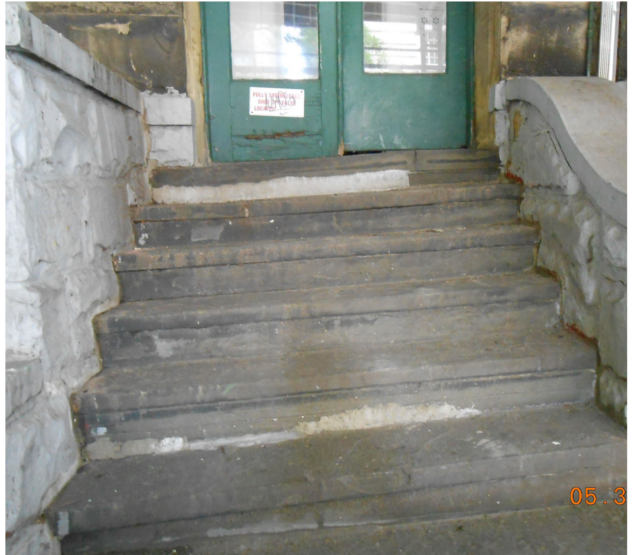
231 W 75 th St (Displacement at Stoop)- Photos taken 2012
