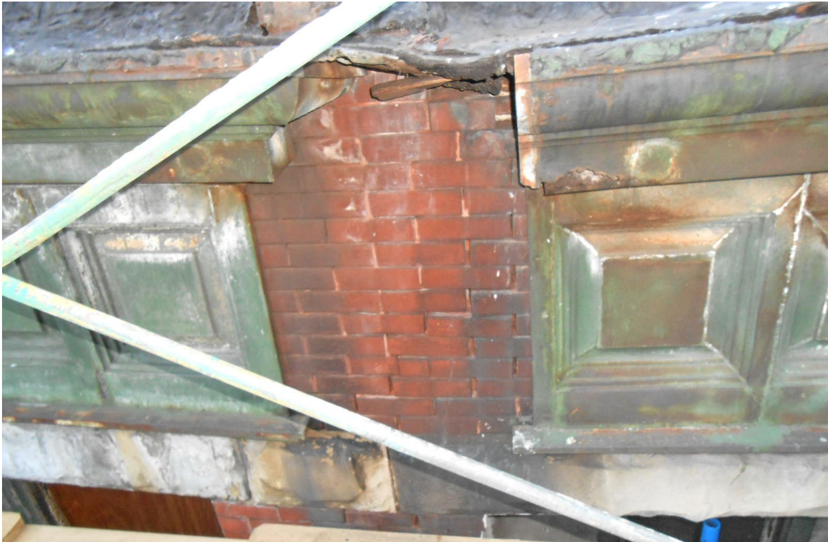
231 / 233 West 75 th Street (Differential Façade Settlement visible at misaligned gutters and mortar joint widths )
