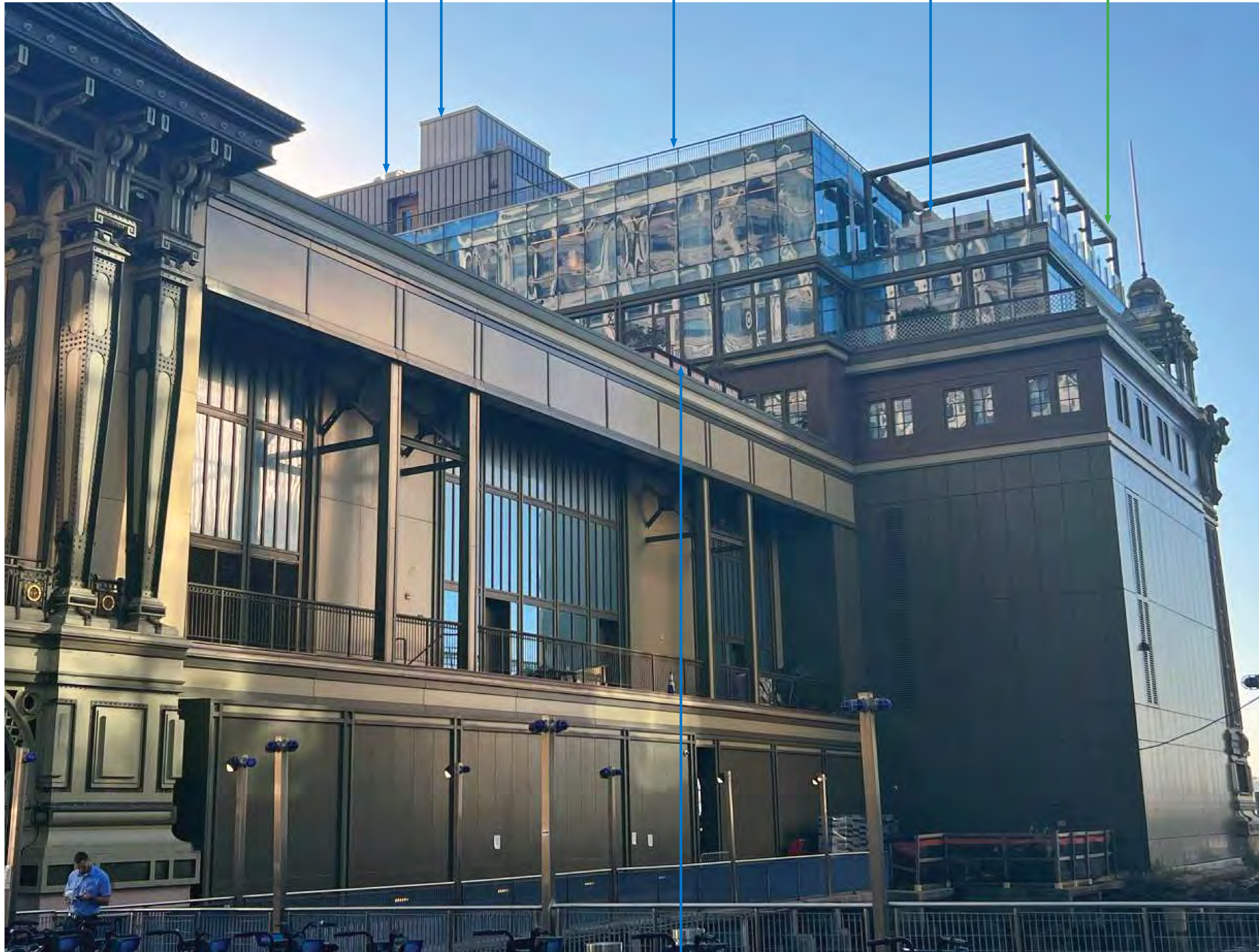
PHOTO | WEST ELEVATION
