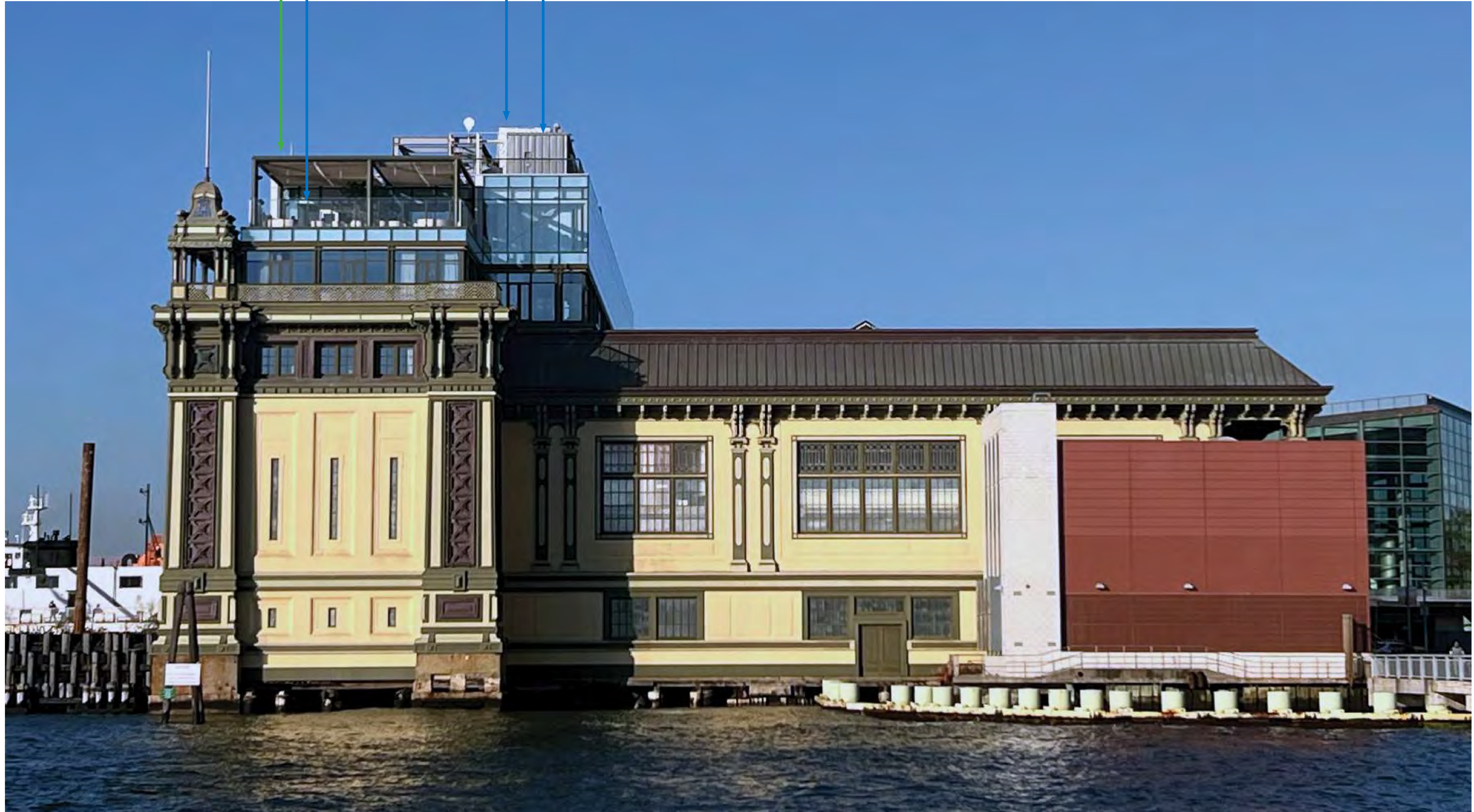
PHOTO | EAST ELEVATION
