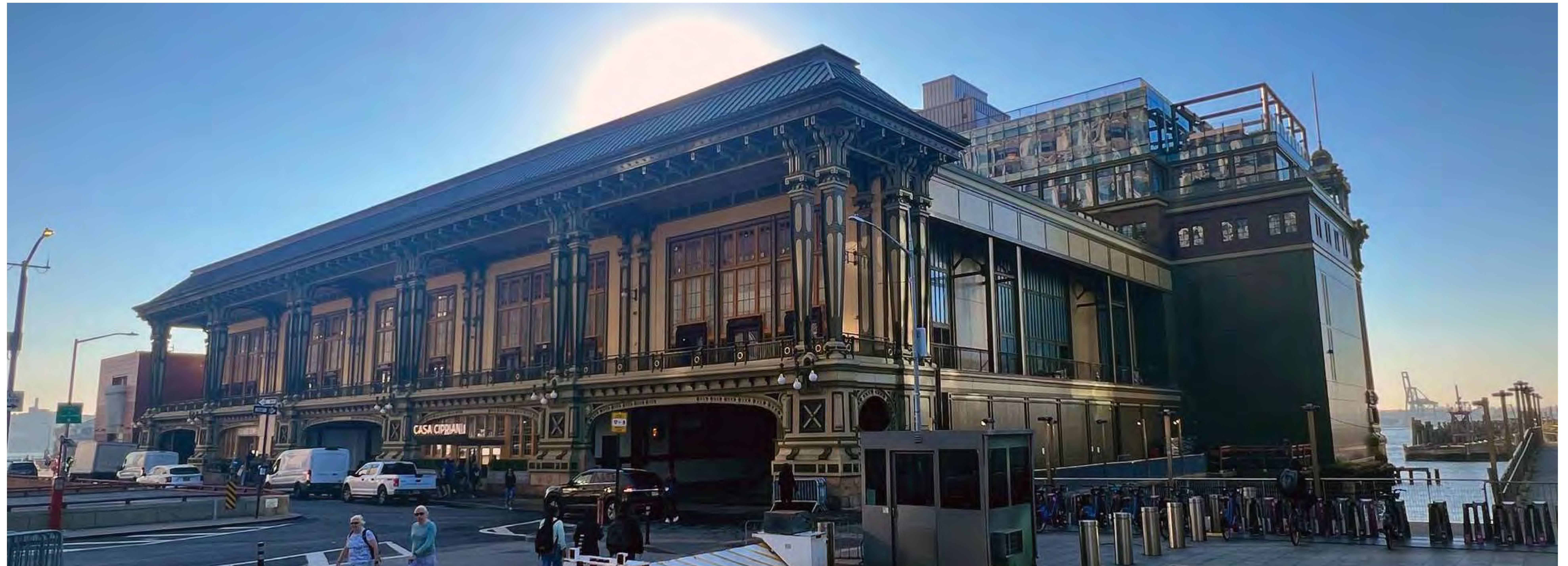
PHOTO | NORTHWEST ELEVATION
