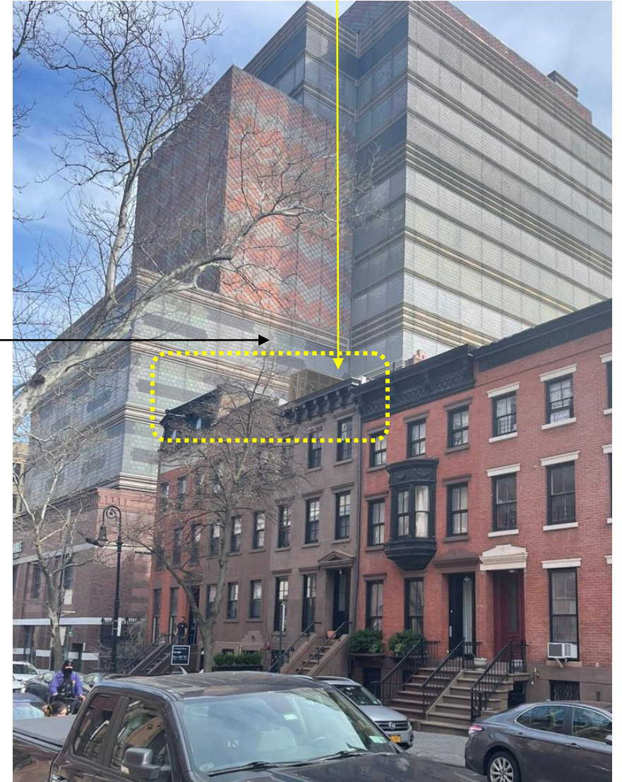
AREA OF NEW PROPOSED ROOF MOCK-UP AREA STREET VIEW
