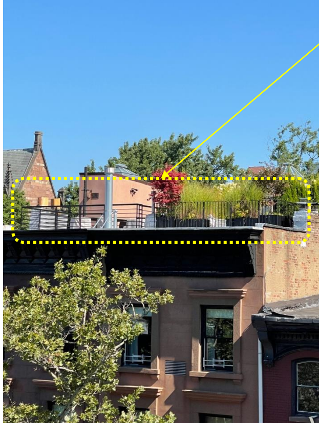
29 SCHERMERHORN & 31 SCHERMERHORN ST ROOF TOP GARDEN AND RAILING
