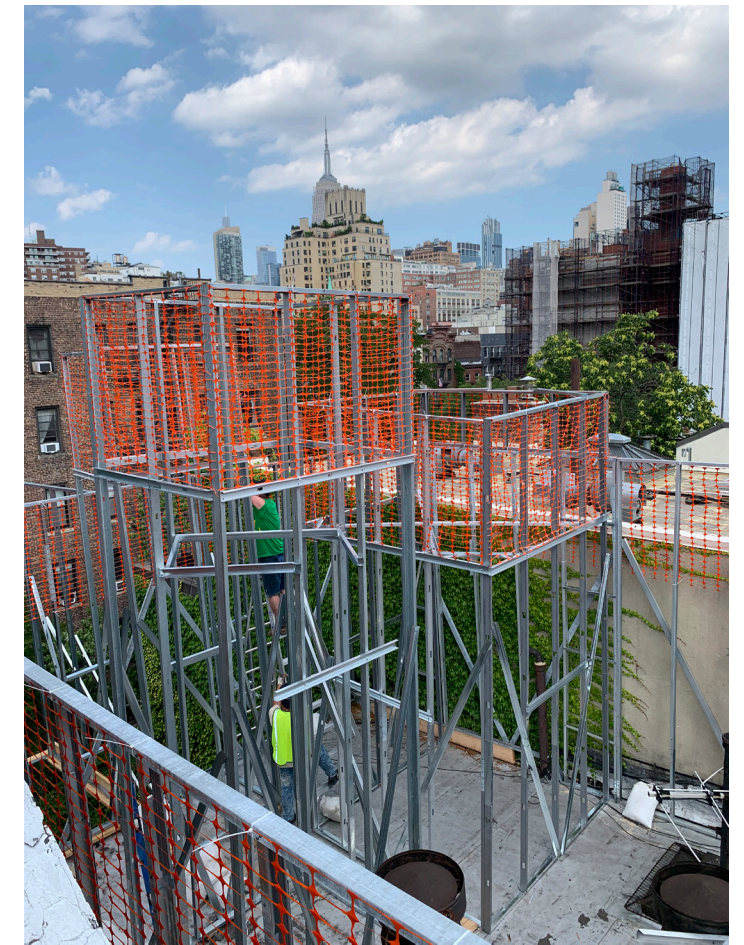
mock up on roof
