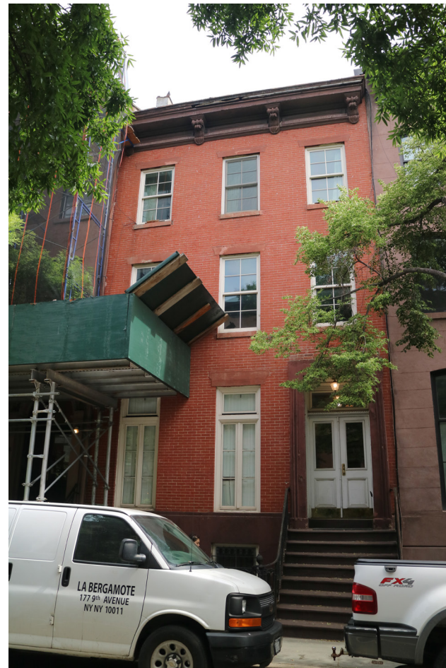
existing (close up)
