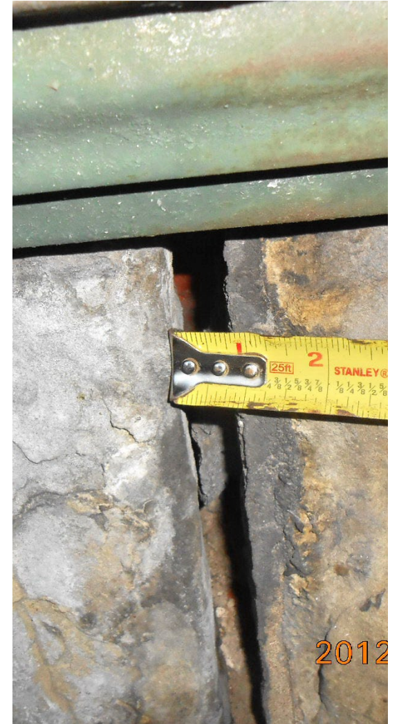
231 / 233 West 75 th Street (Differential Façade Settlement visible at misaligned gutters and mortar joint widths )
