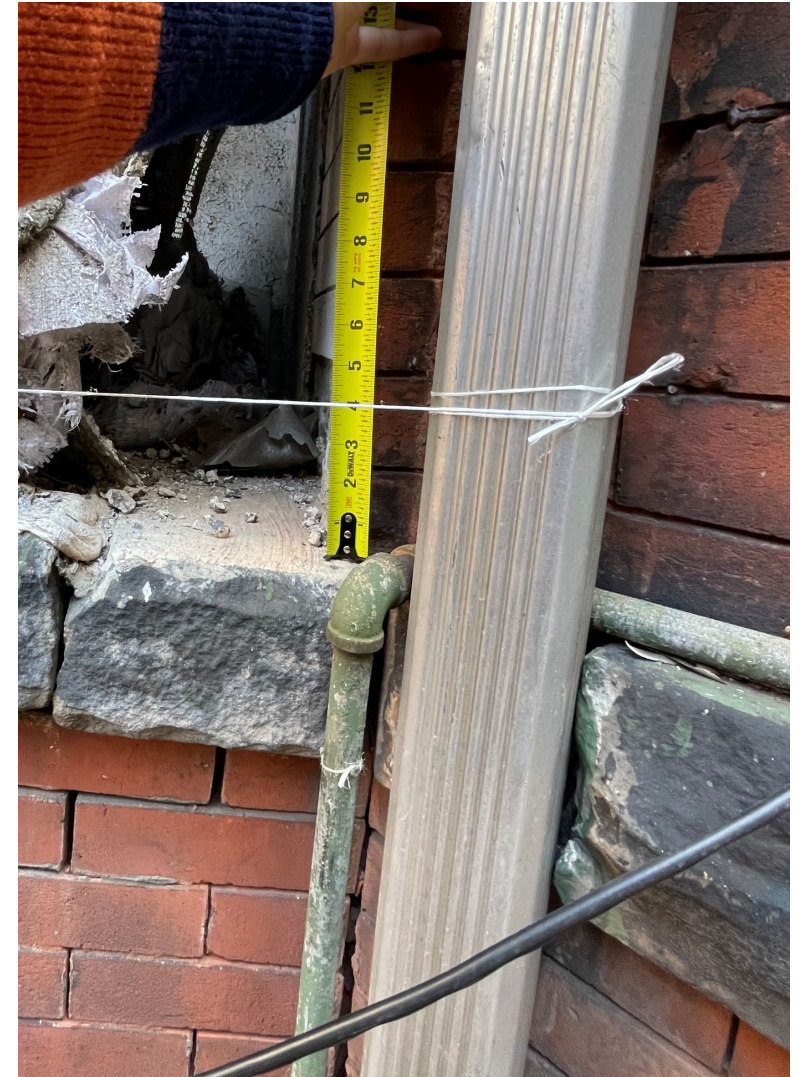
String Level indicates that portion of building adjacent to party wall between (2) buildings has settled close to 3 inches relative to West end of 233 and East end of 231.) Photos taken 2022
