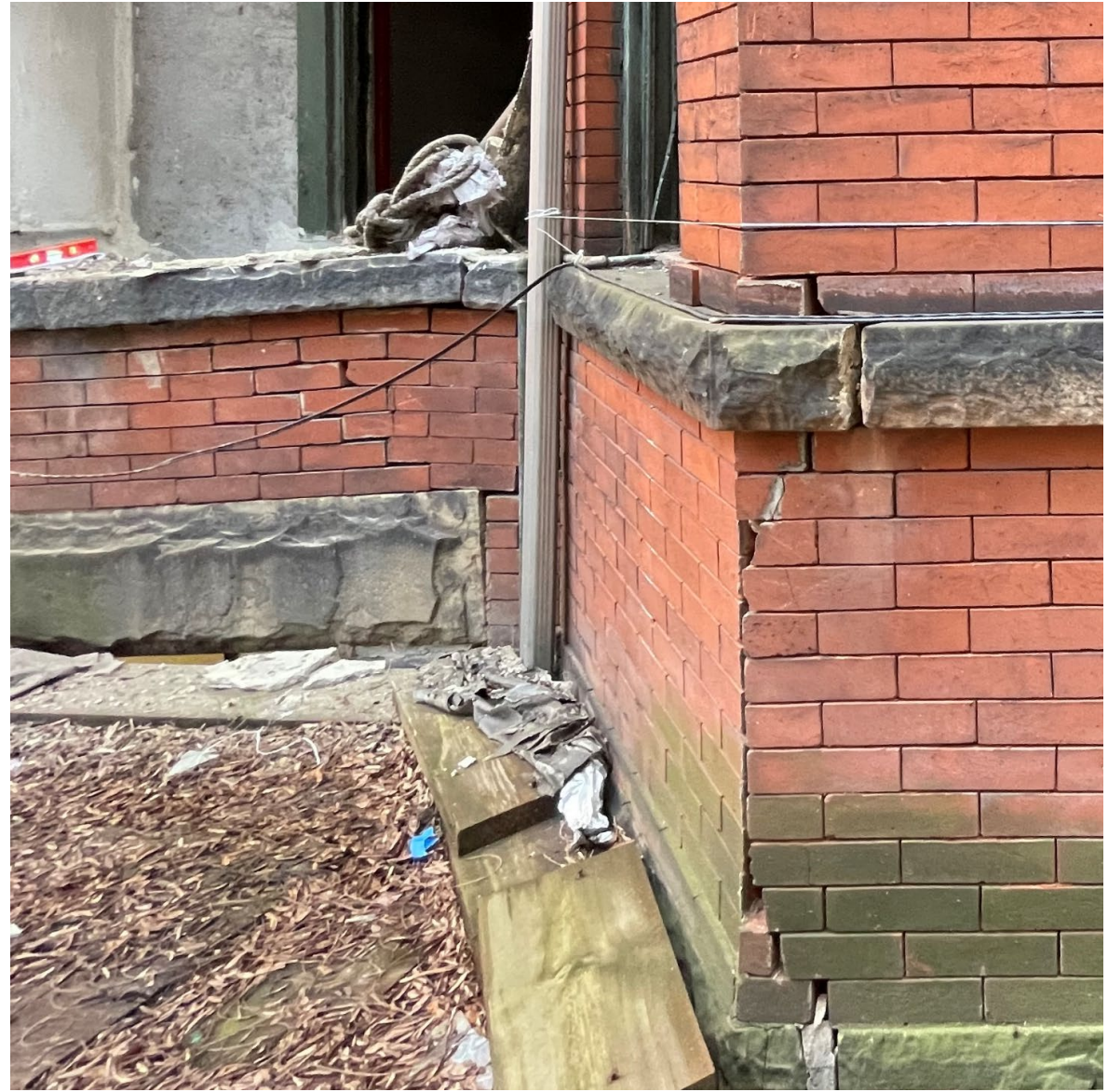
231 West 75 th Street (Bay window segment coming apart at corner and cracked vertically from settlement.)
