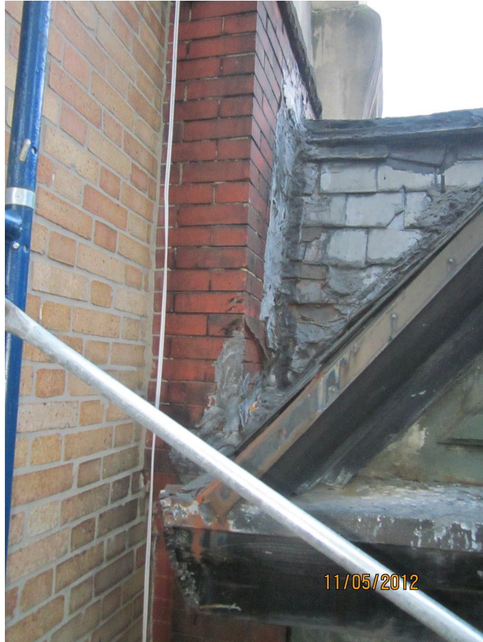
233 West 75 th Street (Severe deterioration of Mansard and Gable Roofs and Integral gutter) Photos taken 2012
