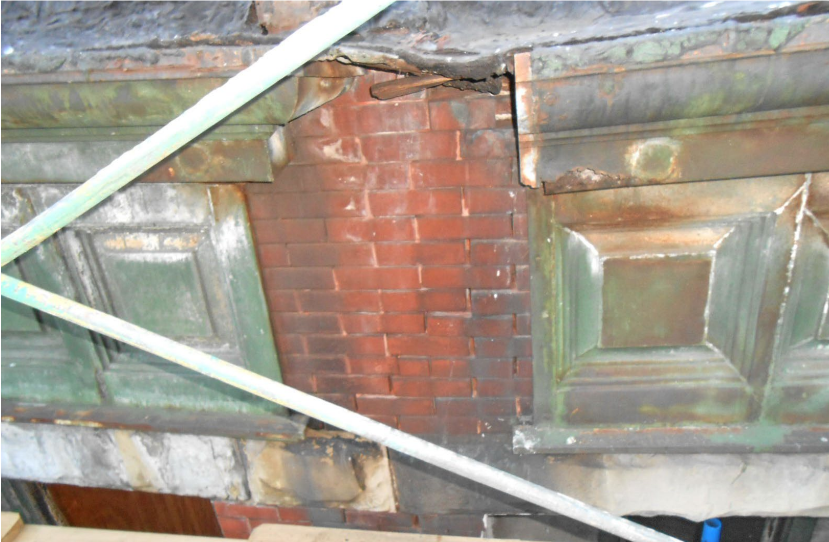
231 / 233 West 75 th Street (Differential Façade Settlement visible at misaligned gutters and mortar joint widths )
