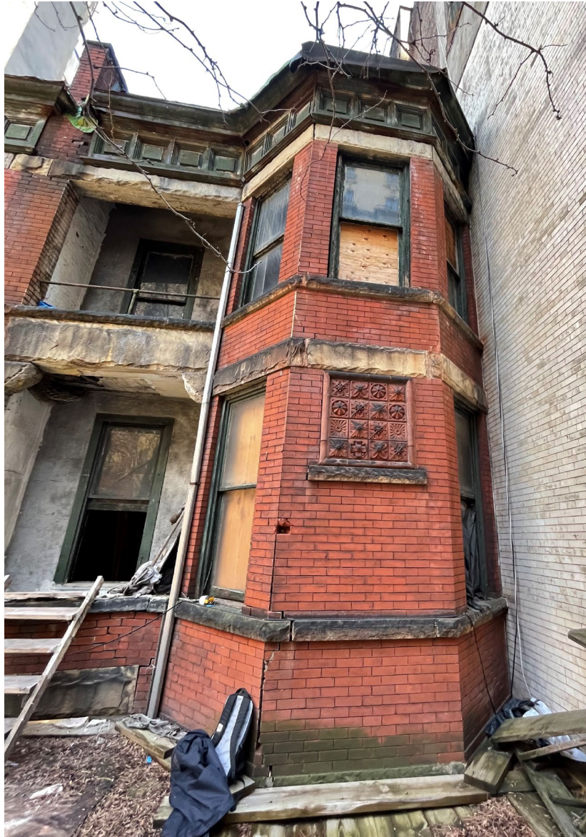
231 West 75 th Street (Bay window segment coming apart at corner and cracked vertically from settlement.)
