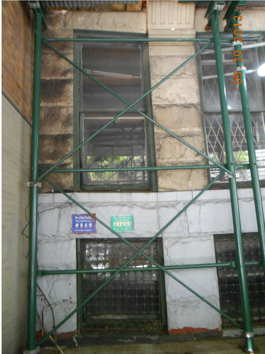
233 W 75 th St (Displacement of Wdw. Ltl.)
